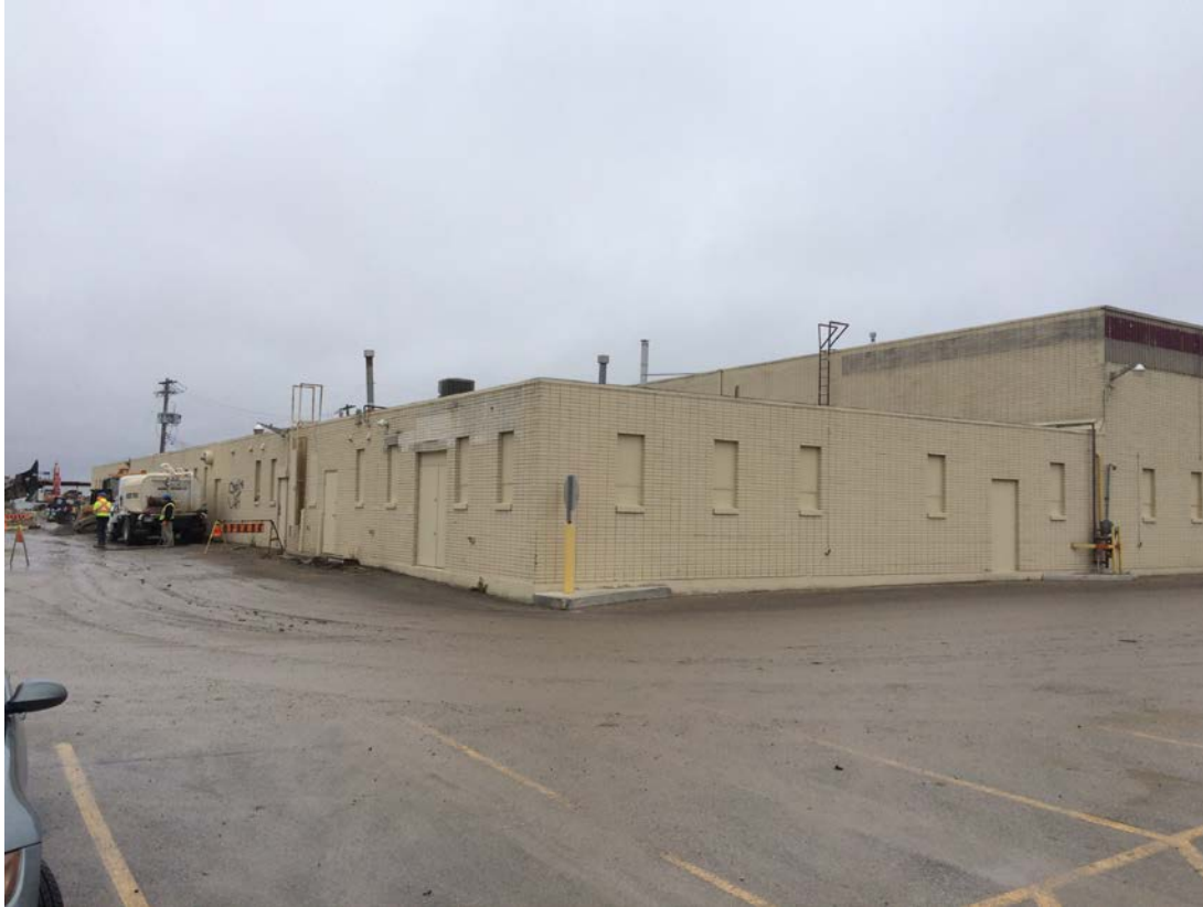
South West Corner of 890-904 St James Ave
