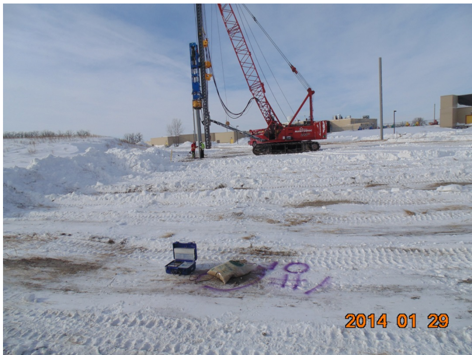
Photo 2 – Pile #1, Showing Monitor M1
