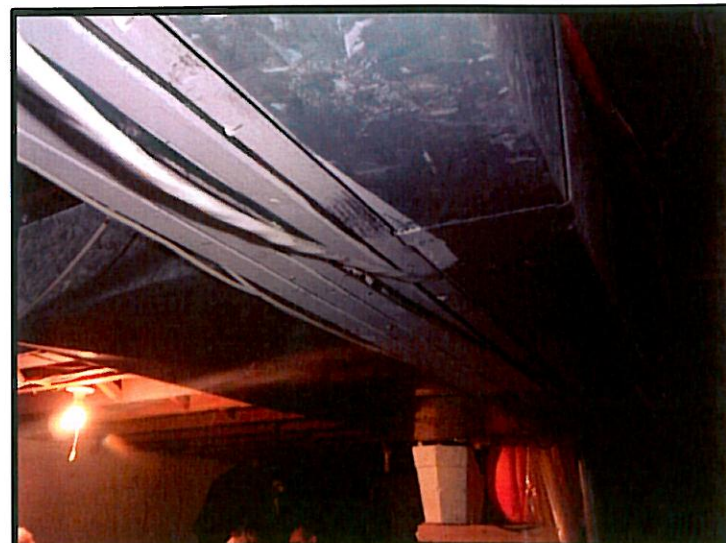
PHOTOGRAPH #16: FACING NORTHWEST, SHOWING MAIN WOOD BEAM OF EXISTING HOUSE.
