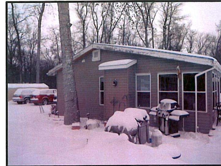
PHOTOGRAPH #12: FACING NORTHWEST, SHOWING SOUTH FACE OF EXISTING HOUSE.
