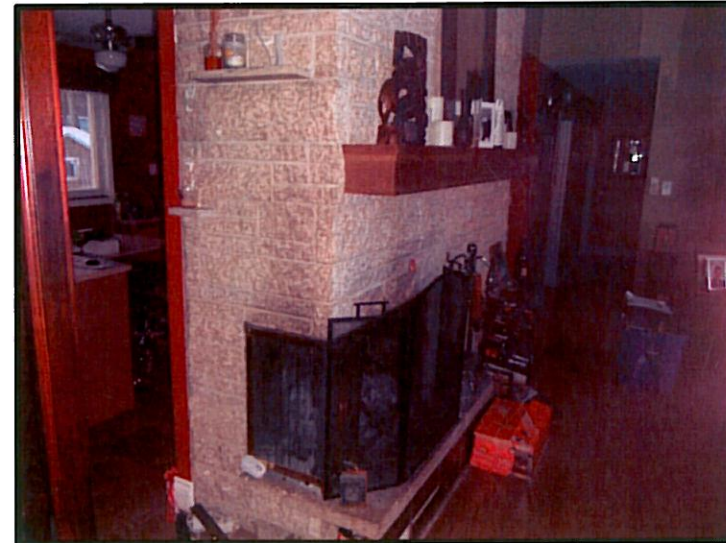
PHOTOGRAPH #14: FACING NORTHWEST, SHOWING EXISTING STONE FIREPLACE.
