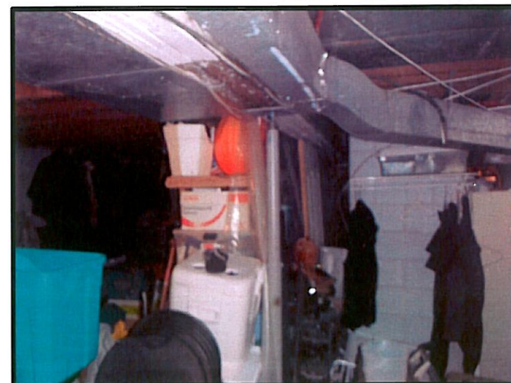
PHOTOGRAPH #17: FACING NORTHWEST, SHOWING EXISTING TELEPOST FROM EXISTING HOUSE FOUNDATION
