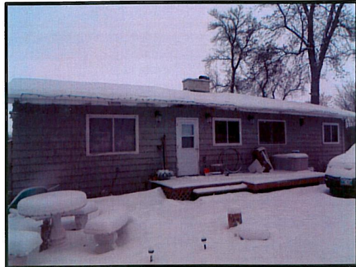
PHOTOGRAPH #13: FACING EAST, SHOWING WEST FACE OF EXISTING HOUSE.
