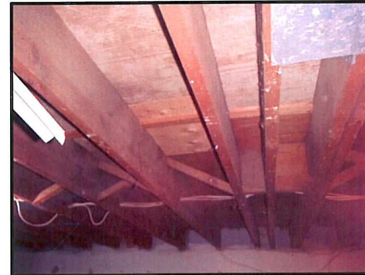
PHOTOGRAPH #15: FACING EAST, SHOWING FLOOR JOIST OF EXISTING HOUSE.
