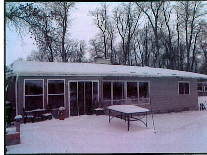
PHOTOGRAPH #11: FACING NORTHEAST, SHOWING EAST FACE OF EXISTING HOUSE.
