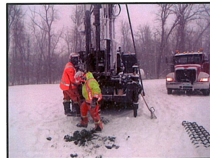
PHOTOGRAPH #18: FACING NORTH, SHOWING THE DRILLING OF TEST HOLE THROUGH THE EXISTING EARTHEN CLAY MOUND.
