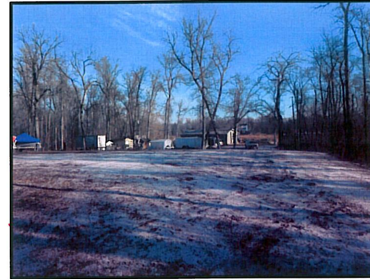
PHOTOGRAPH #3: FACING NORTHEAST, SHOWING CONSTRUCTED FLOOD PROTECTION BERM FROM TOP OF BERM.
