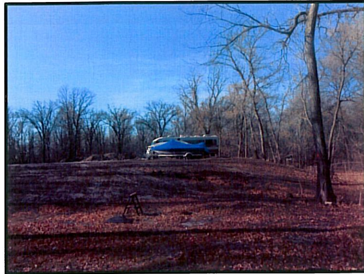
PHOTOGRAPH #1: FACING WEST, SHOWING CONSTRUCTED FLOOD PROTECTION PRE- HOUSE RELOCATION ALONG NORTH PROPERTY BOUNDARY.
