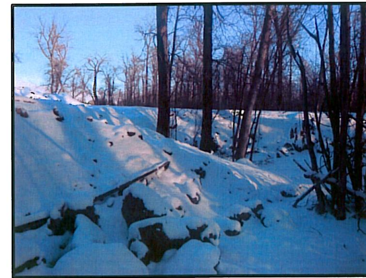
PHOTOGRAPH #9: FACING SOUTHEAST, SHOWING THE LOCATION OF TREE WITHIN THE AREA OF THE SIDE SLOPE OF THE BERM.
