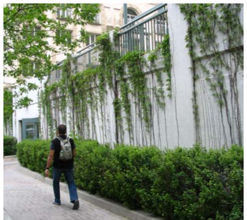
Vines against this downtown parkade deter graffiti and soften the exterior of the walls.
