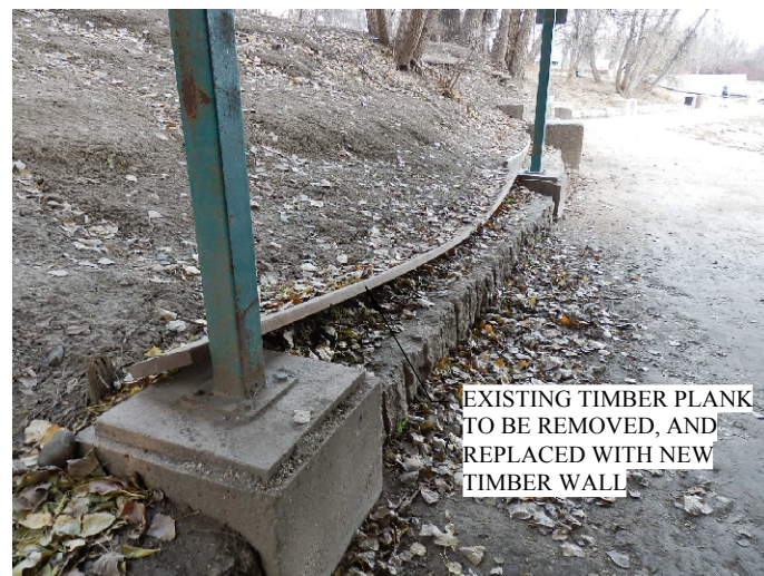
3 EXISTING TIMBER PLANK WALL PHOTO L2 Scale: 1:200
