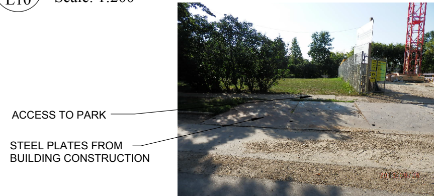
3 EXISTING PHOTO - STREET VIEW L10 Scale: 1:200
