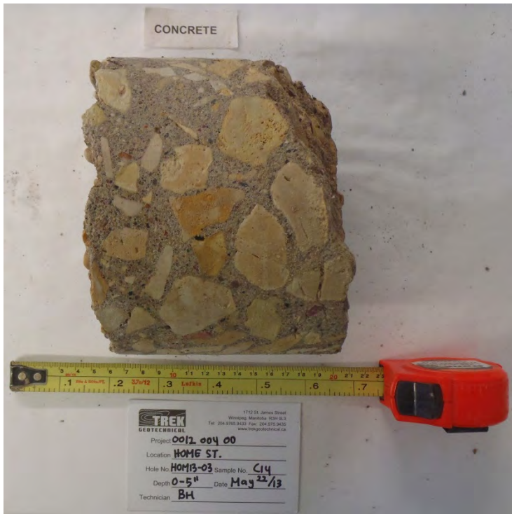
Photo 3: Concrete Core Sample from Test Hole HOM13-03
