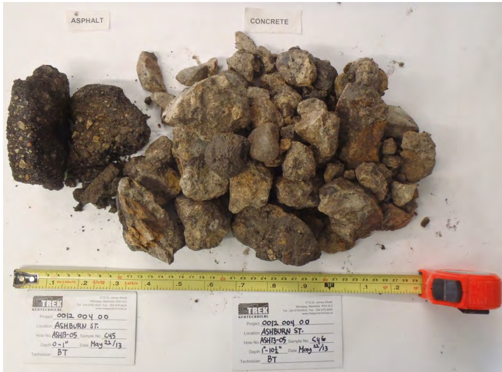
Photo 5: Asphalt and Concrete Core sample from Test Hole ASH13-05
