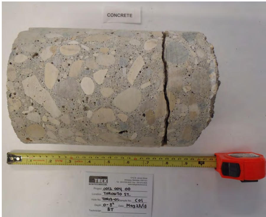
Photo 1: Concrete Core Sample from Test Hole TOR13-01
