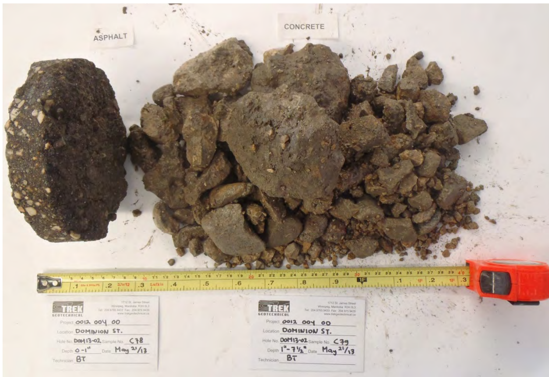
Photo 2: Asphalt and Concrete Core Sample from Test Hole DOM13-02
