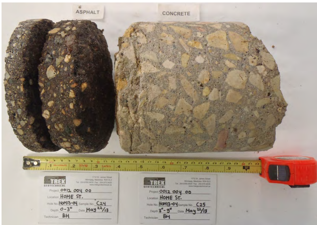
Photo 4: Asphalt and Concrete Core Sample from Test Hole HOM13-04
