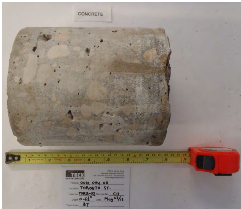
Photo 2: Concrete Core Sample from Test Hole TOR13-02
