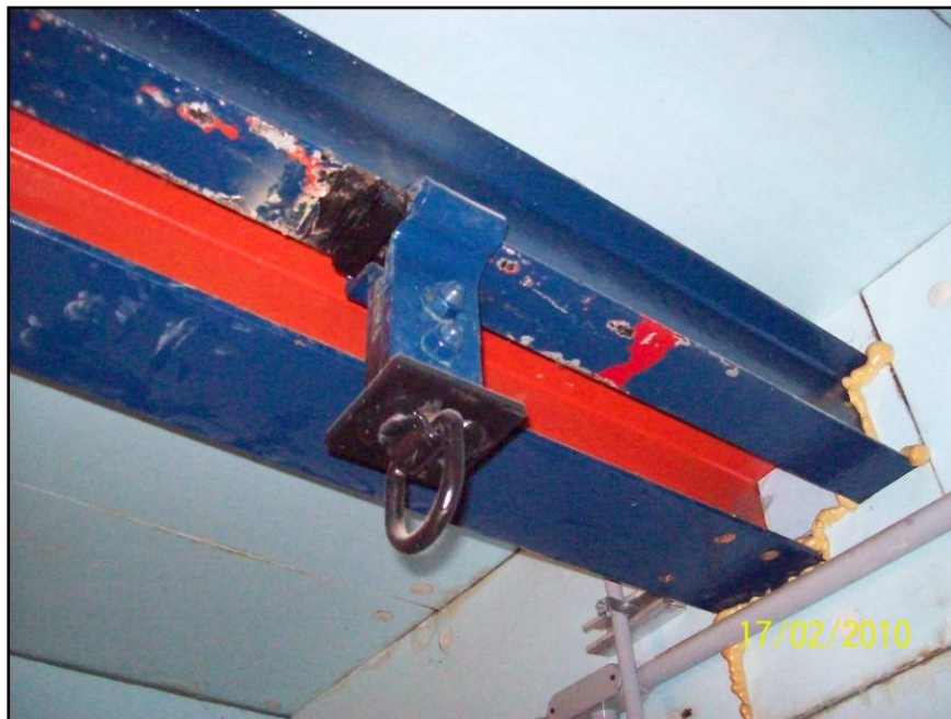
Side by side lifting beams on the main floor
