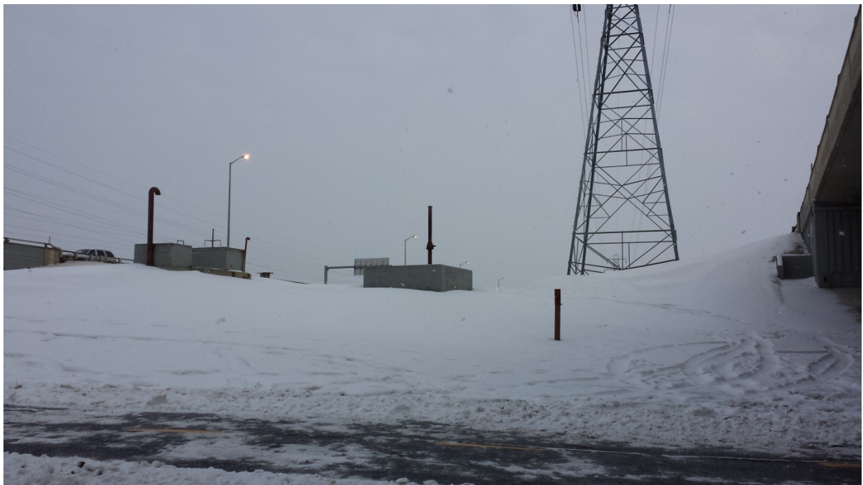
Figure 2 – Siphon Discharge Chamber (left) and Aqueduct Blow Off Chamber (right)
