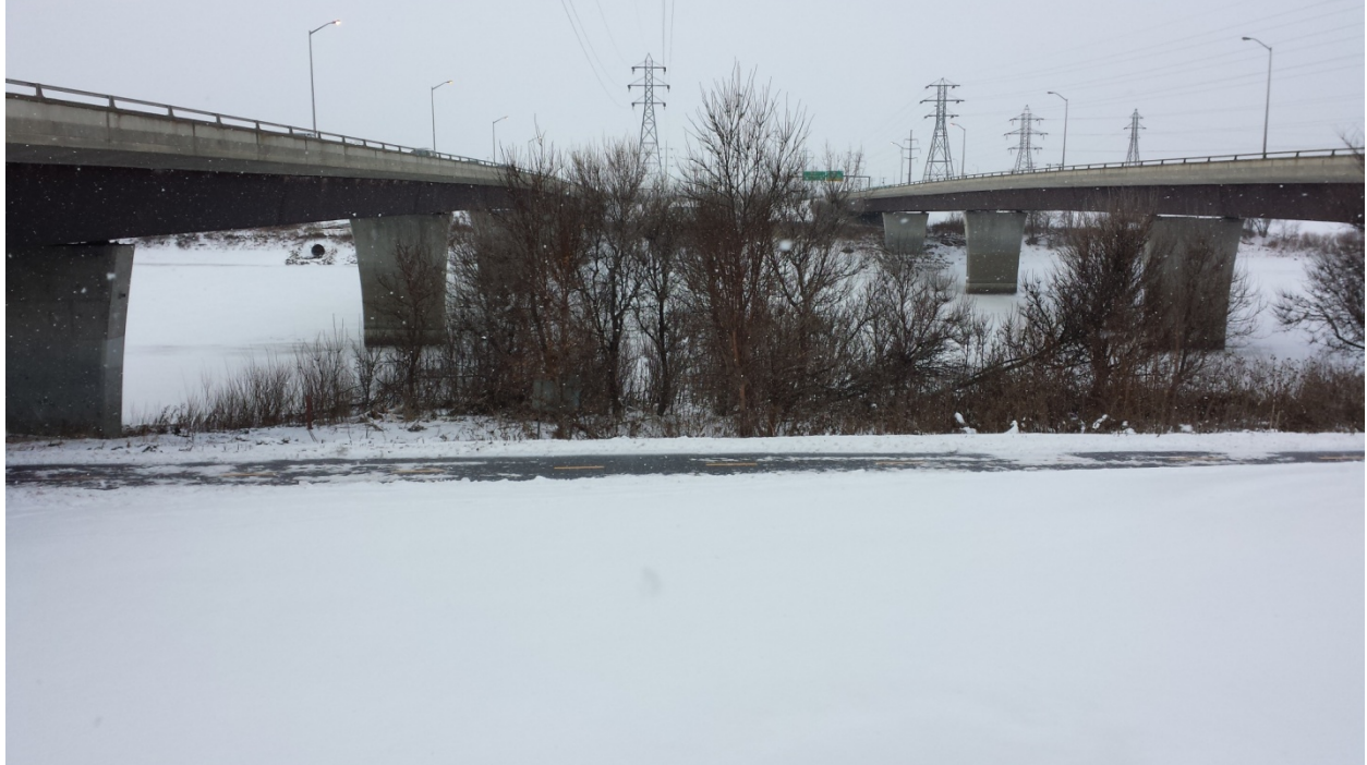
Figure 1 – Repair Area (looking west)
