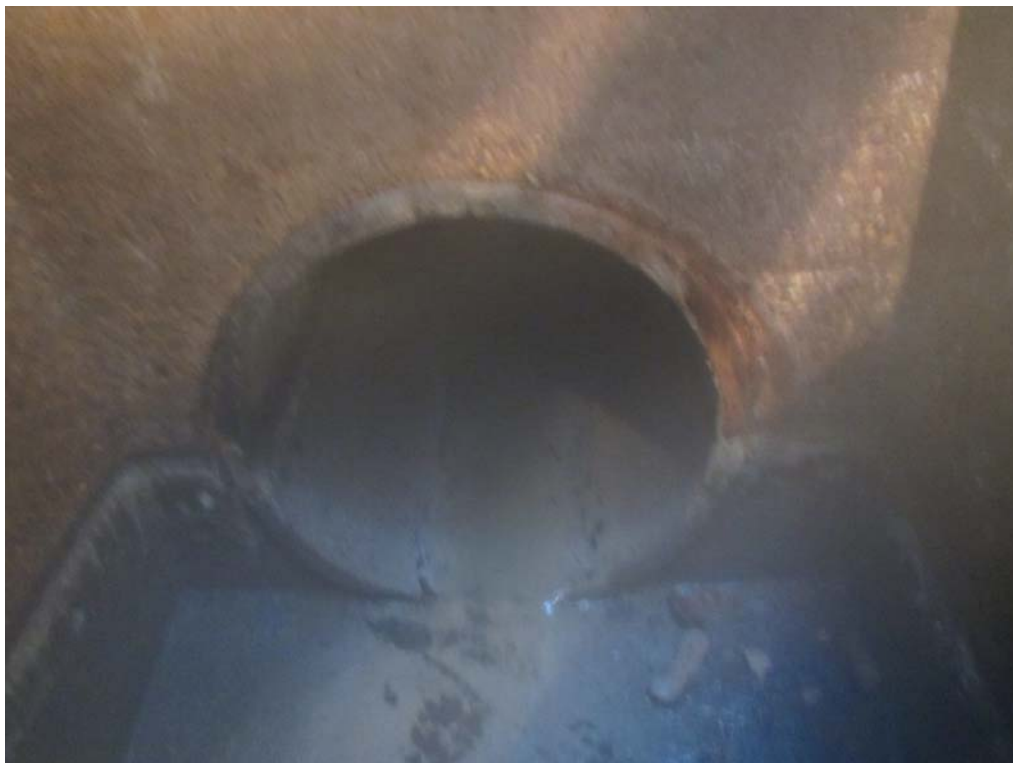
Figure 6 – Siphon Discharge Chamber (800 mm Siphon)
