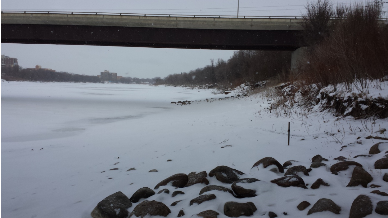
Figure 4 – Riprap Installation Area (looking north)
