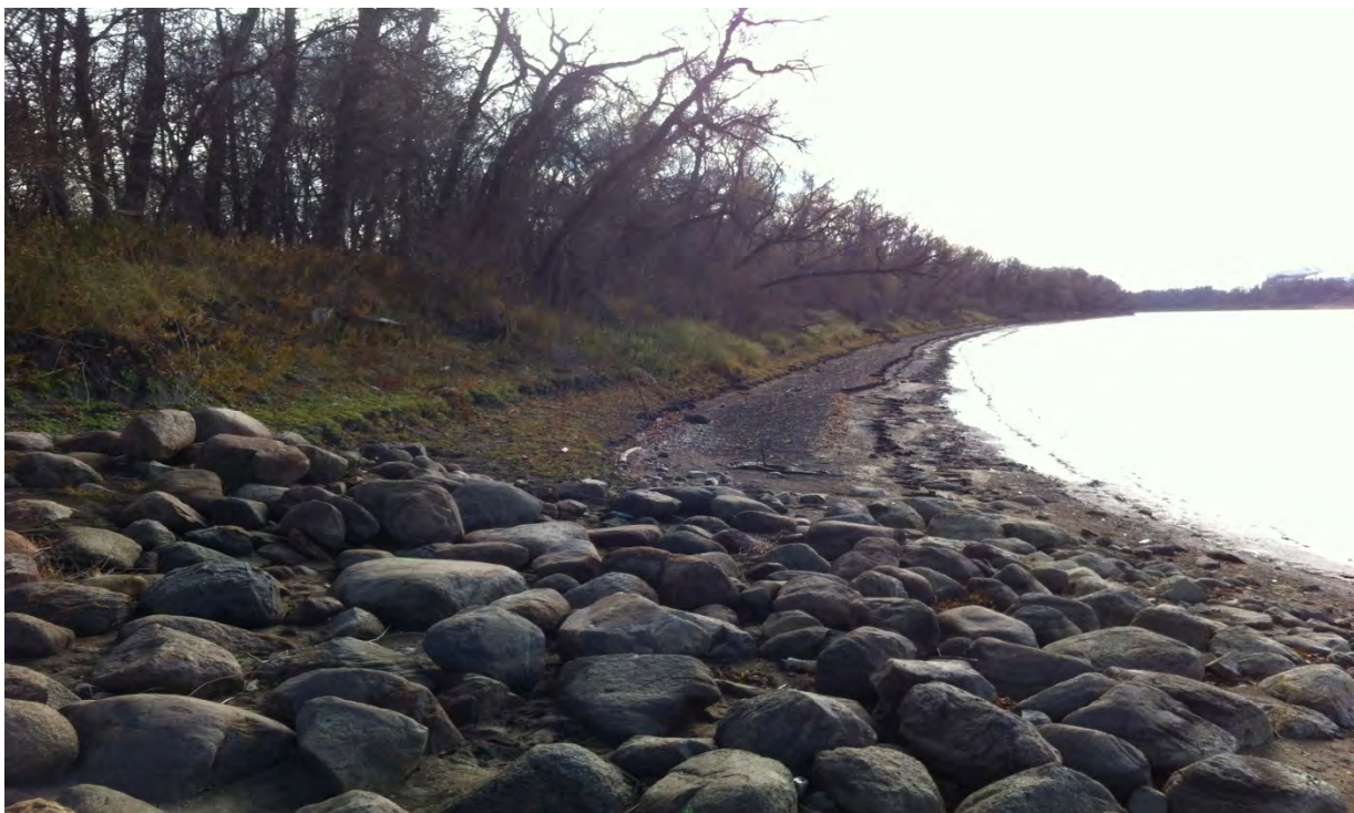
Photo 4: Rip-rap blanket placed below eastbound Bishop Grandin Bridge, facing south.
