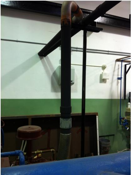
Photo A-7: Fire Pump #2 Exhaust and Wall Penetration
