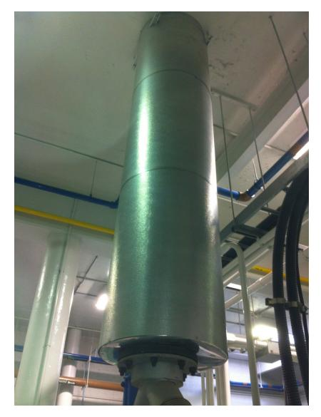
Photo A-1: Emergency Generator Exhaust Vertical Section
