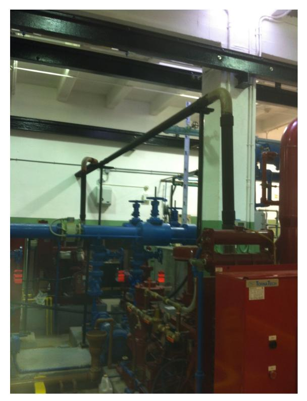
Photo A-8: Fire Pump #1 Exhaust Pipe Run
