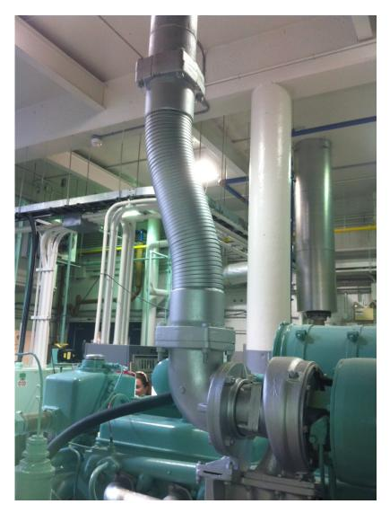
Photo A-4: Low Lift Pump Exhaust Flexible Section
