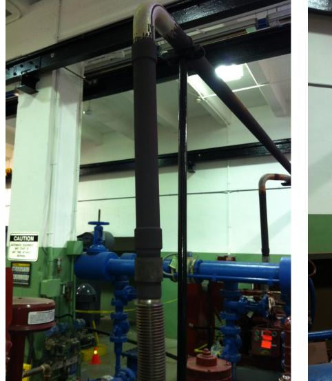
Photo A-6: Fire Pump #1 Vertical Exhaust and Bend
