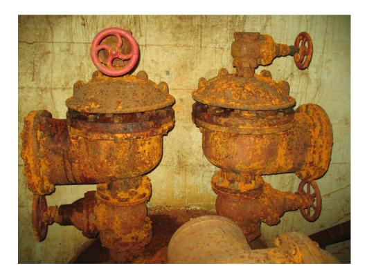
Figure 11 - DAV1 - Existing Air Release Valve Assemblies
