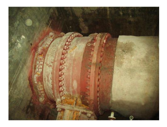
Figure 7 – VC4 - Existing 1500 mm Motorized Valve and Vic Coupling
