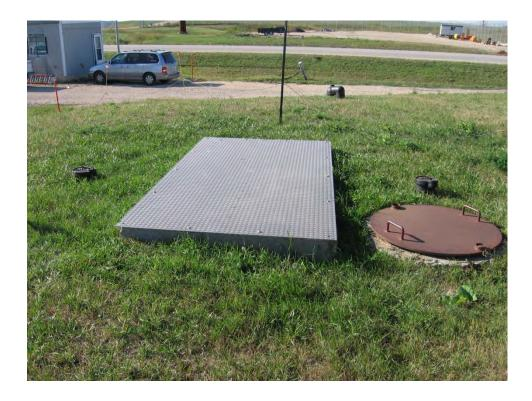
Figure 9 - DAV1 - Existing Cover and Access Manhole
