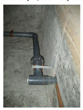
Figure 18 - Chlorine Contact Chamber - Existing PVC Injector Piping at Wall
