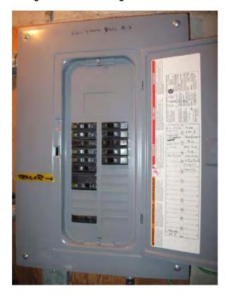
Figure 4 - VC4 - Existing Electrical Panel
