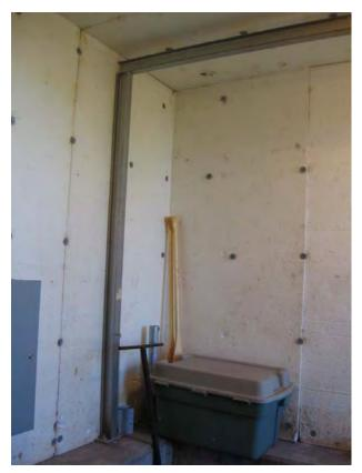
Figure 16 - Cell 1 Dewatering Pump Station - Lifting Frame and Insulation
