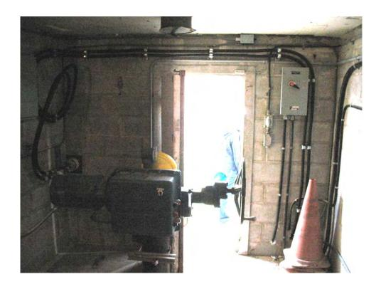
Figure 5 - VC4 - Existing Valve Actuator Motor
