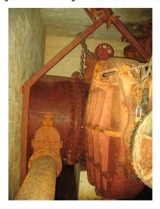
Figure 12 - DAV1 - Existing 300 mm Gate Valve and Drain Piping
