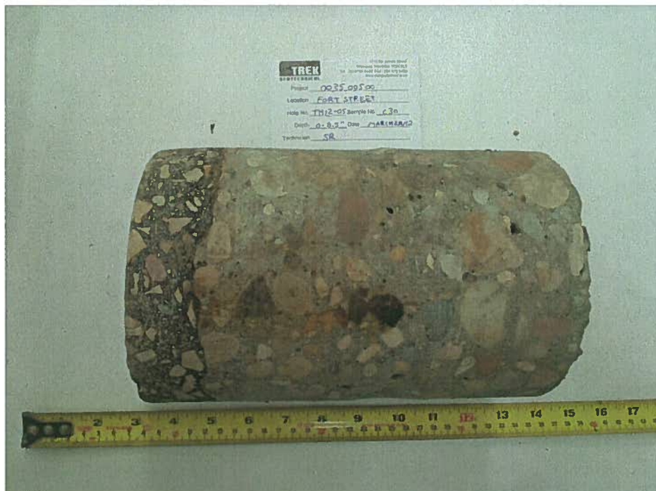
Photo 7: Asphalt and concrete core sample from Test Hole TH12-05
