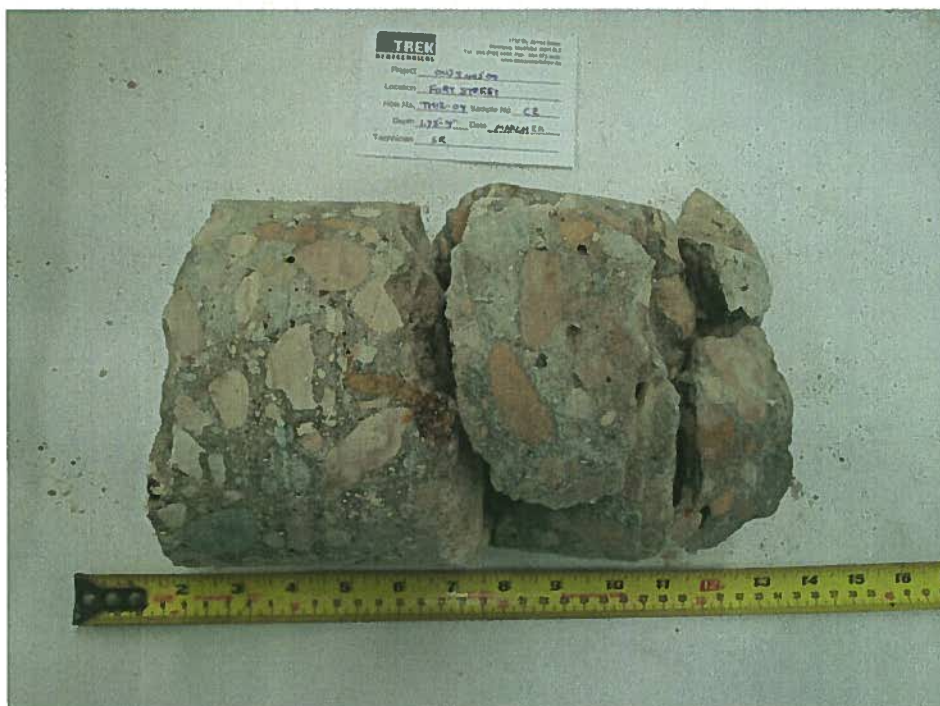
Photo 6: Concrete core sample from Test Hole TH12-04
