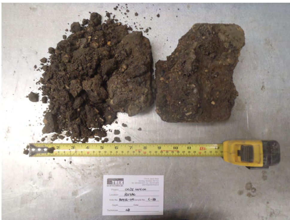
Photo 4: Asphalt core sample from Test Hole ROY12-04
