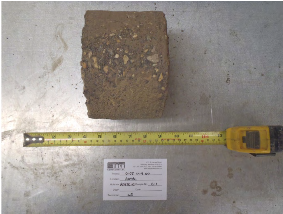
Photo 1: Asphalt core sample from Test Hole ROY12-01
