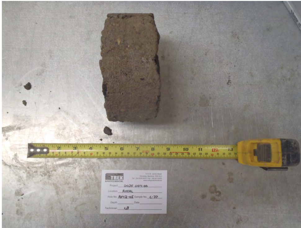
Photo 5: Asphalt core sample from Test Hole ROY12-05
