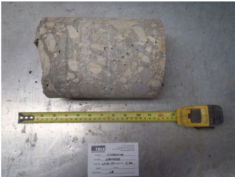
Photo 9: Concrete core sample from Test Hole LY12-03
