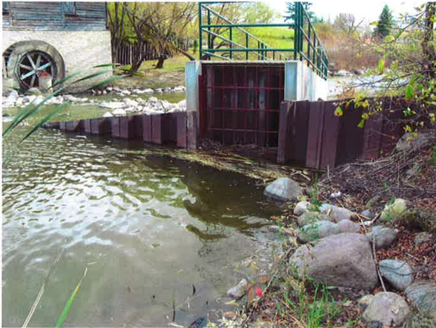
Photo # 9: Sturgeon Creek, upstream entrance to fish ladder at Old Grant's Mill, October 14, 2010.
