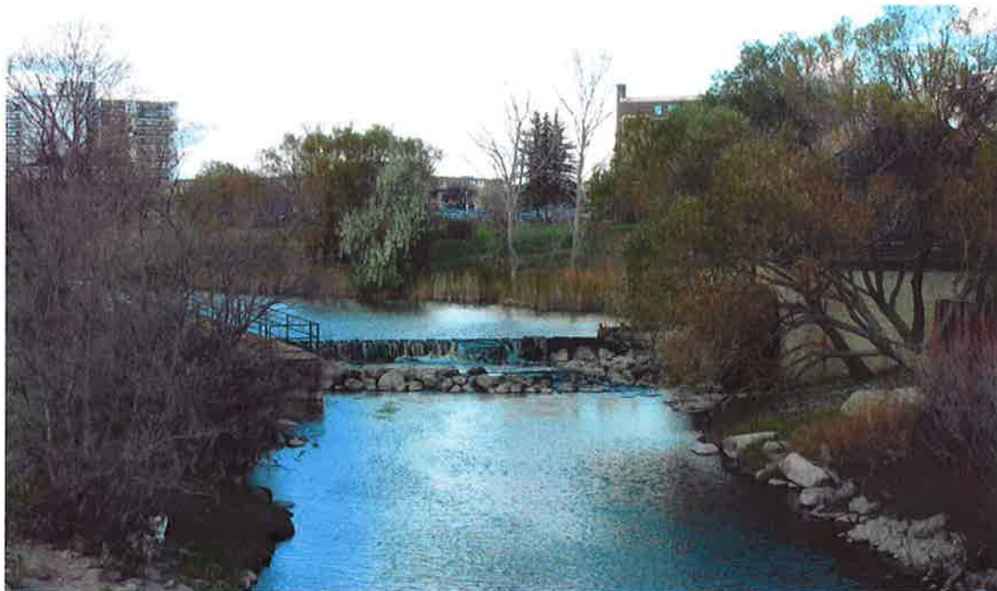
Photo #8: Sturgeon Creek, Old Grant's Mill, looking upstream from Portage Bridge, October 14, 2010.
