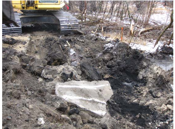
Looking south at excavated area. 2008-03-23_Field Excavation_P010
