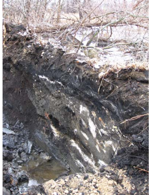
Looking south at excavated area. Note foundation wall beneath existing retaining wall approximately 2.5m deep. 2008-03-23_Field Excavation_P014
