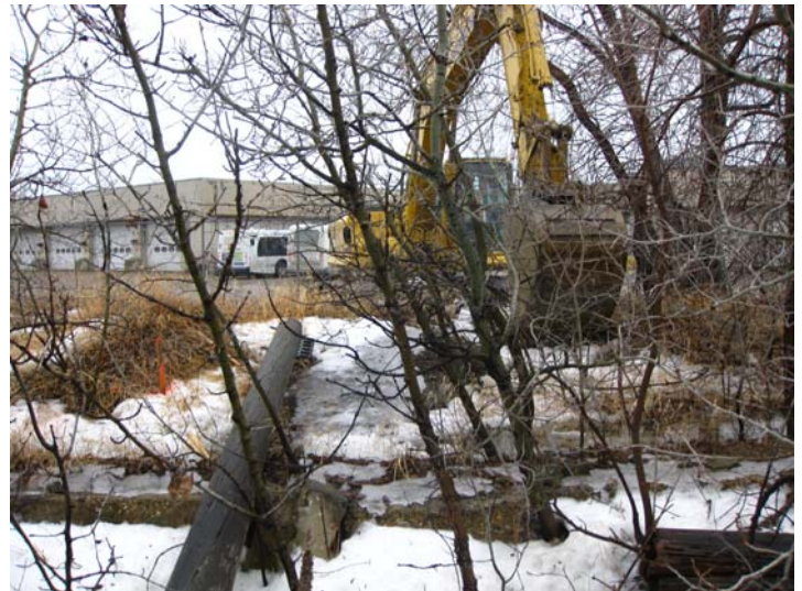
Looking east at area just prior to excavation. 2008-03-23_Field Excavation_P004
