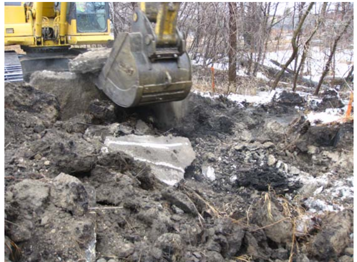
Looking south at excavated area. Note concrete slabs. 2008-03-23_Field Excavation_P008
