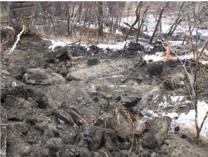
Looking south at excavated area. 2008-03-23_Field Excavation_P007
