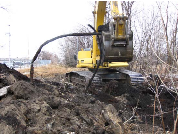
Looking south at excavated area. Note abandoned steel pipe. 2008-03-23_Field Excavation_P011
