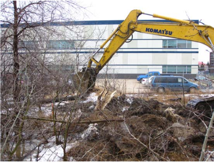
Looking north at excavated area. 2008-03-23_Field Excavation_P005
