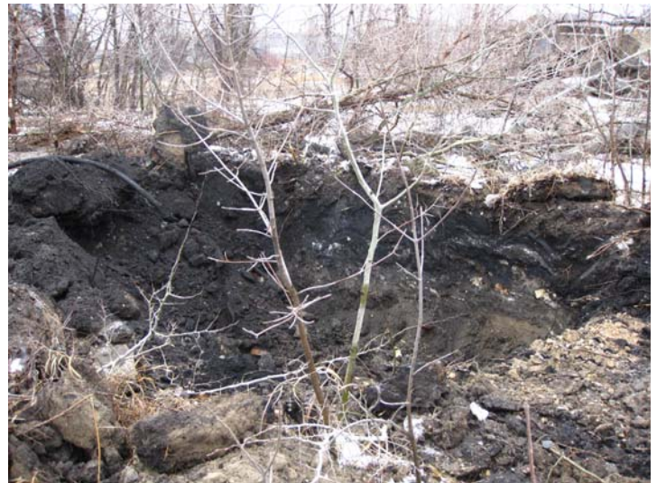
Looking west at excavated area adjacent existing retaining wall. 2008-03-23_Field Excavation_P012
