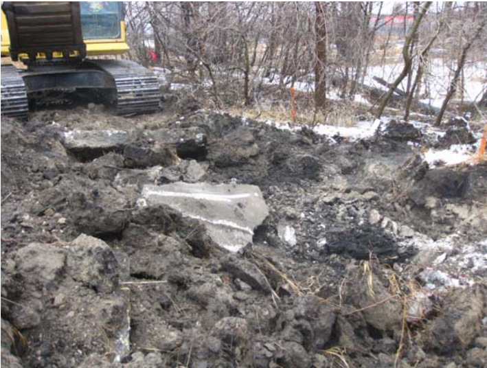
Looking south at excavated area. 2008-03-23_Field Excavation_P009
