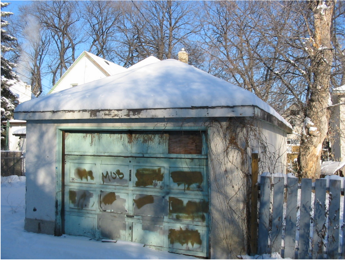
394 Alfred Ave – Garage
