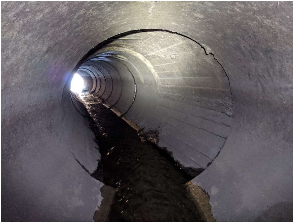
Photo Date: December 4, 2020 / at 1m upstream from bend location, looking downstream
