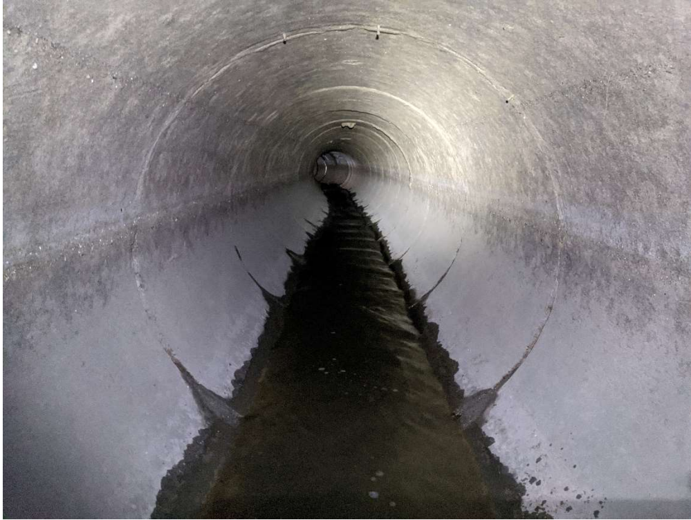
Photo Date: December 4, 2020 / At chamber wall looking downstream
