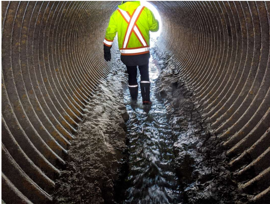
Photo Date: December 4, 2020 / at CMP transition looking downstream along invert
