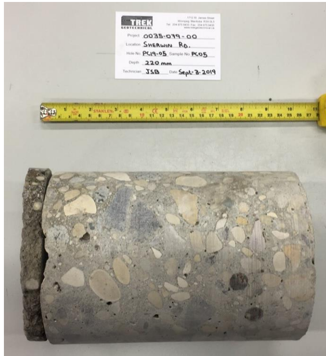
Photo 5: Pavement Core Sample at Test Hole TH19-05
