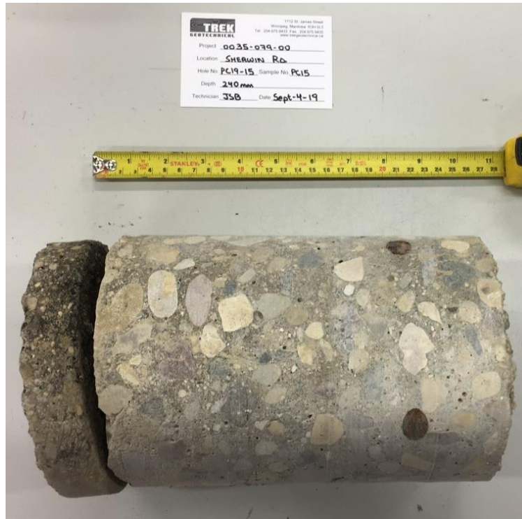
Photo 15: Pavement Core Sample at Test Hole TH19-15
