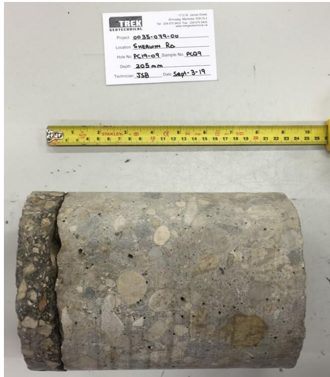
Photo 9: Pavement Core Sample at Test Hole TH19-09
