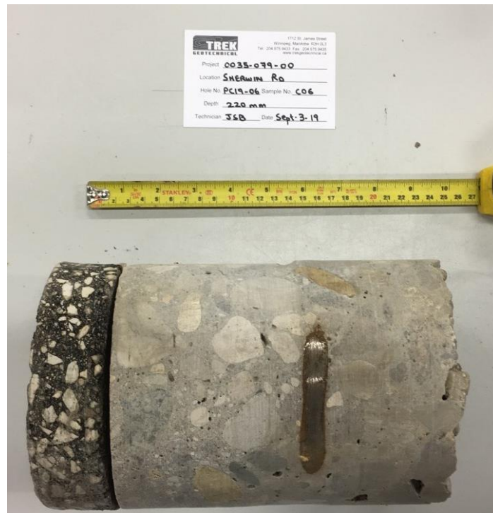
Photo 6: Pavement Core Sample at Test Hole TH19-06
