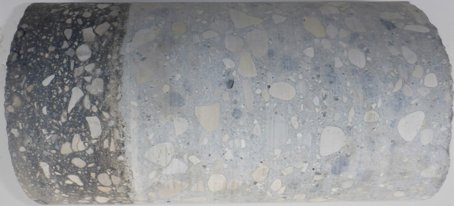
2019 - 2023 Downtown Streets Renewal Fort Street TH19-38
