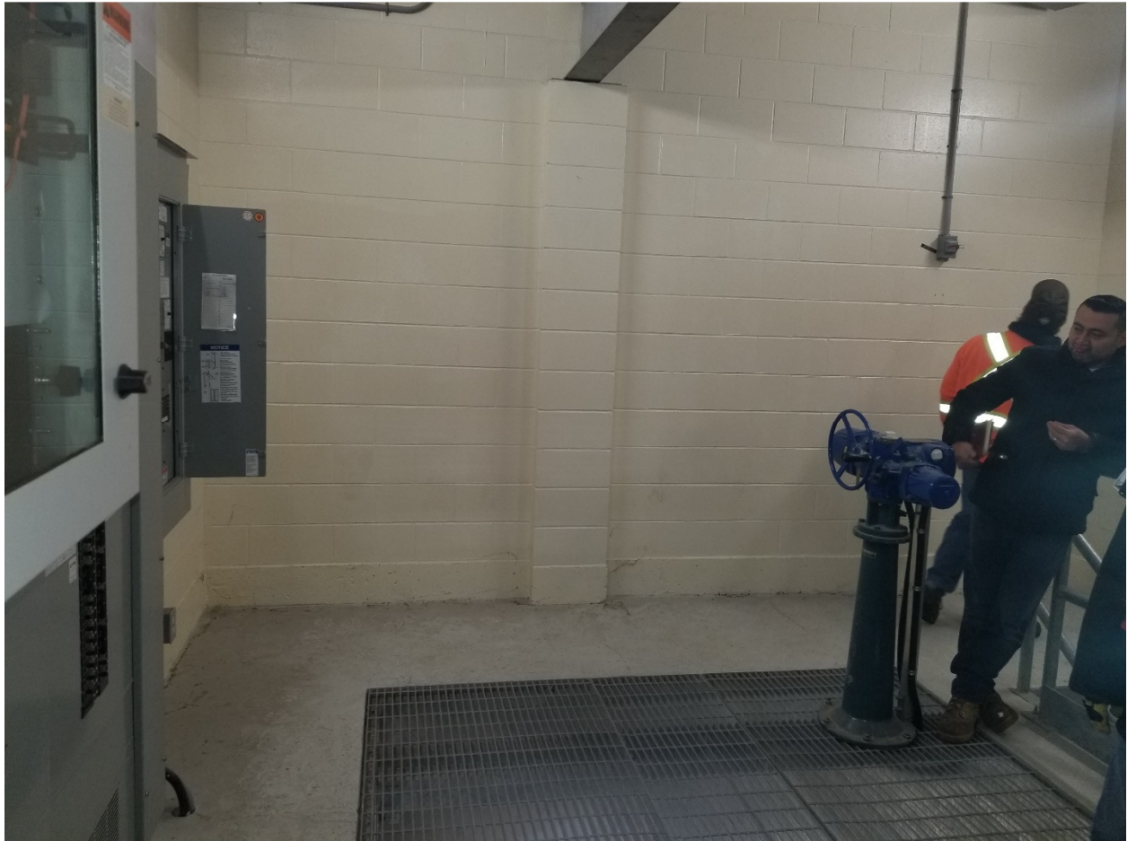
PHOTOGRAPH 30: McPhillips Regional Pumping Station –Branch 1 Aqueduct Valve Chamber – facing west.
