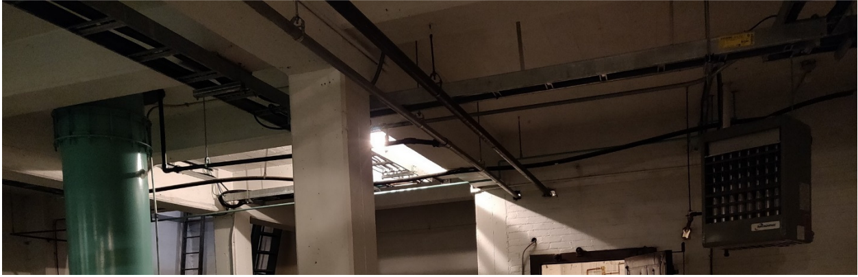
PHOTOGRAPH 41: Tache Booster Pumping Station – Lower Level – facing east showing ceiling.
