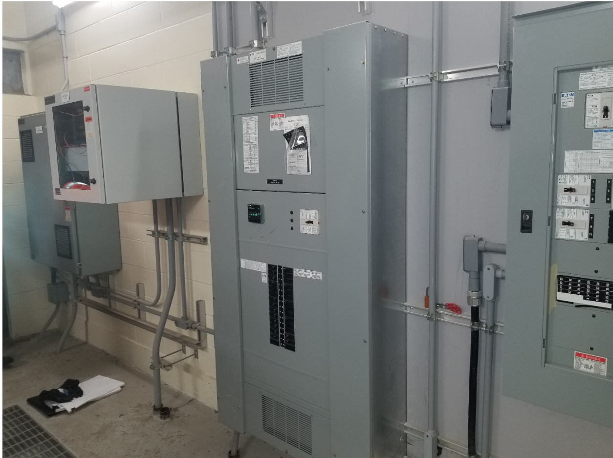
PHOTOGRAPH 29: McPhillips Regional Pumping Station – Branch 1 Aqueduct Valve Chamber – facing south east.
