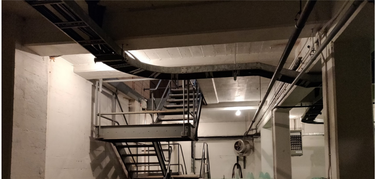
PHOTOGRAPH 40: Tache Booster Pumping Station – Lower Level – facing south west showing ceiling.
