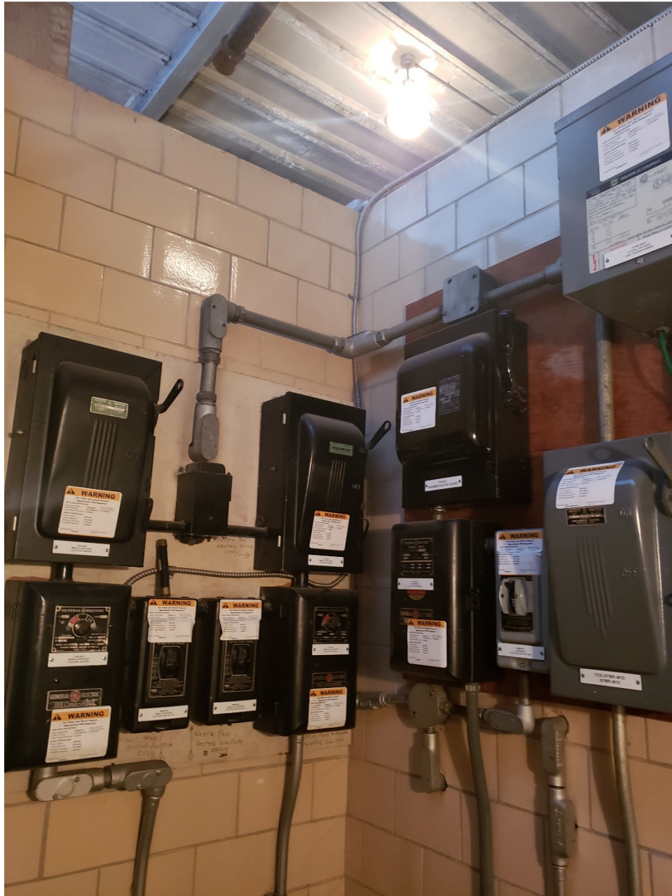
PHOTOGRAPH 38: Tache Booster Pumping Station – Main Level - facing northwest showing Tool Room.
