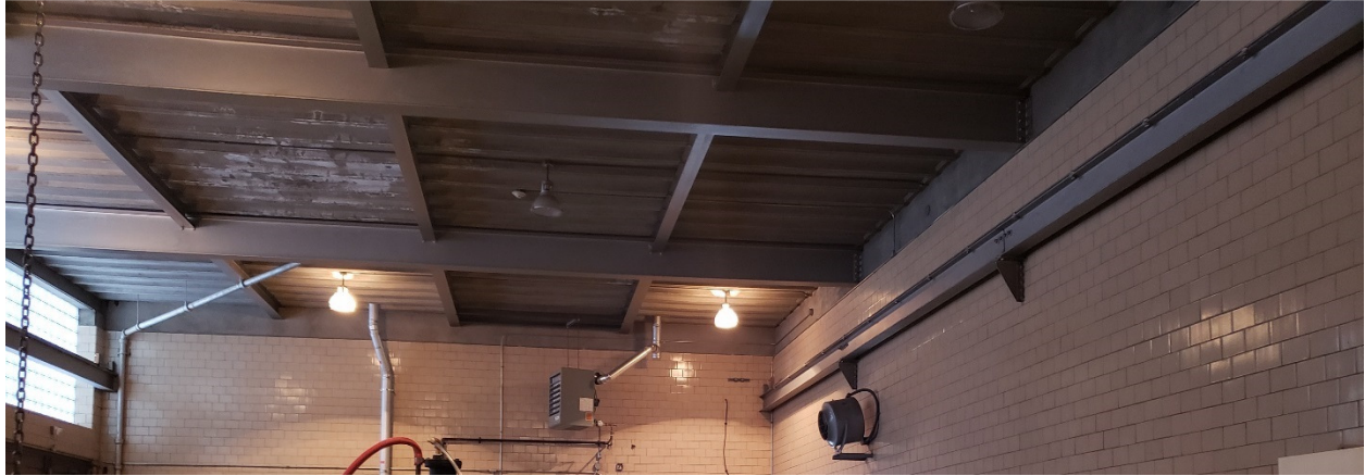
PHOTOGRAPH 35: Tache Booster Pumping Station – Main Level - facing southwest showing ceiling.
