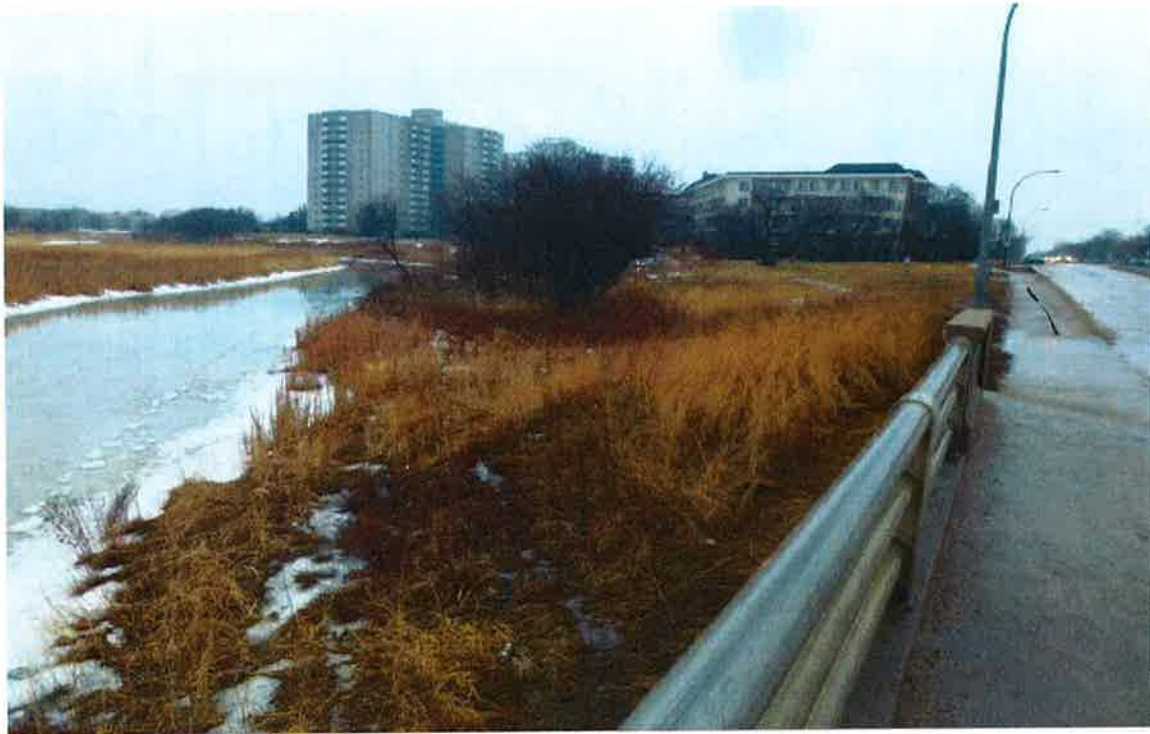
Photo 1: North-West Existing Bridge Abutment - Looking North
