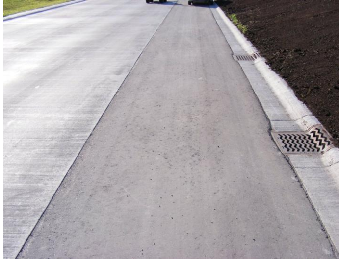
Figure 4.4 – Example of properly spaced fly-by catch basins.
