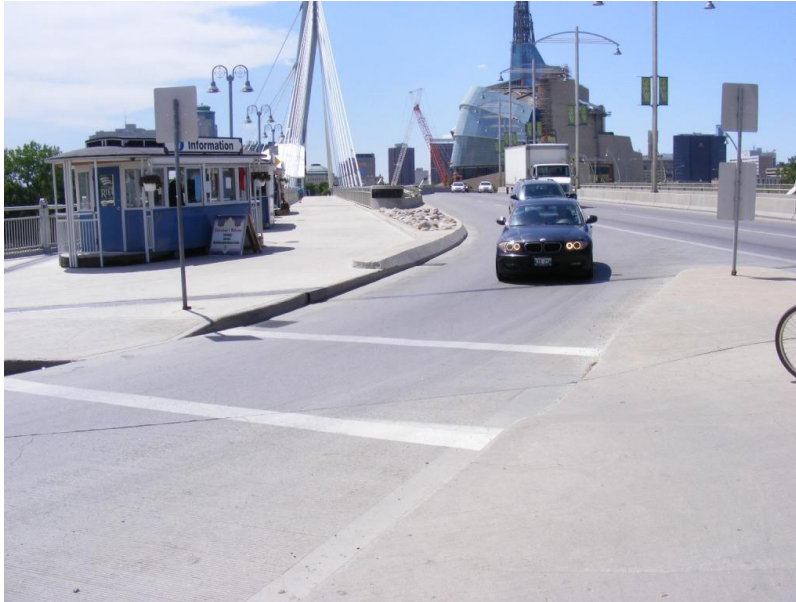
Figure 4.12 – Provencher Boulevard right turn onto Tache Avenue demonstrates how the downstream crossing allows for good sight lines for the driver.
