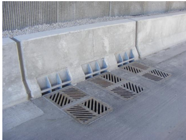
Figure 4.2 – Example of a way to maximize catchment efficiency at the low point of an underpass.
