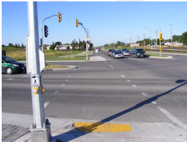
Figure 4.6 – Good median design on Chief Peguis Trail allows for the bullnoses to be placed adjacent to the pedestrian crossing.
