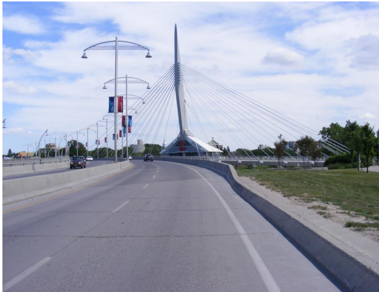
Figure 5.4 – F-shape barriers can be introduced by transitioning to a safety curb for lower speed roadways.
