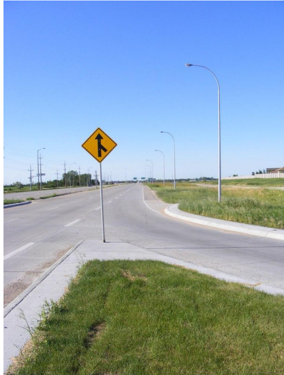
Figure 4.14 – Merging onto Lagimodiere Boulevard from Warde Avenue demonstrates proper curb termination that encourages driver comfort to merge
