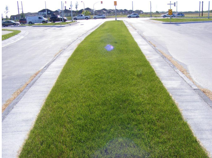
Figure 4.7 – Warde Avenue show the standard median design for developmental collectors and arterials that includes an integral modified barrier curb with a separate splash strip
