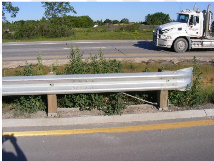
Figure 5.7 – A typical downstream end treatment for a W-beam guardrail
