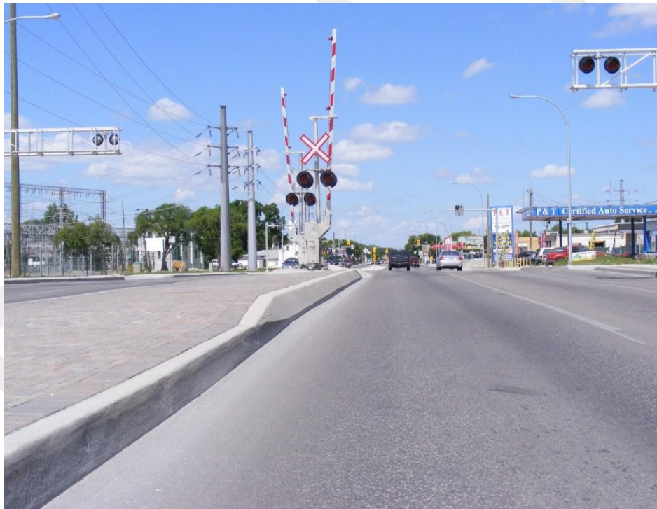
Figure 5.9 – Safety curb protection utilized at rail crossing on McPhillips Street
