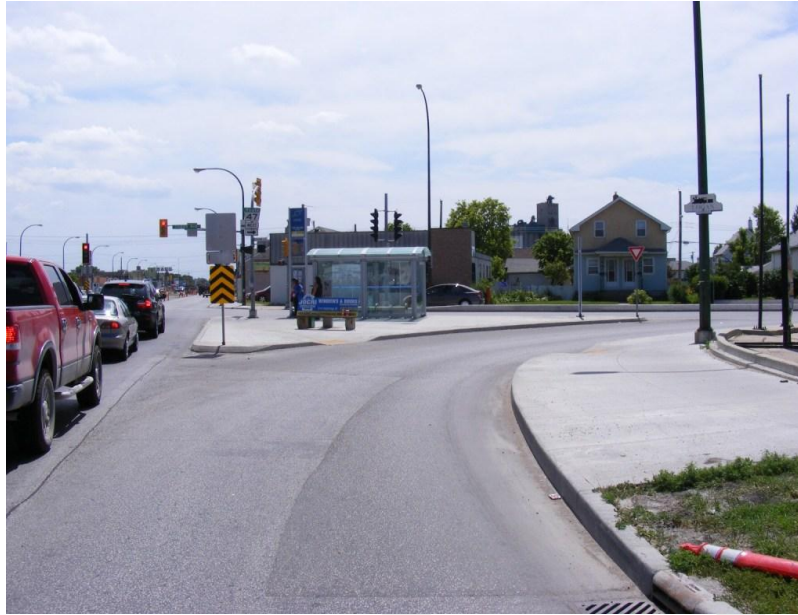
Figure 4.13 – McPhillips Street right turn onto Logan Avenue demonstrates the benefits of placing the pedestrian crossing upstream for visibility
