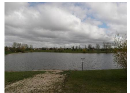
Typical City of Winnipeg retention pond
