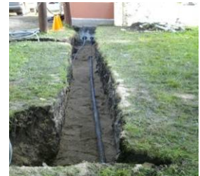
Typical trenching seen with permanent installation.
