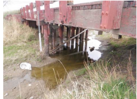
Drain site with bridge.
