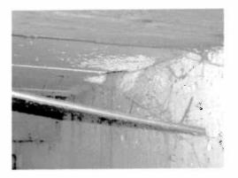
There are a number of areas where ducts are exposed and uninsulated due to the removal or damage of the plywood soffits.
