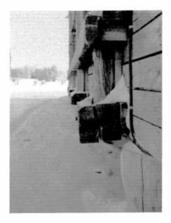
The foundations below the area beneath the building are made up out of concrete piles and grade beams. Wooden joists span across the grade beams at the exterior deck. The rest of the main floor soffit is insulated and covered with plywood.
