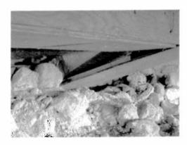
The foundations are comprised of one row of driven treated wooden piles along the exterior perimeter with the remainder of the foundations being cast-in place concrete friction piles.
