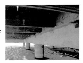
A number of the concrete friction piles were originally constructed with some honeycombing and there are a number of areas where the concrete grade beams also have honeycombing in them.
