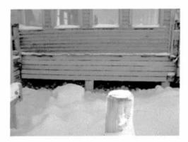
The section of timber pile, which is most at risk of undergoing rot, is that section of pile in the uppermost 300mm section below water level. Due to the frozen conditions, it was not possible to expose this section of pile. It is suggested that an additional inspection be undertaken once the spring thaw has occurred to determine the condition of the timber piles.
