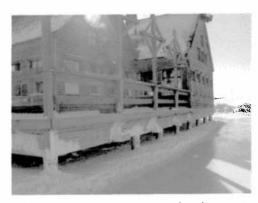
decking is comprised of 75x150 treated wood decking on 38x240 wooden beams.
