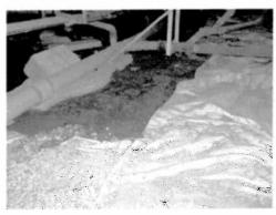
caused by intermittent flooding of the space, and likely a high water table due to the retention pond. The City could consider the installation of additional sump pits, and the installation of additional granular fill and ventilation; however, these measures will not solve the overall problem of flooding, they will only help to alleviate the moisture following a flood.
