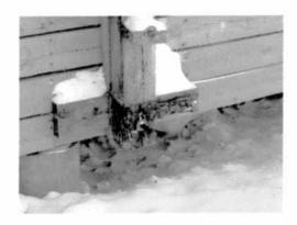
The lower 900mm of skirting around the building is made of pressure treated wood. The exposed tops of the piles appear to be in good condition.
