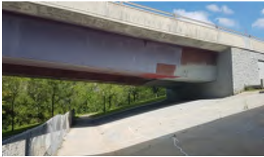
Path Under Bridge
