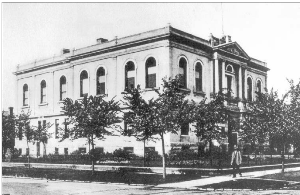
Plate 4 – Carnegie Library shortly after its addition, ca.1910. (Courtesy of the Provincial Archives of Manitoba, N1044.)
