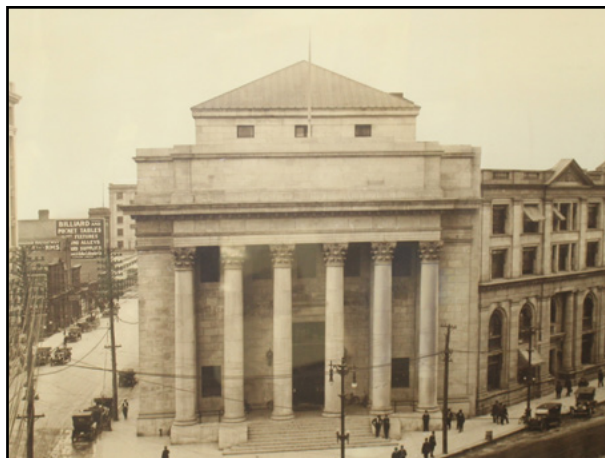
An early photograph of the Bank of Montreal Building, 335 Main Street, showing the original metal roof. (Bank of Montreal)
