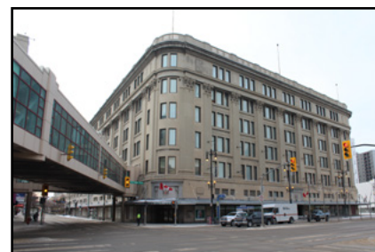
The Bay, 450 Portage Avenue, north and east façades, 2021. (M. Peterson)
