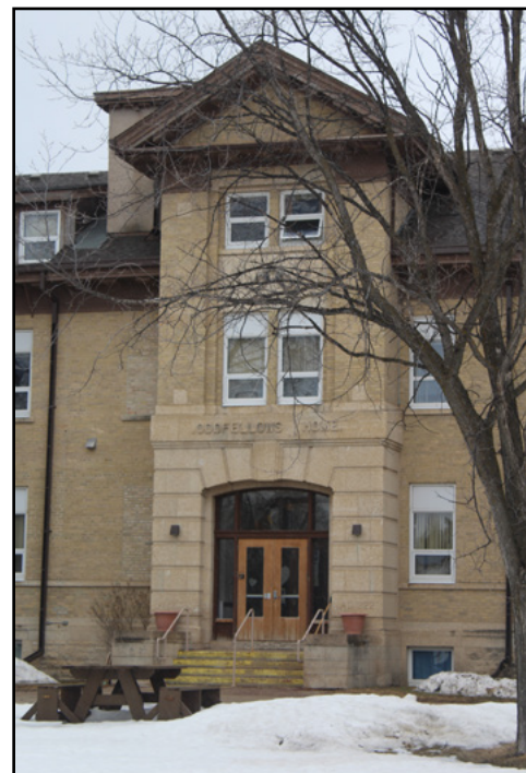
IOOF Home, 4025 Roblin Boulevard, detail of front (south) entrance, 2022. (M. Peterson)
