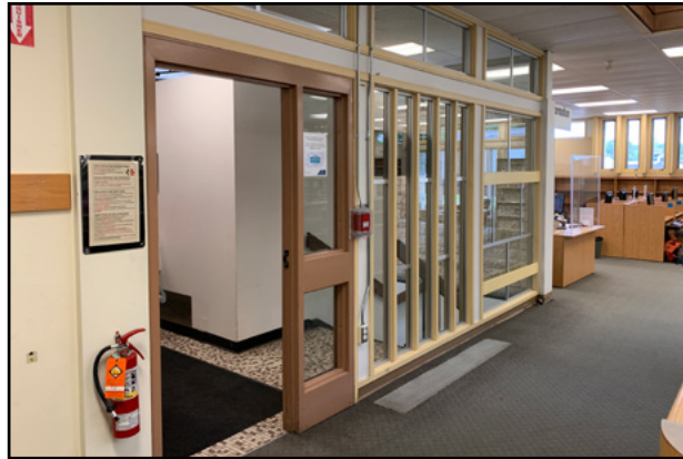
West Kildonan Public Library, 365 Jefferson Avenue, original rear staircase detailing, 2021. (M. Peterson)
