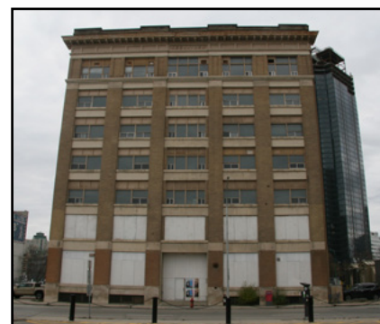
Keewayden Block, 138 Portage Avenue East, front (north) façade, 2021. (M. Peterson)
