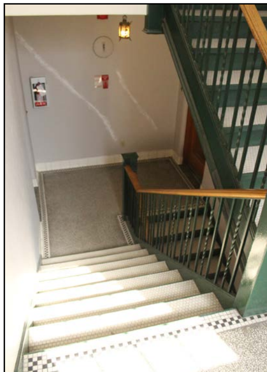
Locarno Apartments, 1 Roslyn Road, main staircase, Building B
