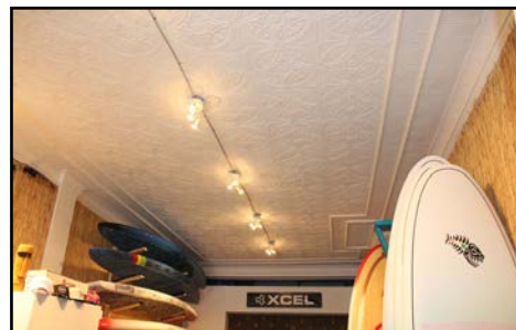
Johnstone Block, 209 Pacific Avenue, retail store tin ceiling
