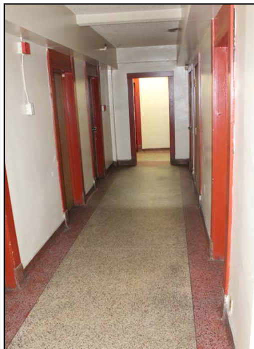
McLaren Hotel, 554 Main Street, second floor hallway
