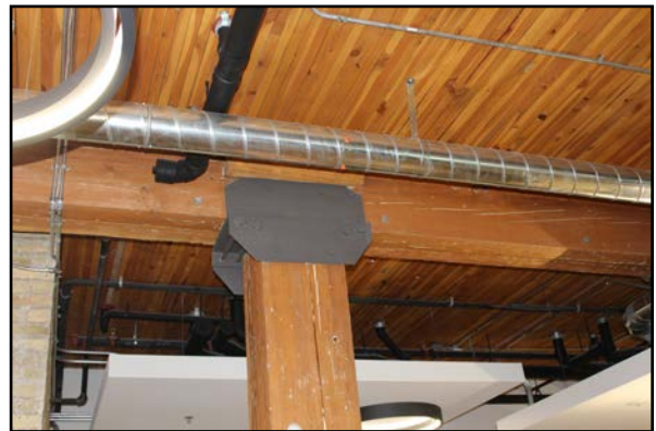
Stanley Brock Building, 145 Market Avenue, structural support system, ground floor
