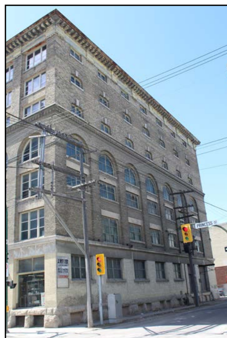
Cockshutt Plow Company Building, 238 Princess Street, north façade
