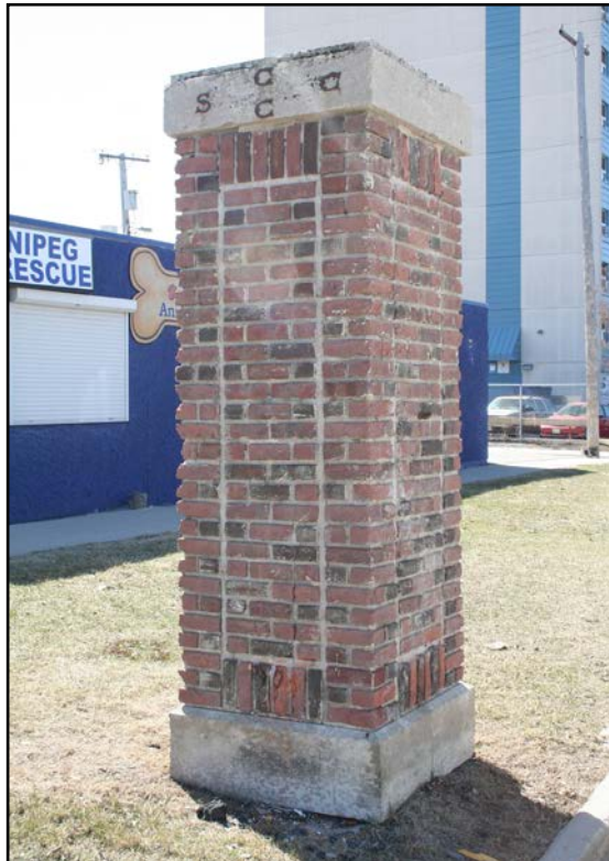
Street pillar, Portage Avenue at Country Club Boulevard
