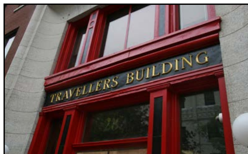
Western Building, west façade, prior to renovations
