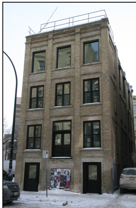
Western Building, west façade, today
