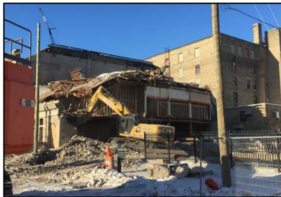
Thomas Scott Memorial Orange Hall, demolition in progress
