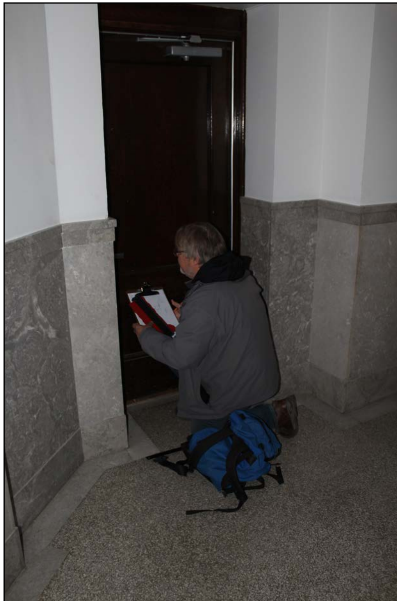
Historical Buildings Officer G. Menzies measuring interior elements, Administration Building, University of Manitoba, 66 Chancellors Circle
