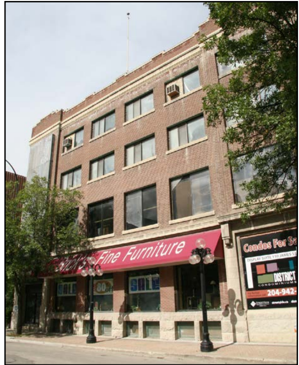
Stanley Brock Building, 145 Market Avenue
