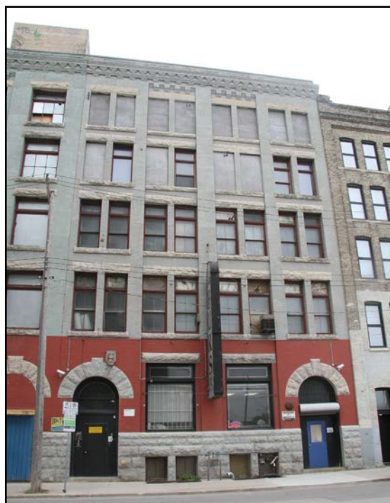
Trees-Spriggs Building, 312 Ross Avenue
