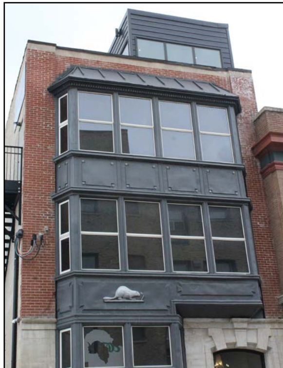
Douglas & Company Building, 52 Adelaide Street, detail of front (east) façade
