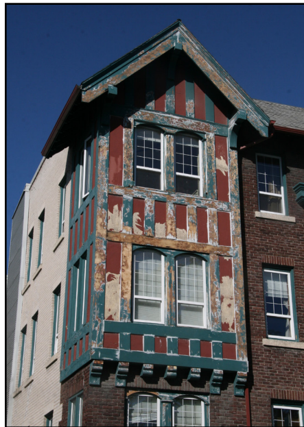
Thelma Apartments, preparation work completed for exterior painting
