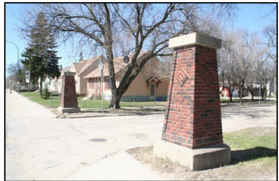
Street pillars, Henderson Highway at Helmsdale Avenue, from the north
