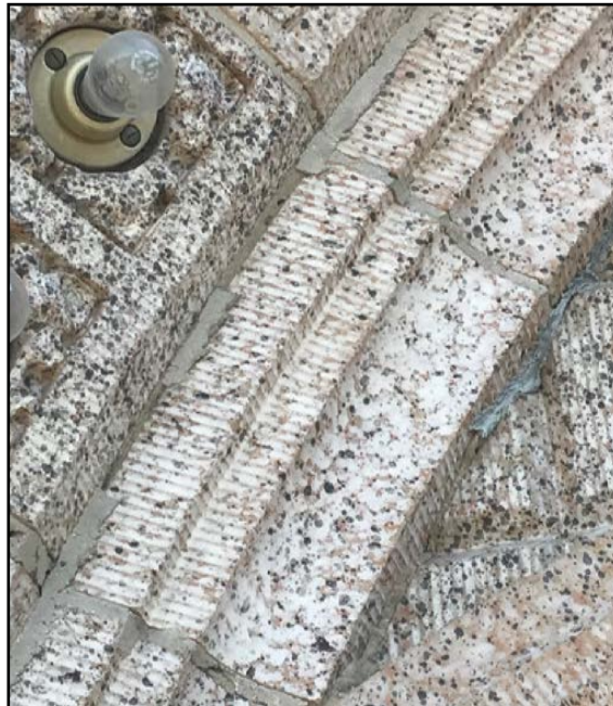
Electric Railway Chambers, terra cotta (Courtesy of Crosier Kilgour & Partners)
