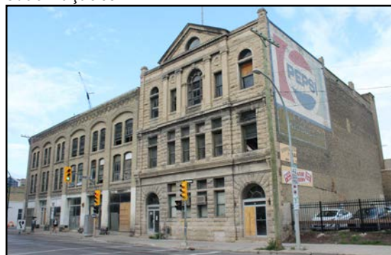
206-210 and 216 Princess Street, front (east) and north façades
