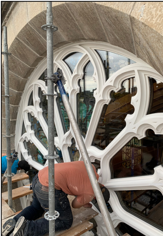
Westminster United Church, rose window installation
