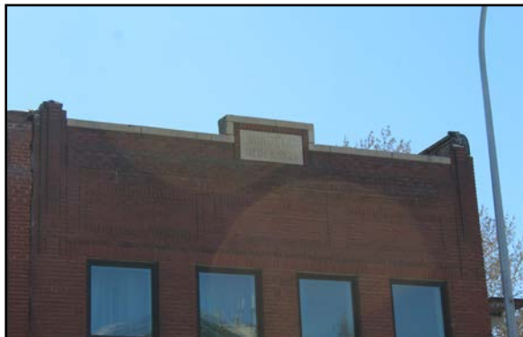
Mindell Block, 607 Main Street, front (west) façade detail
