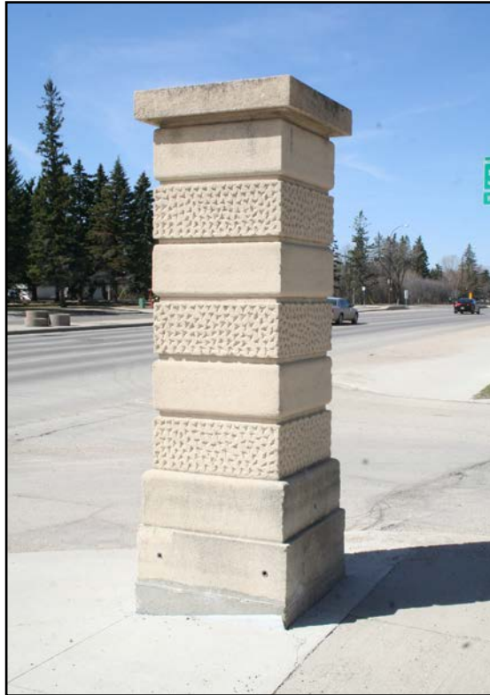
Street pillars, Portage Avenue at Moorgate Street, east pillar
