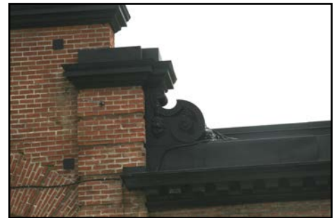
Hudson's Bay Company Garage, 115 Garry Street, front (west) façade detail
