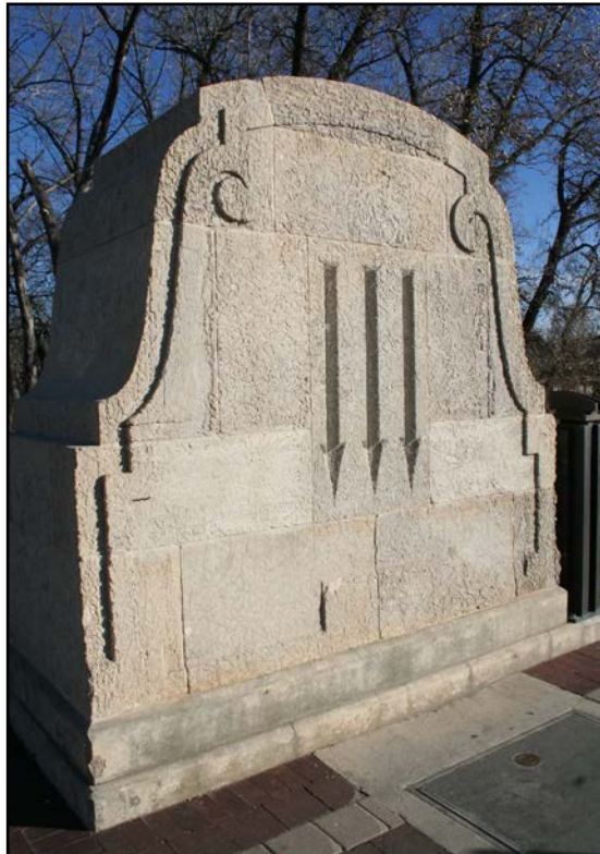
Main Street Bridge, limestone pylon
