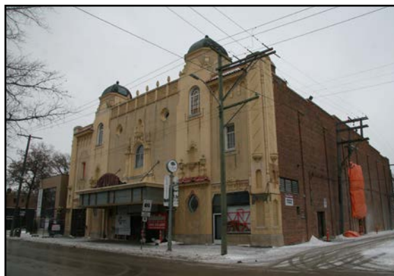
Uptown Theatre/Lanes, restoration of front (north) façade underway
