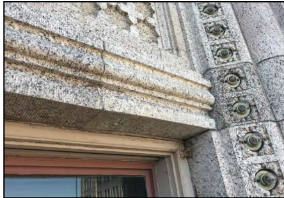
Electric Railway Chambers, terra cotta (Courtesy of Crosier Kilgour & Partners)
