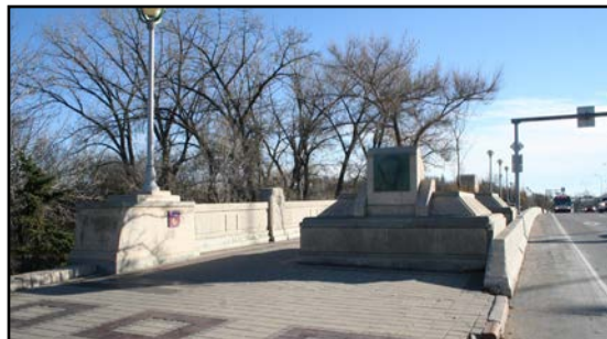
Main Street Bridge, limestone wall
