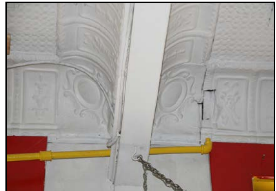
Leadlay Building, 306-310 Ross Avenue, ornamental tin ceiling on the first floor
