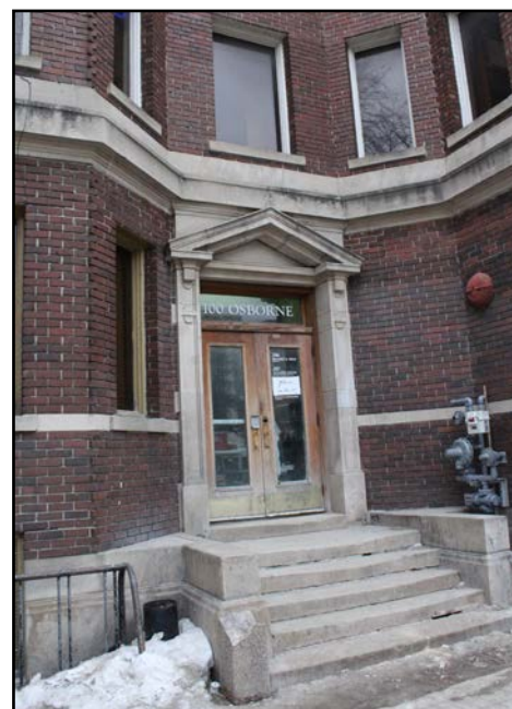
Osborne-River Building, 100 Osborne Street, northeast entrance
