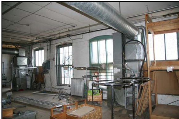
Leadlay Building, 306-310 Ross Avenue, fourth floor space
