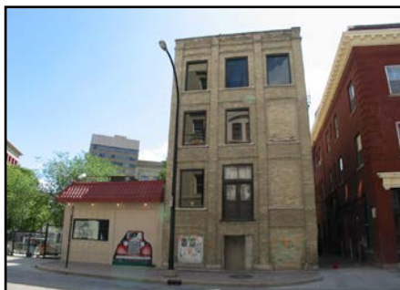
Western Building, west façade, prior to renovations
