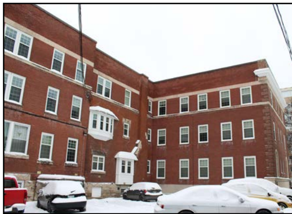
East façade, Rossmore Apartments, 80 Roslyn Road
