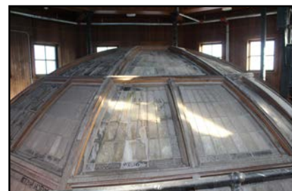
Administration Building – University of Manitoba, 66 Chancellors Circle, interior dome in cupola
