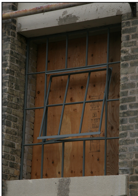
Scott Fruit Company Warehouse, original metal windows on east façade
