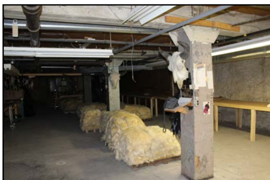
Trees-Spriggs Building, 312 Ross Avenue, basement
