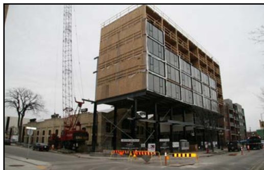
James Avenue Pumping Station, east side apartment building
