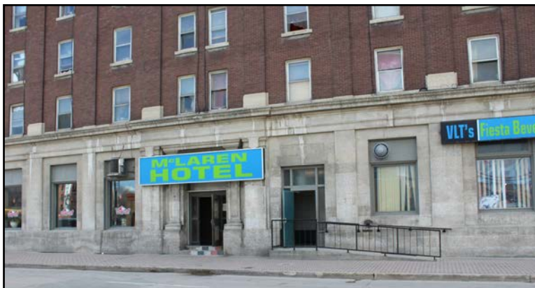
McLaren Hotel, 554 Main Street, detail of north entrances
