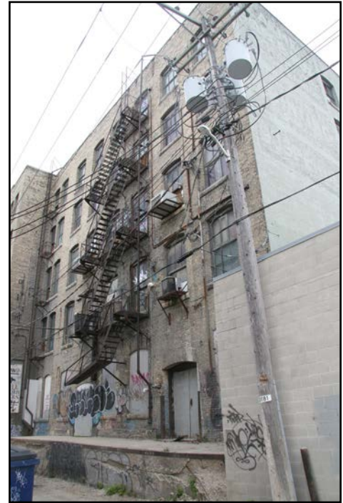
Leadlay Building, 306-310 Ross Avenue, rear (south) façade
