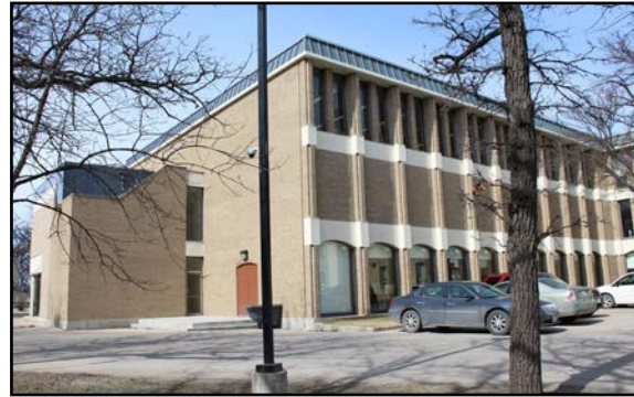
St. Mary's Academy, 550 Wellington Crescent, 1963 addition, south and east façades
