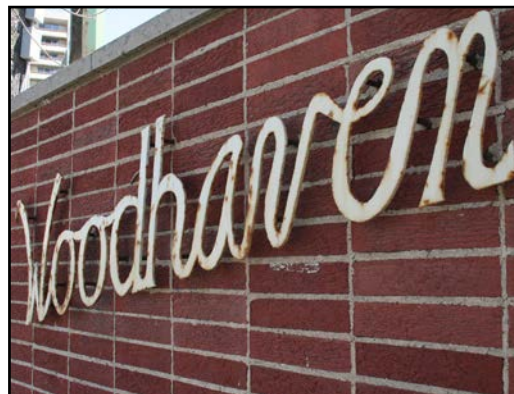
Gate, Portage Avenue at Woodhaven Boulevard, west façade detail
