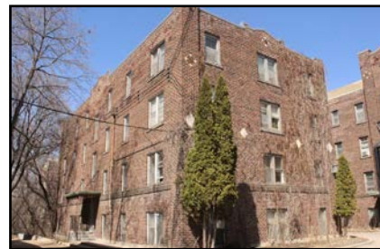
Locarno Apartments, 1 Roslyn Road, Building A
