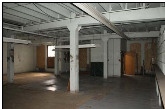
Trees-Spriggs Building, 312 Ross Avenue, 3rd floor
