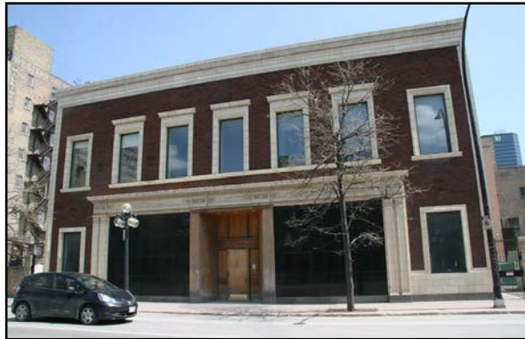
Winnipeg Hydro Showroom, 55 Princess Street
