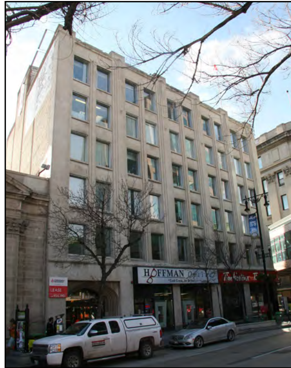
Power Building, 428 Portage Avenue
