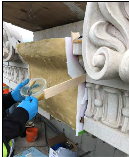
Plastic moulding of the damaged terra cotta section
