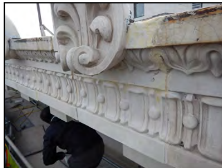
New terra cotta piece in place, known as a "Dutchman Repair"
