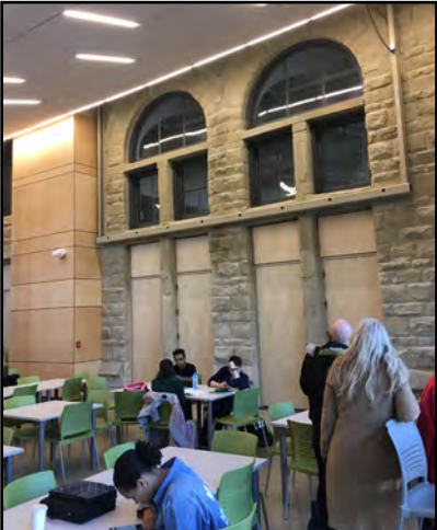
Second floor cafeteria space at the new Leatherdale Hall, University of Winnipeg, with exposed exterior wall of the original building
