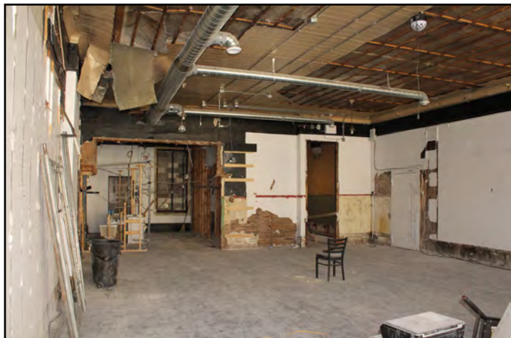
Third floor of the Leckie Building
