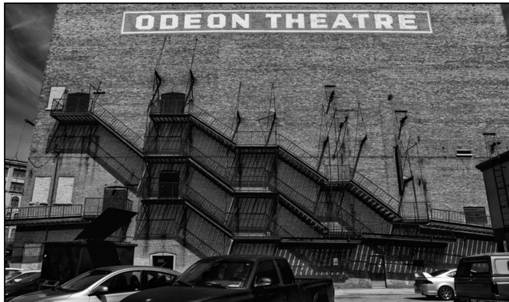
Old painted signage and metal fire escape on the north elevation of the Burton Cummings Theatre, Smith Street (G. Cline)
