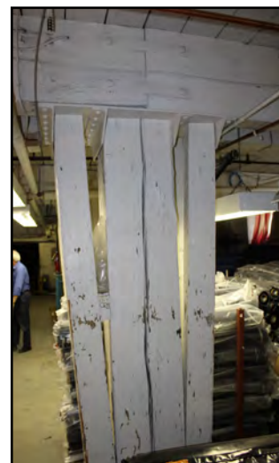
Example of the heavy mill construction, Miller, Morse and Company Building
