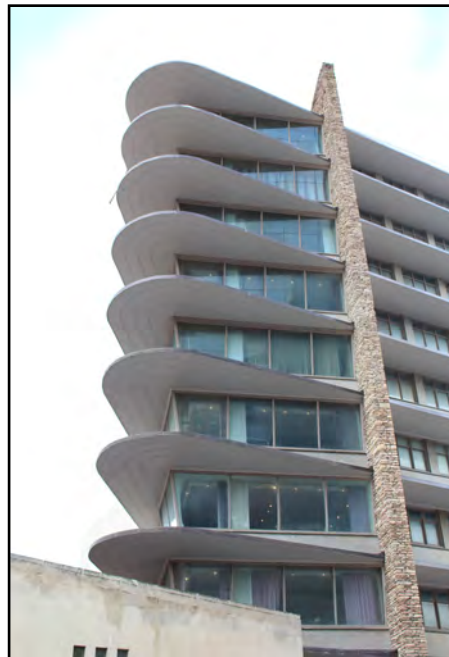
Detail of the exterior windows, southwest corner, Winnipeg Clinic
