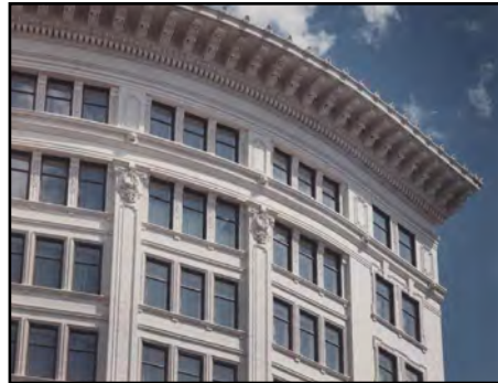
Close up of the cornice and Main Street façade
