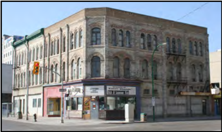
MacDonald and Fortune Blocks, 224-234 Main Street, with the original metal cornice still attached to the MacDonald Building
