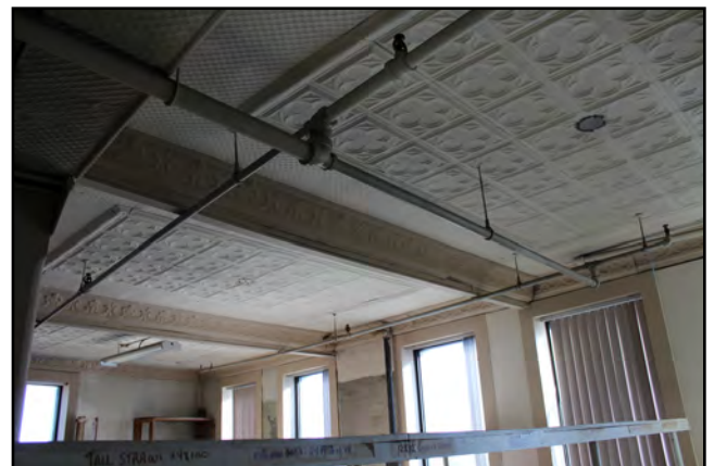
Original ornamental tin ceiling, 3rd floor, Scott-Bathgate Building
