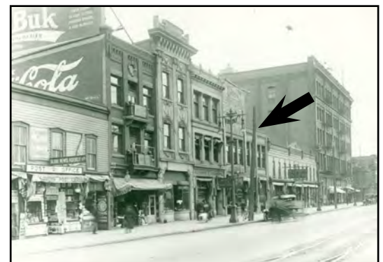
East side of Main Street from Logan Avenue to Henry Avenue, 1918. The Calder Building, 661 Main Street, is at the arrow. (Archives of Manitoba, Outsize 728, Winnipeg-Streets- Main 1.)
