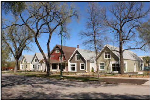
51 Balmoral Street, Milner Residence (centre), part of the new daycare facility
