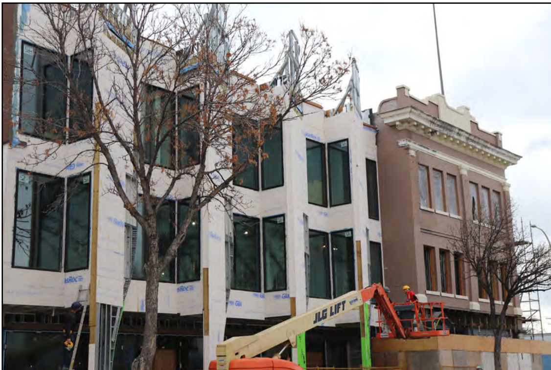
Work continuing on the renovation of the Merchants Hotel, 2017
