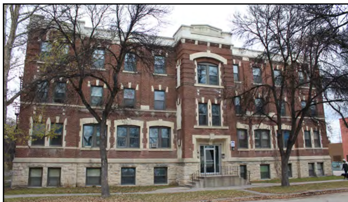
Church Block Apartments, 259 Church Avenue
