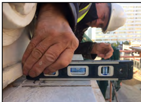
Restoration work continues on the NWCTA Building, fall 2017
