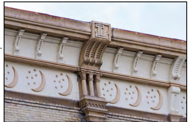
Detail of metal roof, I.O.O.F. Hall, 72 Princess Street (G. Cline)
