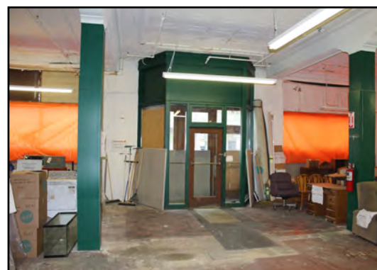
Ground floor entrance, south end, 208 Princess Street
