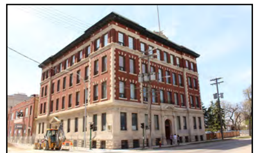
Manitoba Telephone System – Garry Exchange, 474 Hargrave Street
