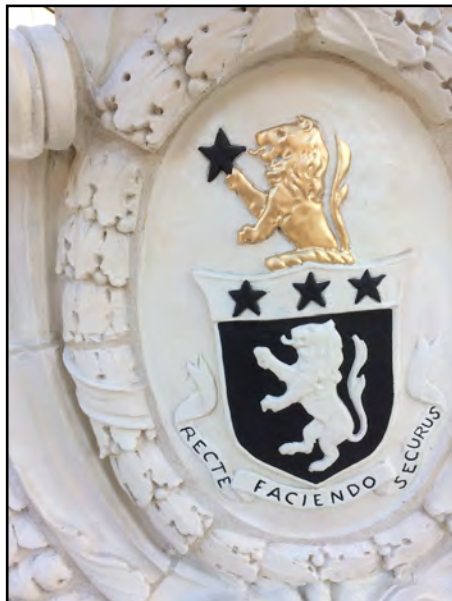
Detail of the fully restored crest, NWCTA Building
