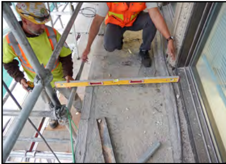
Workmen on site
