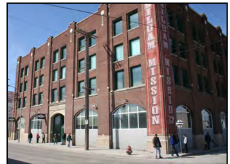
Canadian Fairbanks Morse Company Warehouse, 300 Princess Street
