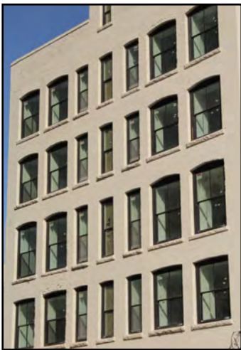
272 Main Street, Scott Block, window replacement on the rear (west) façade
