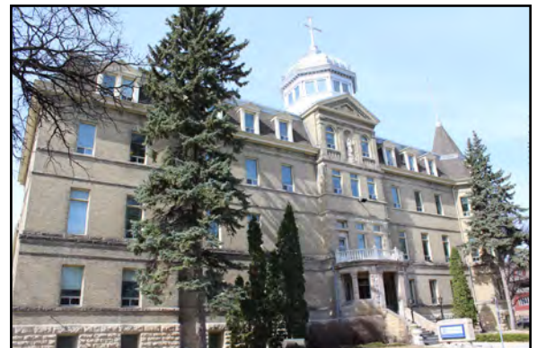
Front (north) façade of the 1902 St. Mary's Academy, 550 Wellington Crescent
