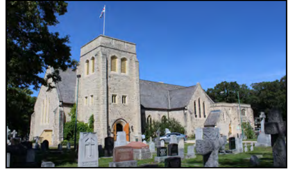
St. John's Anglican Church and Cemetery, 135 Anderson Avenue
