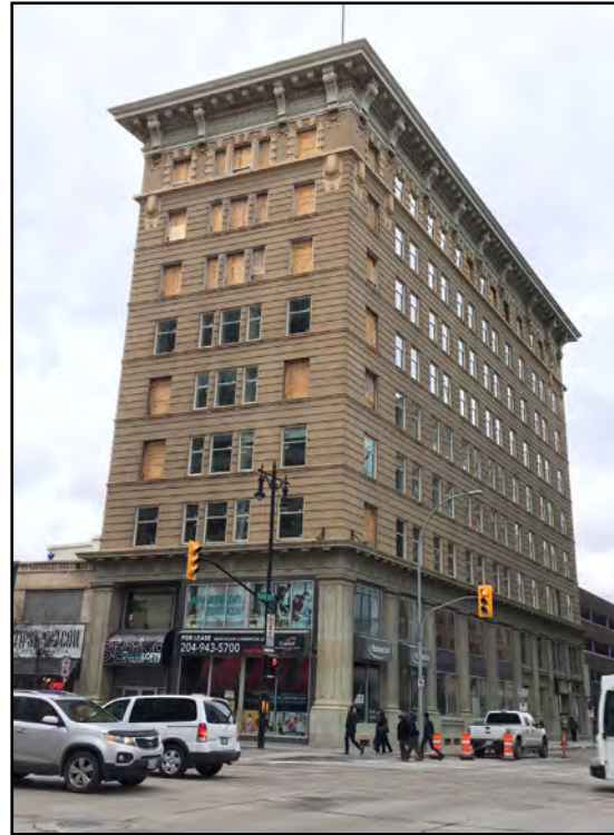
Sterling Bank Building, 283 Portage Avenue during renovations and window replacement, fall, 2017
