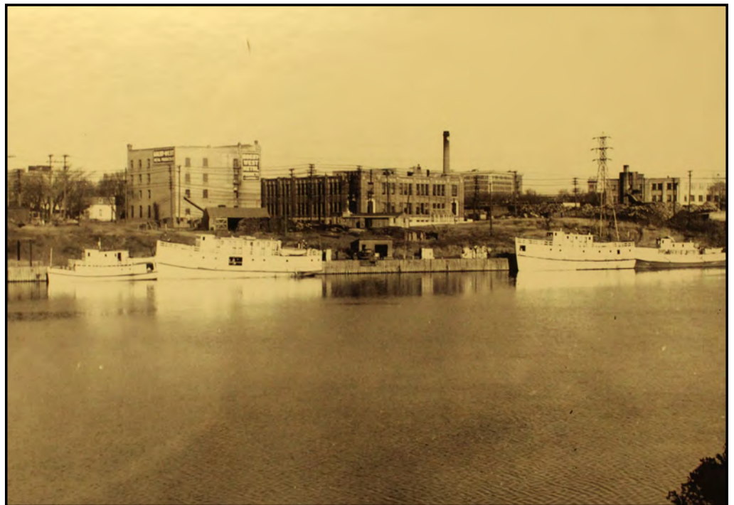
Looking from the St. Boniface side of the Red River with the Alexander Docks in the foreground and Great West Metal Company Building on the left, ca.1940.
