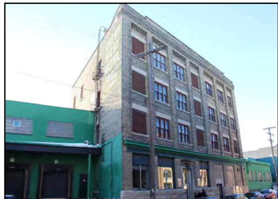
Great West Metal Company Building, 90 Alexander Avenue
