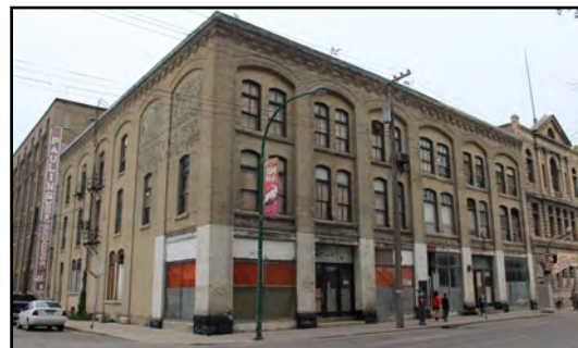
208 Princess Street, McLaughlin Motor Car Company Building
