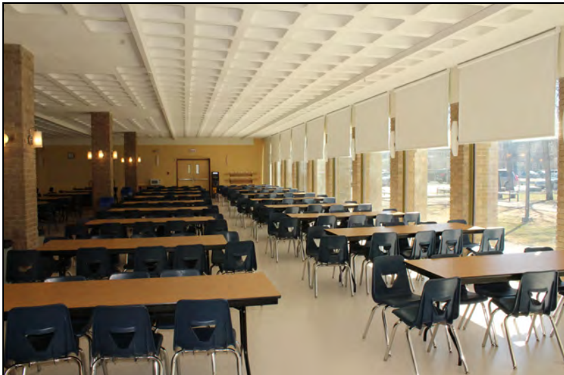
Interior of cafeteria with original waffle ceiling, 550 Wellington Crescent
