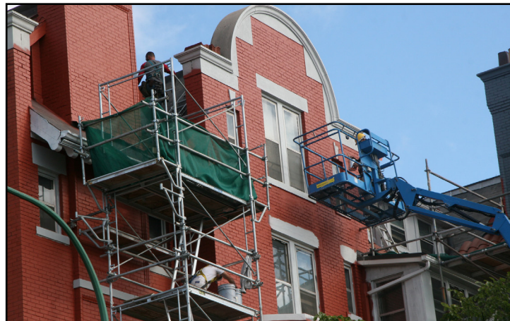
Workers on Roslyn Court Apartments, 40 Osborne Street, September 2015
