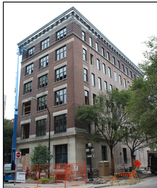
Major renovation work continues at the Porter Building, 165 McDermot Avenue
