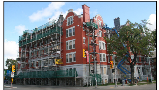
Scaffolding on the Roslyn Court Apartments, 40 Osborne Street, September 2015
