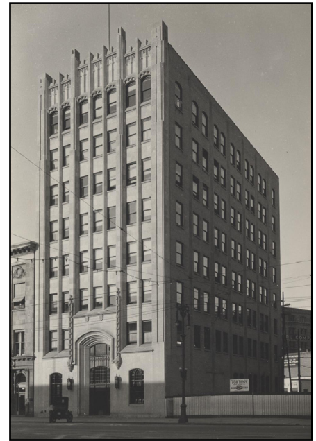
423 Main Street, Canadian Wheat Board Building shortly after original construction in 1928
