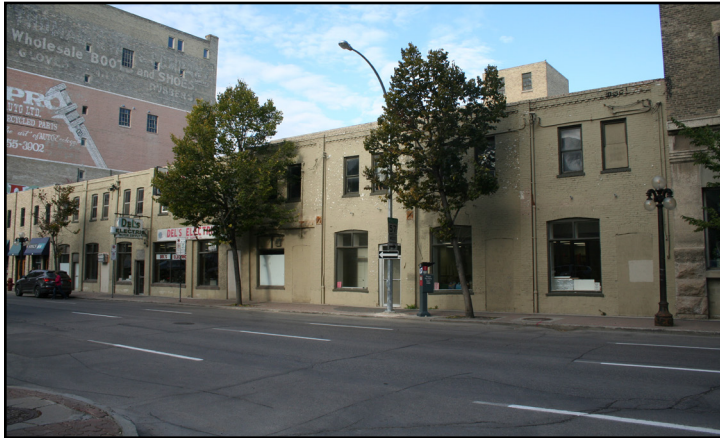
54 & 62 Princess Street, Del Block and Annex
