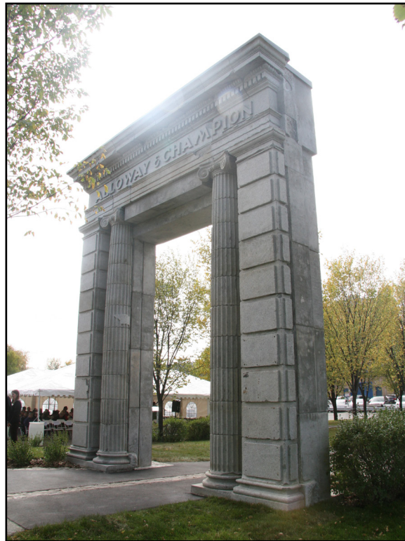
The rebuilt Alloway Arch at The Forks, September 2015
