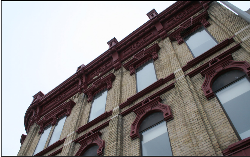
Part of the front façade of the Maycock Block, 586 Main Street
