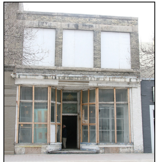
284 William Avenue, Winnipeg Saddlery Building
