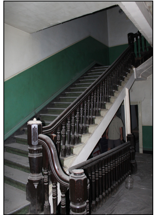
Second store landing and bannister of the main staircase, Fortune Block
