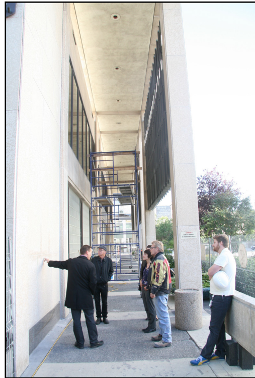
Committee members reviewing repointing work at Winnipeg City Hall, 510 Main Street
