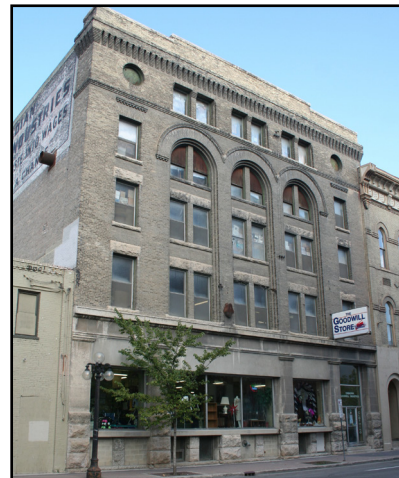
Bole Drug Company Warehouse, 70 Princess Street
