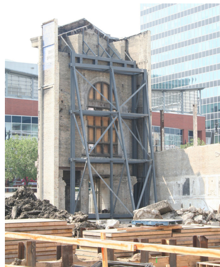
Façade of the Mitchell Copp Building with its steel bracing.
