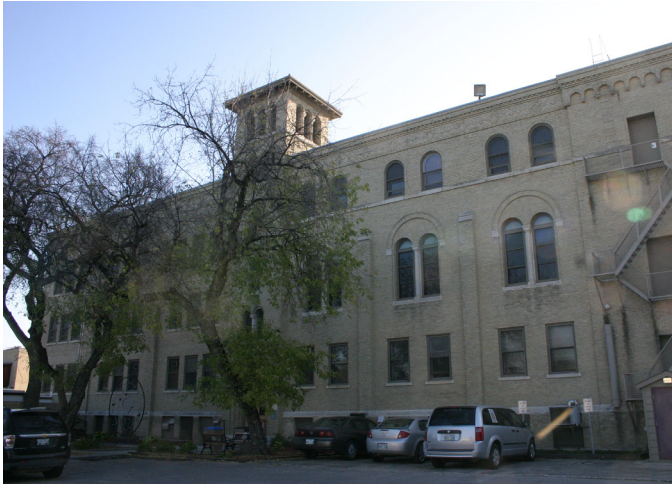
442 Scotia Street, Marymount, former St. Agnes Priory
