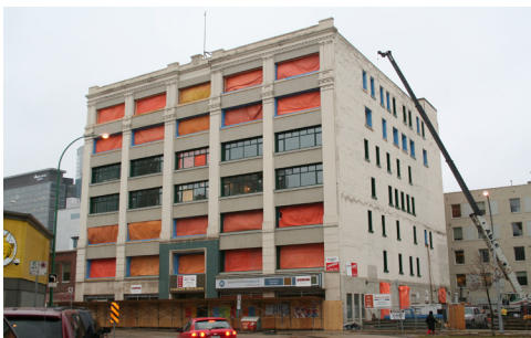
Extensive interior and exterior work on the Canada Building, October 2012.
