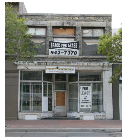
284 William Avenue prior to the boarding up of the windows
