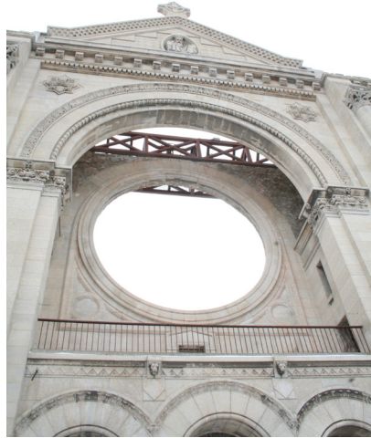
St. Boniface Cathedral, ruins of front (west) façade
