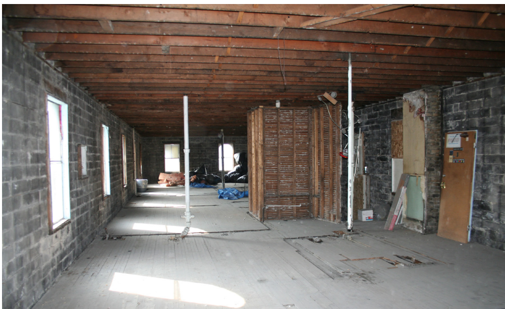
Gutted second floor of the Craik Block
