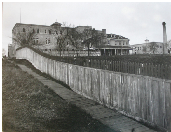
This undated photograph of the Marymound School complex from the riverbank shows the house in the foreground, the Priory behind and the boiler house/laundry to the right. (Courtesy of Marymound.)
