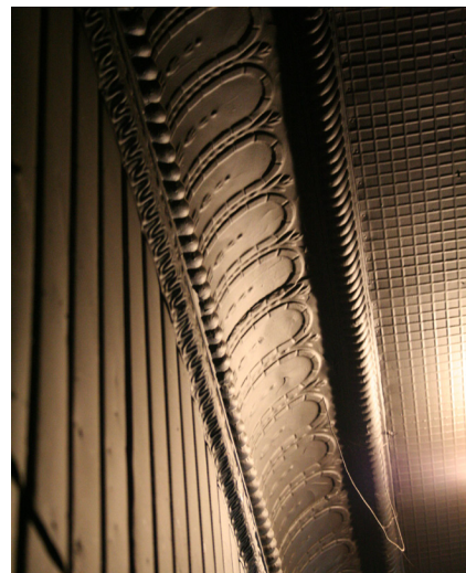
Ornamental tin on the walls and ceiling of the first floor, Weir Block
