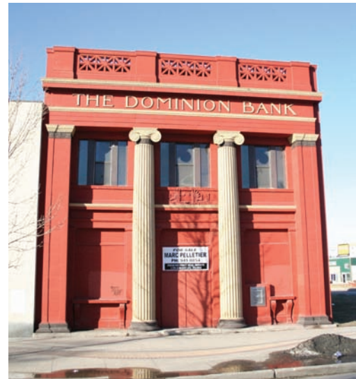
Dominion Bank Building prior to renovations
