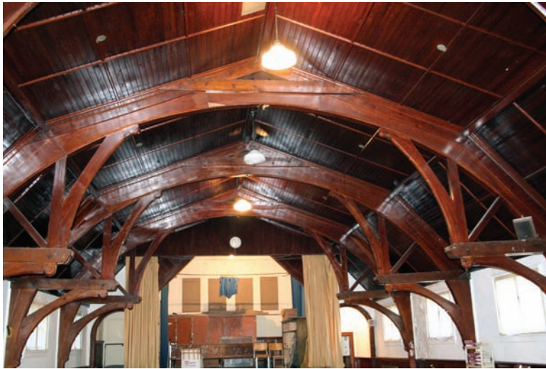
The magnificent hammerbeam ceiling of the former St. John's Anglican Church Parish Hall
