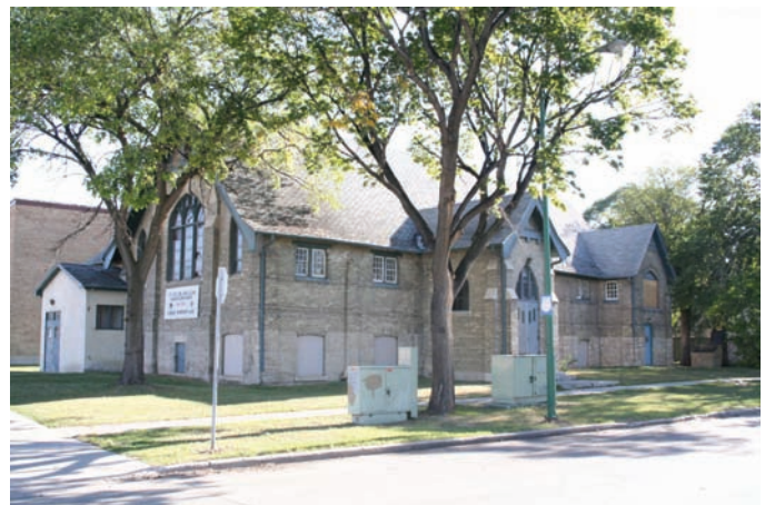
Former St. John's Anglican Church Parish Hall, 181 Church Avenue
