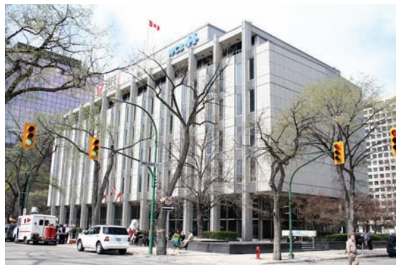
One of Winnipeg's fine Modern Style buildings is the former Monarch Life Building, 333 Broadway
