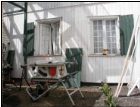
Window repair at St. Boniface Museum
