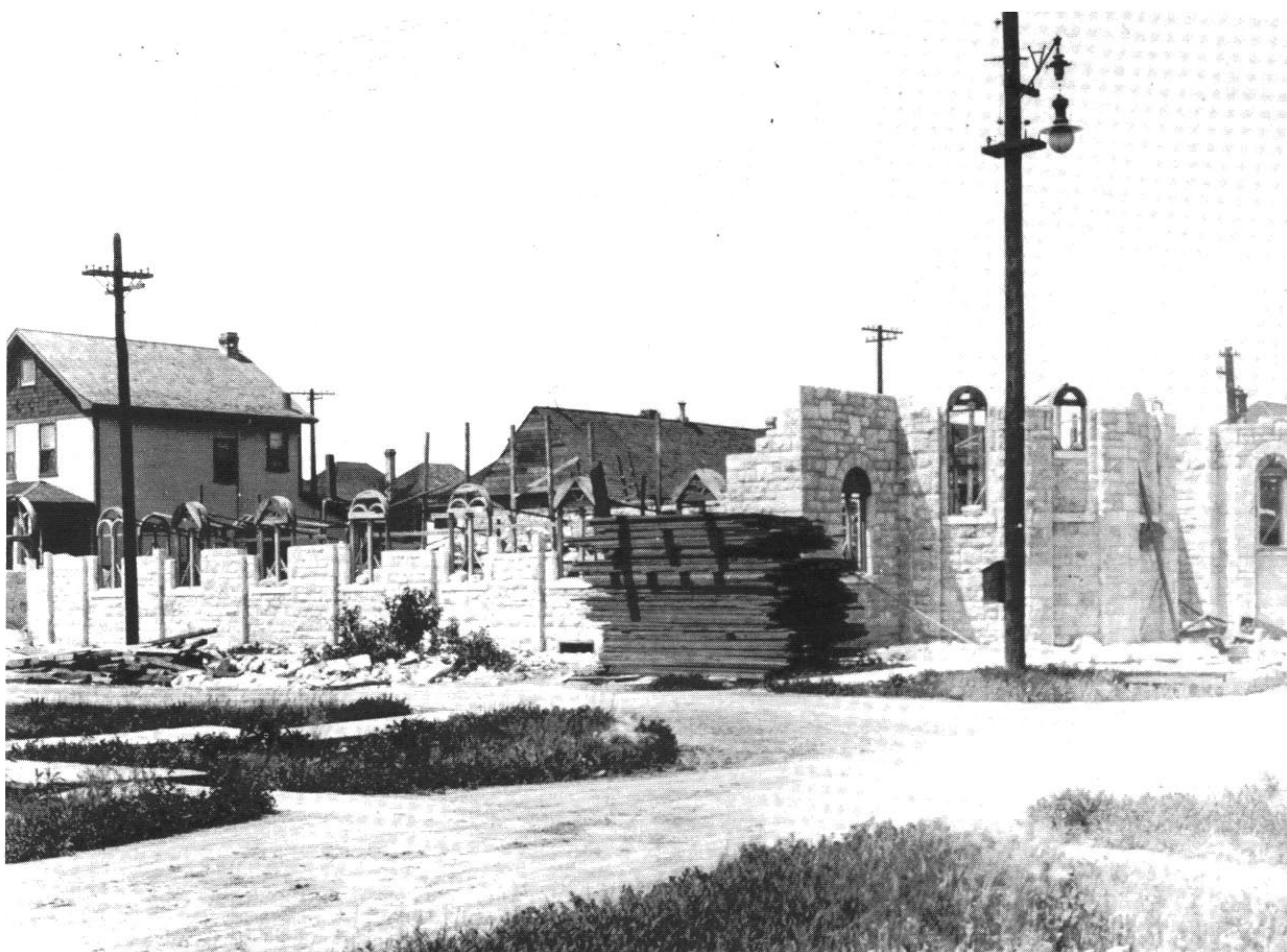
Construction of the church, 1920. St. Michael and All Angels Archives
