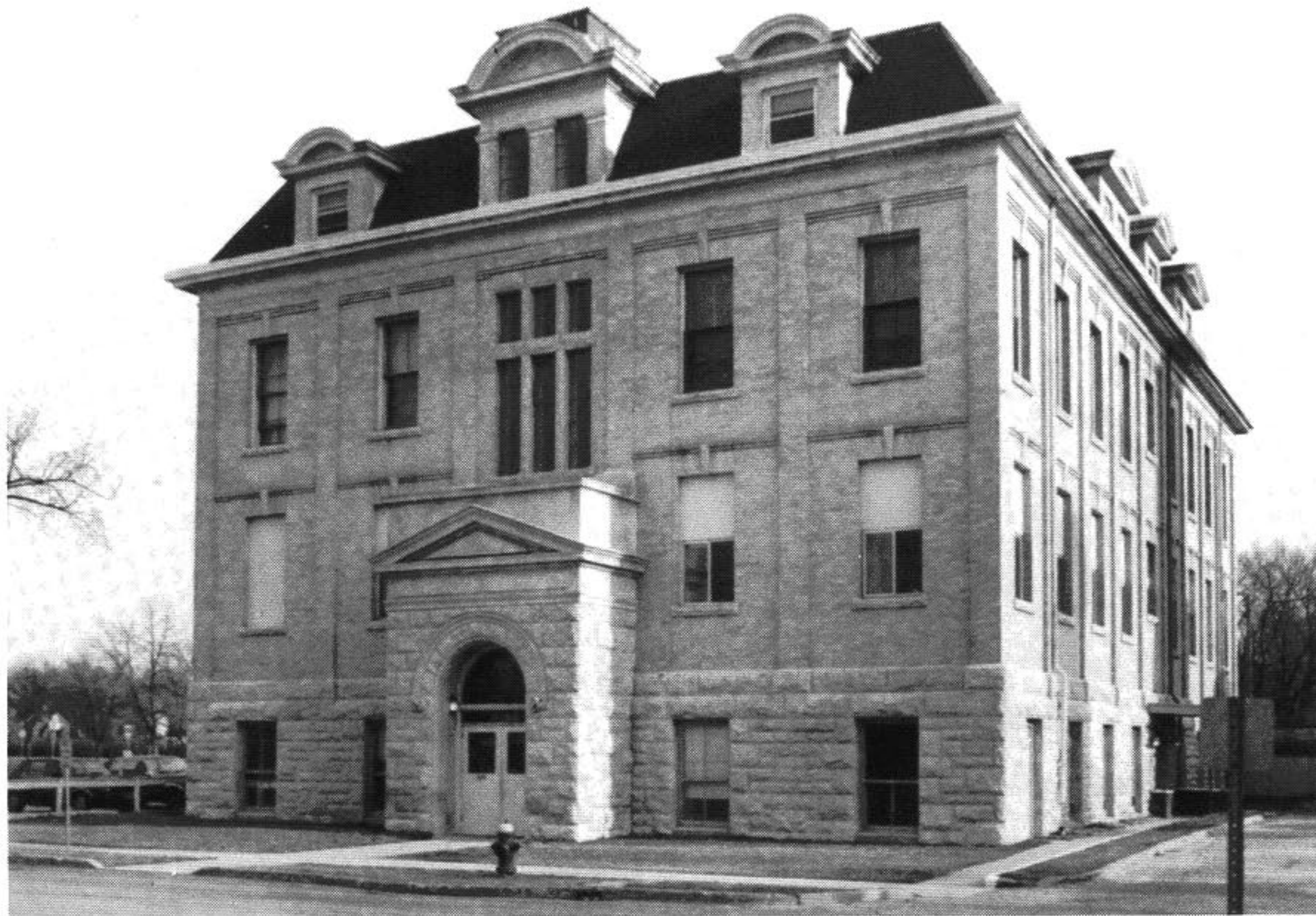
The Dairy and Science Building, 1989. City of Winnipeg
