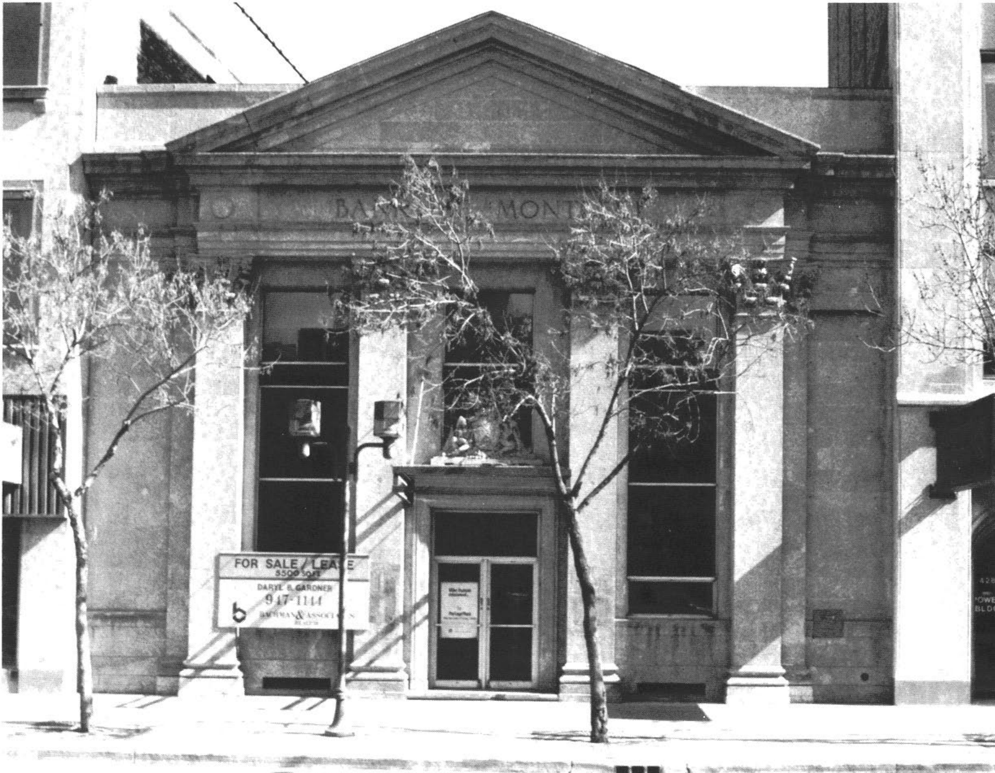
The Tyndall stone facade of the former Bank of Montreal, 1989. City of Winnipeg
