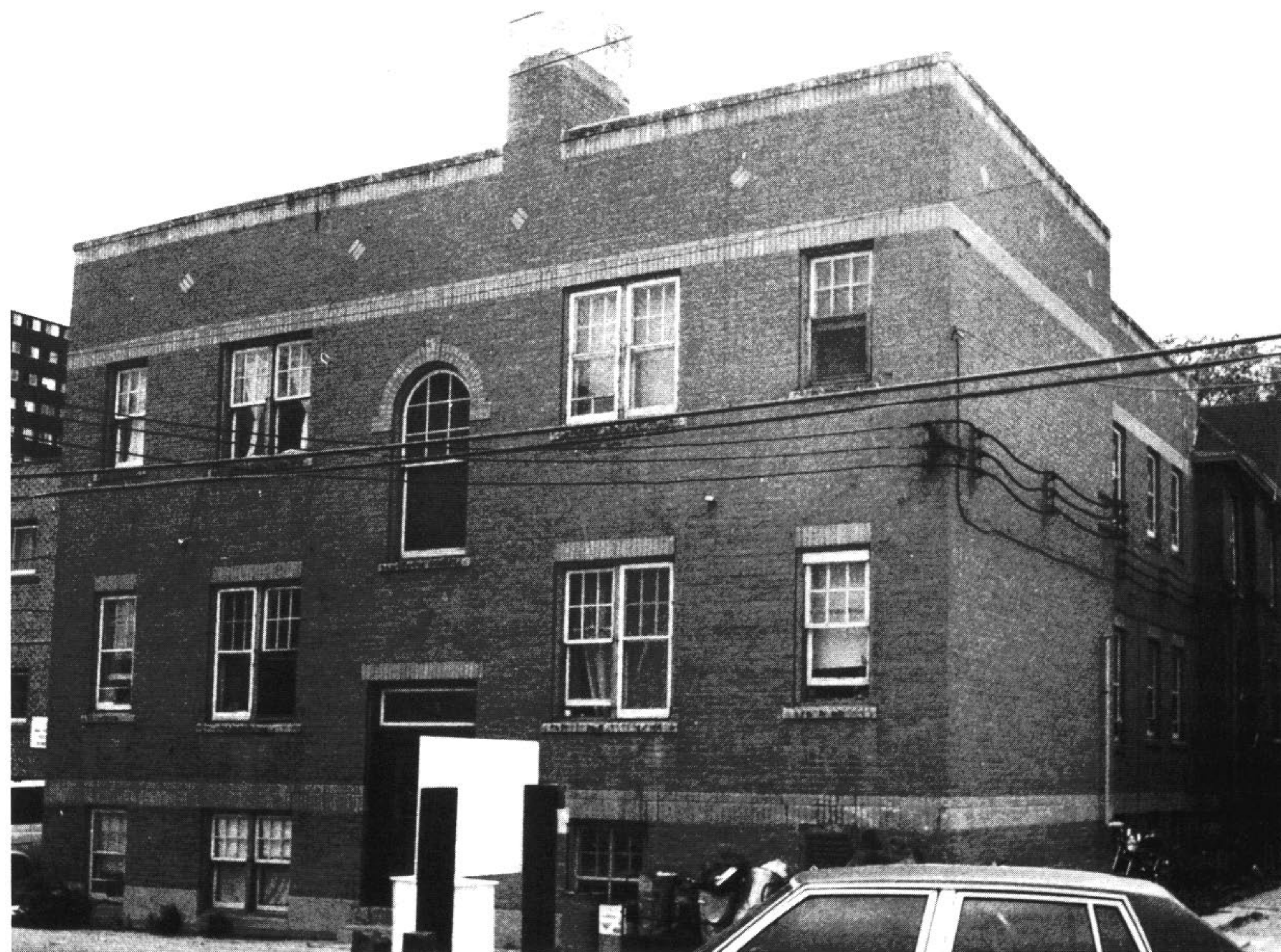
The 1928 addition at the rear of the house. City of Winnipeg
