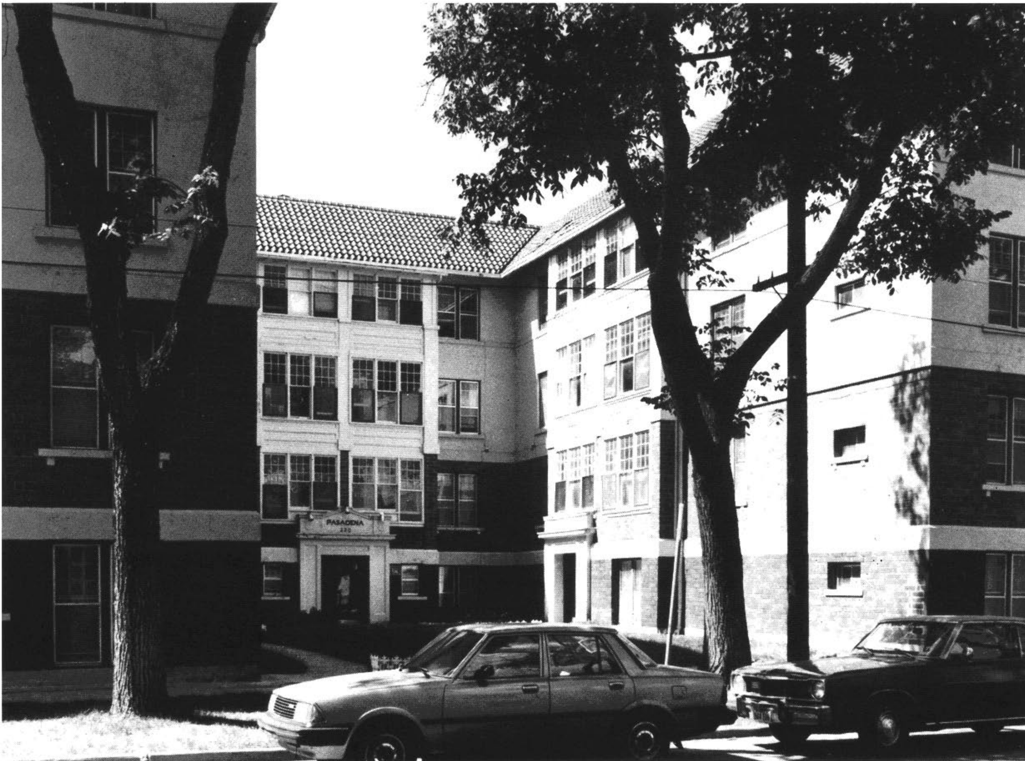
The courtyard of the Pasadena Apartments, 1988. City of Winnipeg
