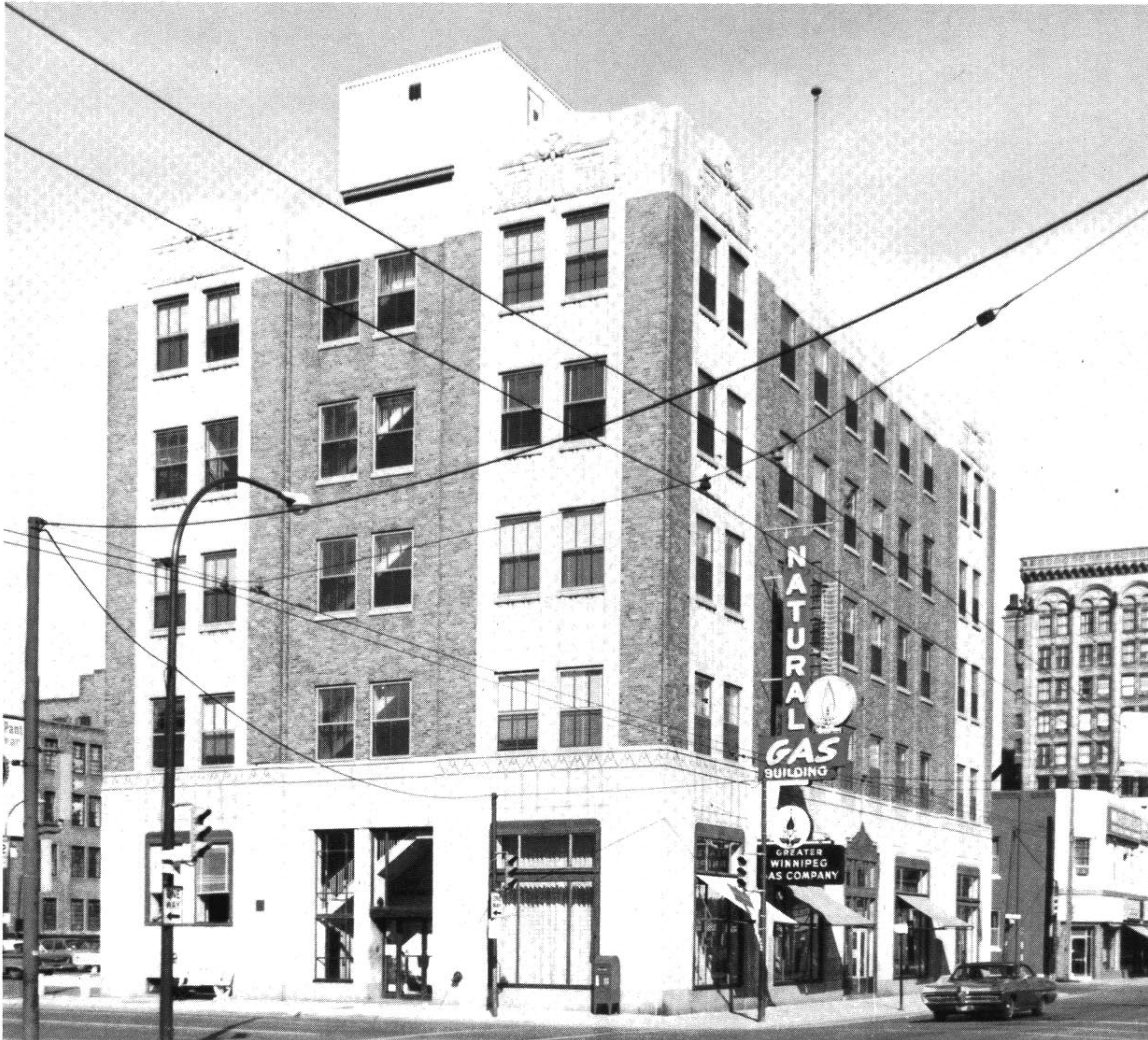
The Winnipeg Gas Company Building, 1970. Provincial Archives of Manitoba
