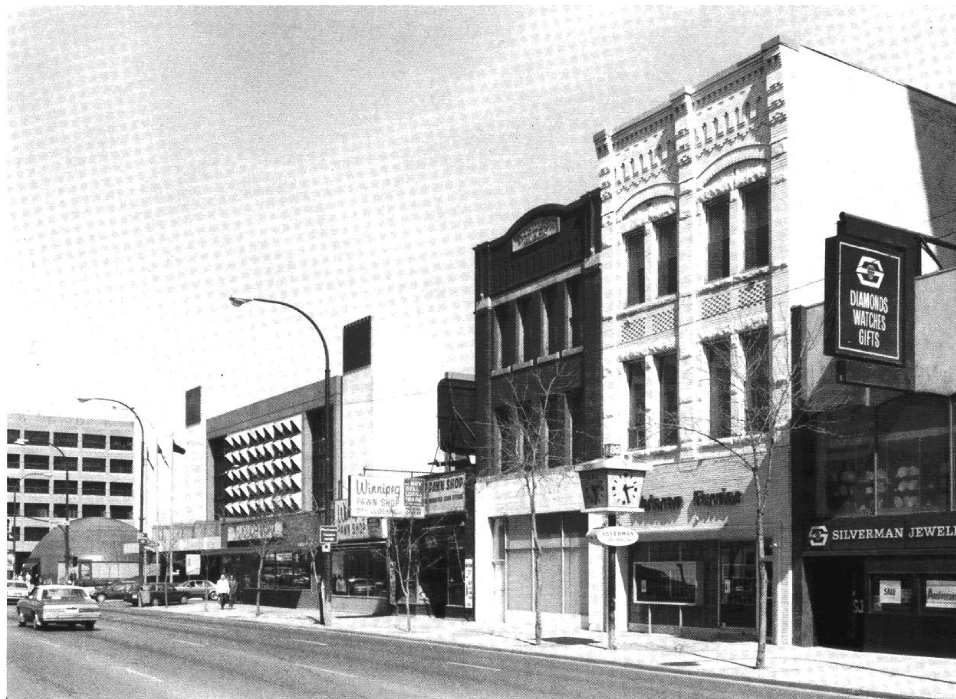
A view of Main Street showing the Macpherson and Thomson Blocks in 1988. City of Winnipeg
