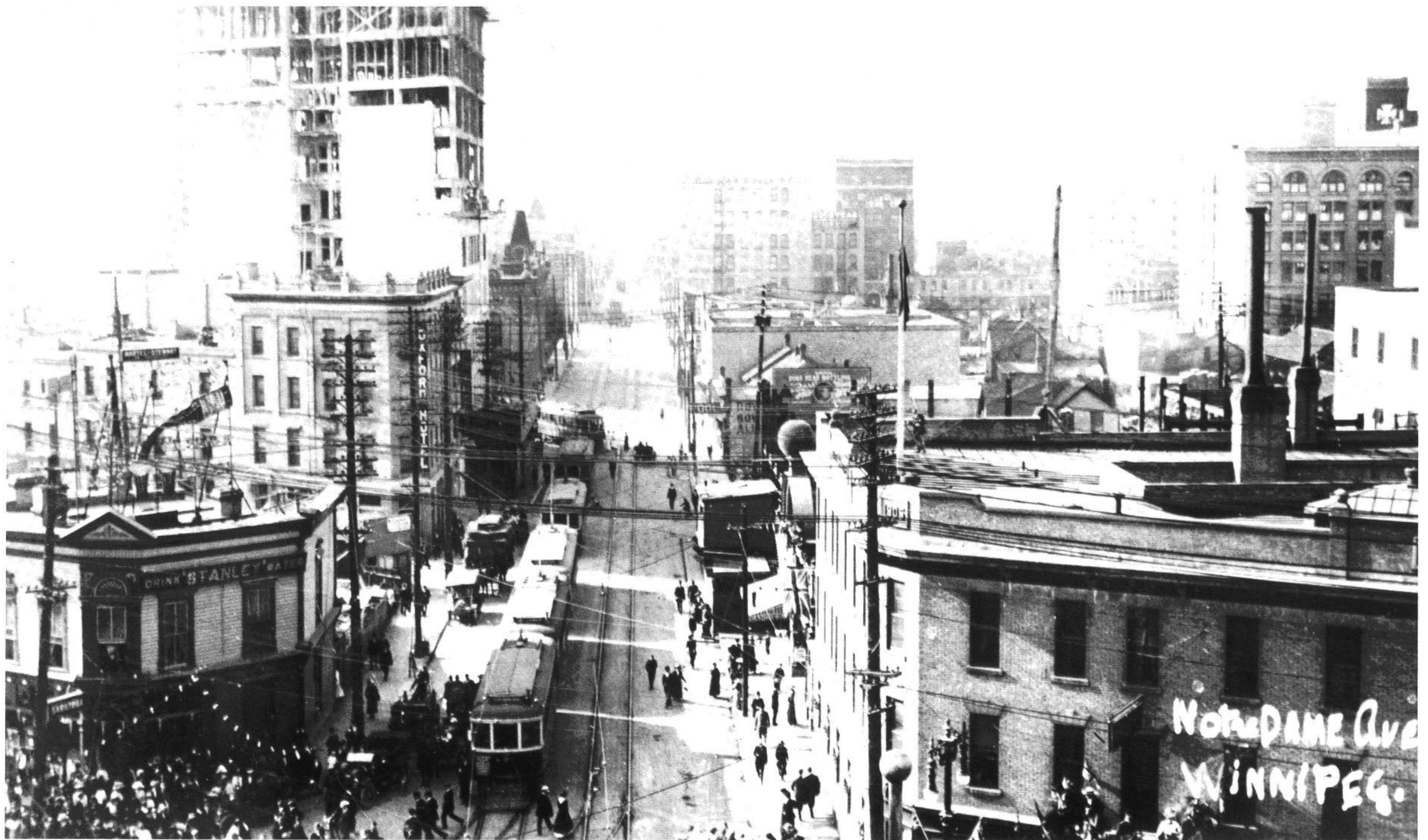
A view of Portage and Notre Dame avenues during construction of the Lindsay Building, c.1911. Provincial Archives of Manitoba
