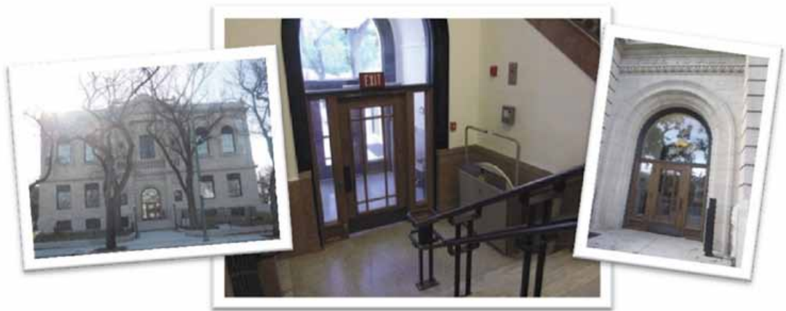
380 William - Renovations to the front entrance and foyer completed in the fall of 2011.
