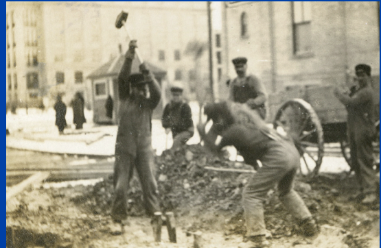
Workers excavate near the General Hospital (Health Sciences Centre) on Bannatyne Avenue, 1914.
