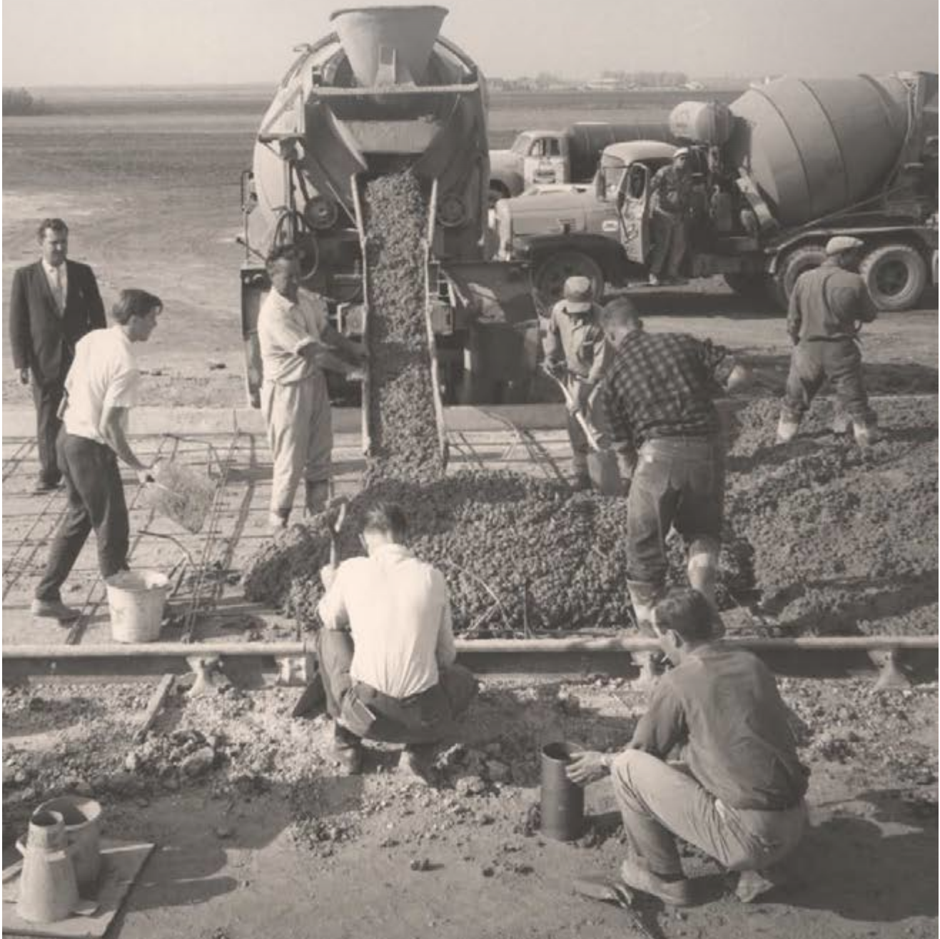
Road work on Waverley Street, October 17, 1963. Photo credit: David Portigal.
