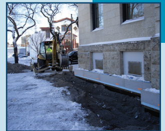
Foundation waterproofing project at 380 William.
