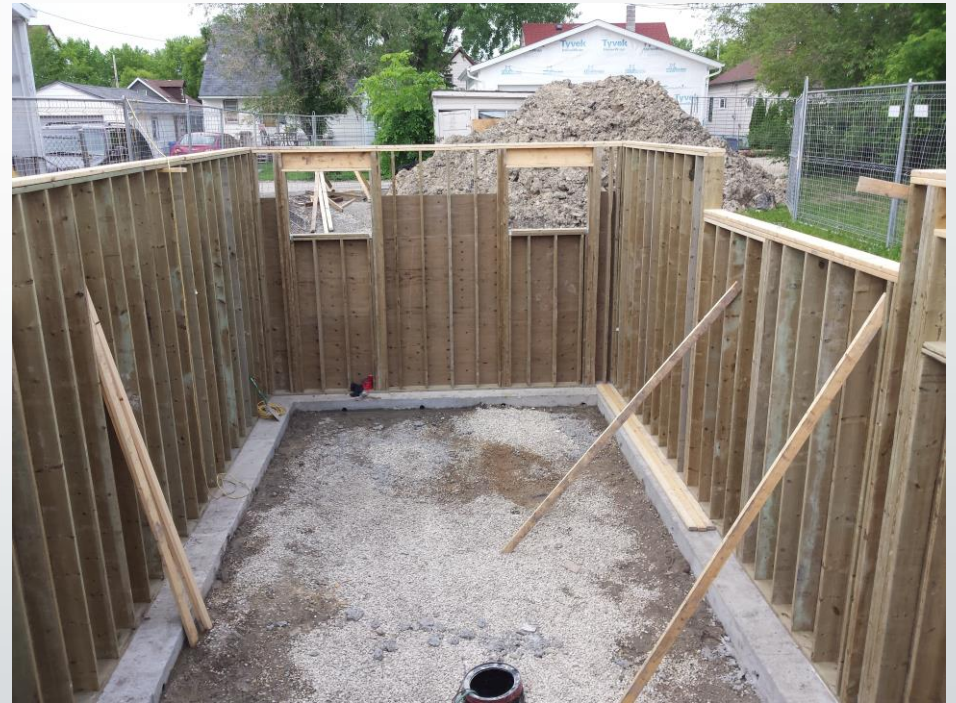
Foundation – PWF walls
