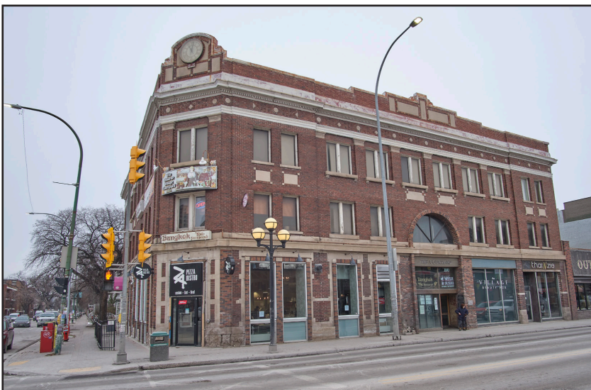
Osborne-River Building, 100 Osborne Street. (G. Cline)
