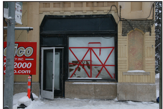
Work continuing on the west store front, 2020. (City of Winnipeg)
