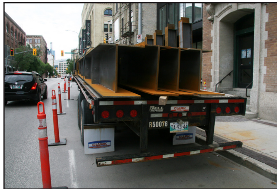
Warehouse, 104 Princess Street, delivery of the Corten steel for application to the 1950 warehouse, 2020. (City of Winnipeg)
