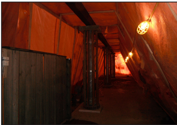
Winter construction work on the pergola under tarps, 2020. (City of Winnipeg)
