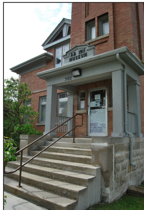
Front steps and façade of Assiniboia Municipal Hall, 3180 Portage Avenue.
