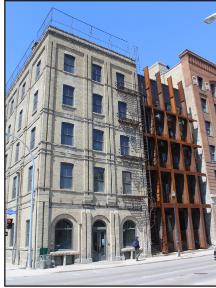
Warehouse, 104 Princess Street, most of the exterior work completed, 2020. (City of Winnipeg)
