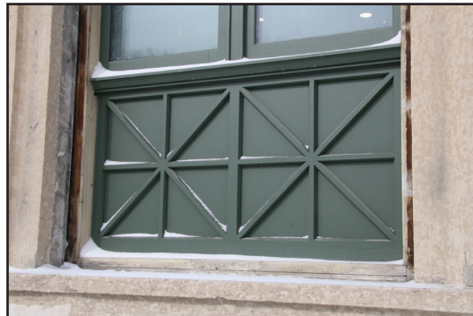
New window unit and ornamental detailing, east façade, Ukrainian Labour Temple, 591 Pritchard Avenue. (City of Winnipeg)
