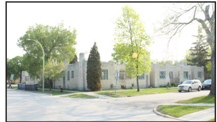
The Ferndale Avenue and Walmar Street façades of the Buena Vista Apartments, 40 St. Mary's Road.
