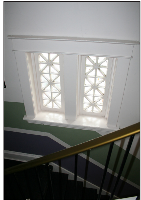
Ornamental windows in staircase of Assiniboia Municipal Hall, 3180 Portage Avenue.
