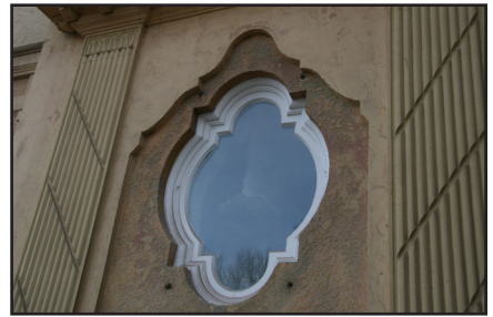
New sashes and niche, 2020. (City of Winnipeg)
