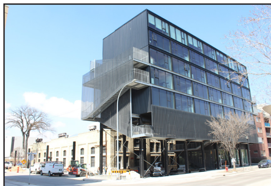
Completed and occupied residential tower to the east of the Pumping Station. (M. Peterson)
