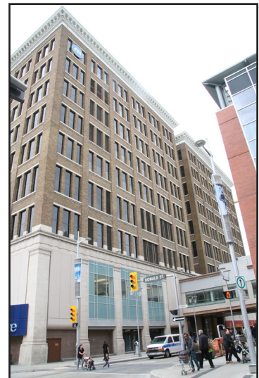
T. Eaton Company's Mail Order and Catalogue Building, 333 St. Mary Avenue, north façade.
