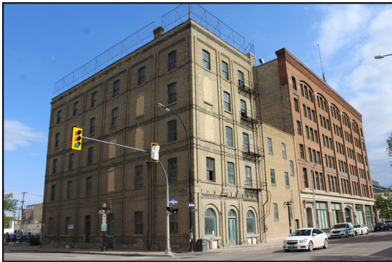
Warehouse, 104 Princess Street, redevelopment underway, 2019. (City of Winnipeg)
