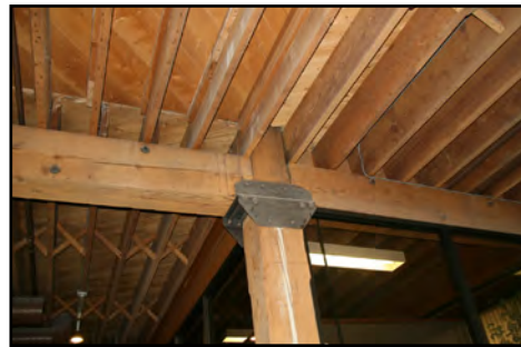
Example of the mill construction, ground floor, 93 Lombard Avenue
