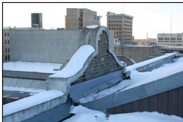
Parapet, Steele Briggs Building
