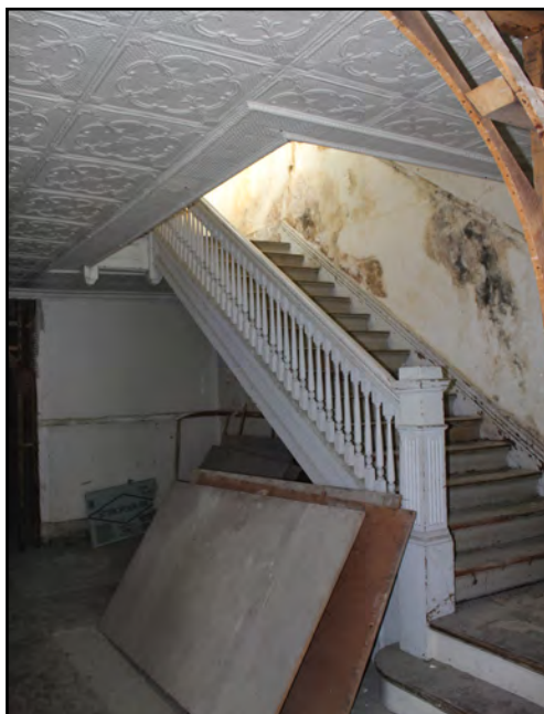
Second floor staircase, Monte Cassino Court
