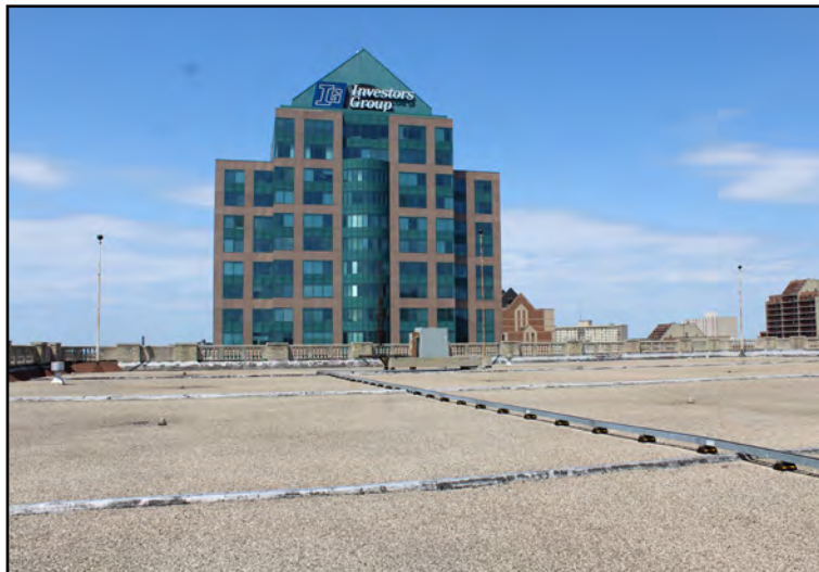
Roof of the Hudson's Bay Company Store, 450 Portage Avenue
