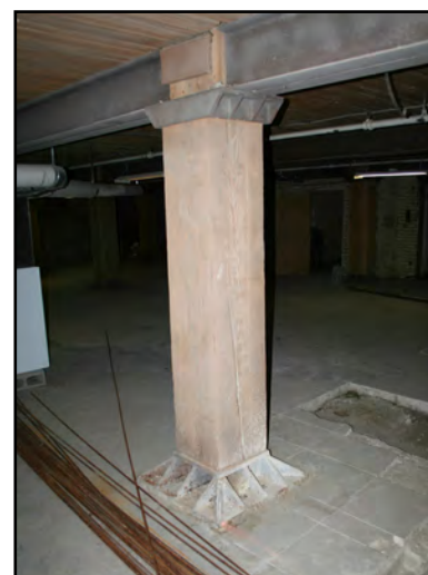
Heavy timber post with steel supports, basement, Steele Briggs Building
