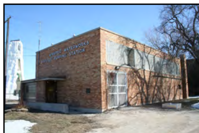
Booster Station, 866 Avenue Taché
