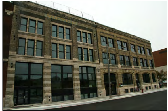
130 and 132 James Avenue façades
