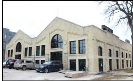
James Avenue Pumping Station, repaired masonry and new windows
