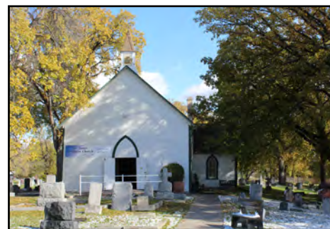
St. James Anglican Church and Cemetery, 525 Tylehurst Street
