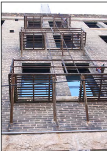
Metal fire escape on west façade, Ryan Brothers Building
