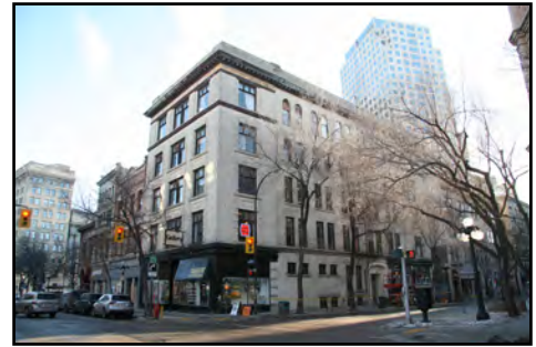
Silvester-Willson Building, 75 Albert Street
