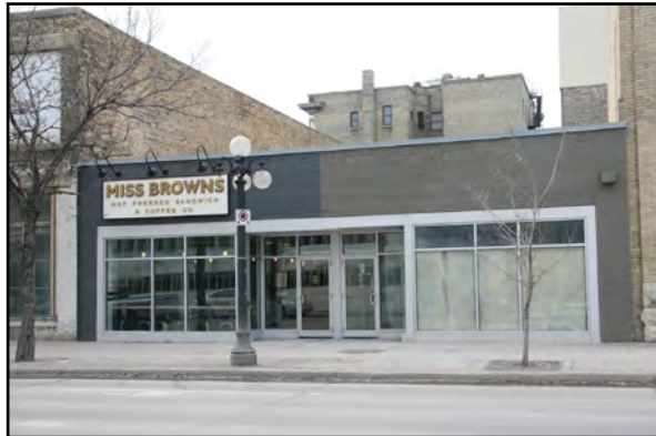
Soudack Building, 288 William Avenue
