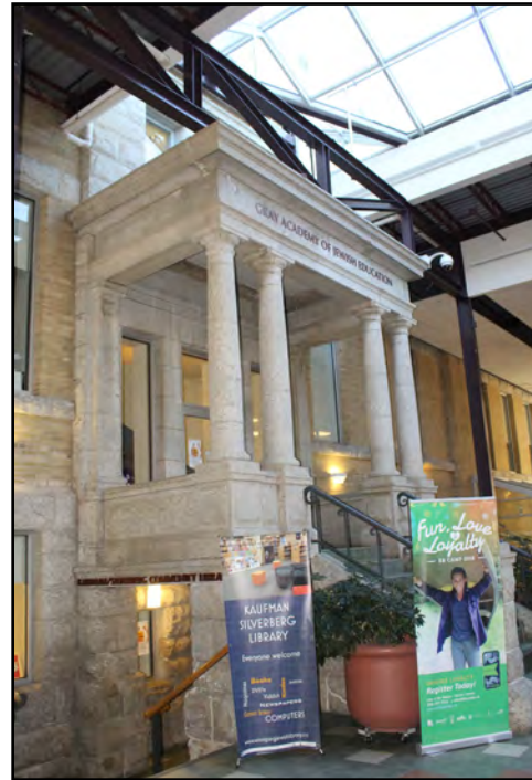
Additions on the north side of the Manitoba Agricultural College Administration Building have created an interior façade of the original north elevation
