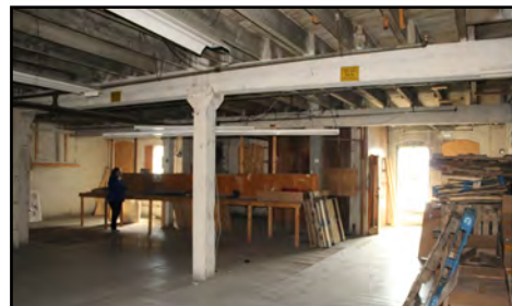
Interior warehouse space, Trees-Spriggs Building
