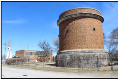
Surge Tank in the foreground with the Booster Station behind, 866 Avenue Taché
