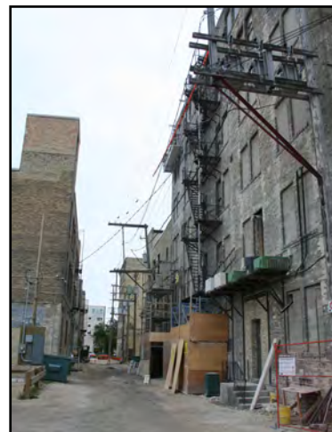
Back lane (formerly Elgin Avenue), between Market and James Avenue, Stanley Brock Building on the right
