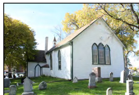
Rear (east) and south façades, St. James Anglican Church
