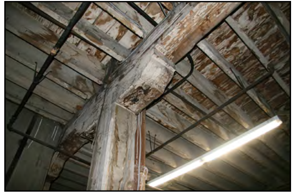
Example of the mill construction, G.F. and J. Galt Block
