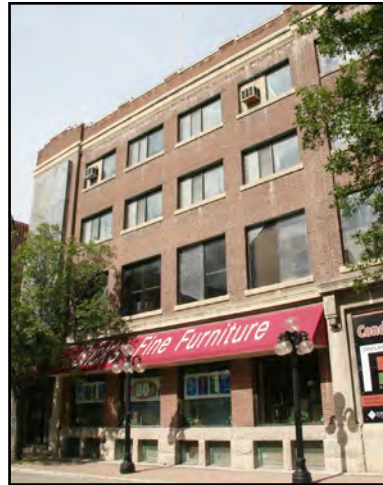
Stanley Brock Building, 145 Market Avenue
