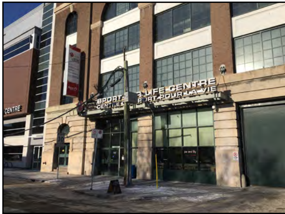
New signage on the Smart Bag Company Building
