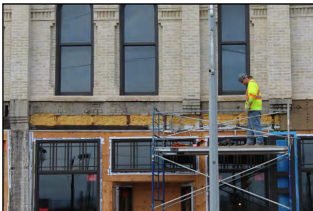
Work on the ground floor retail space
