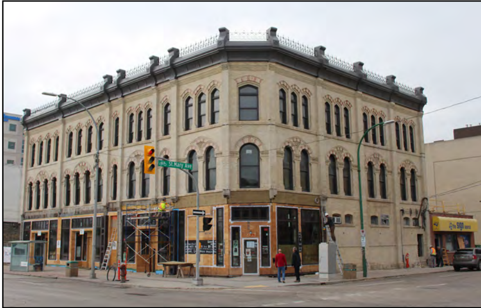
Commercial and Fortune Blocks during restoration
