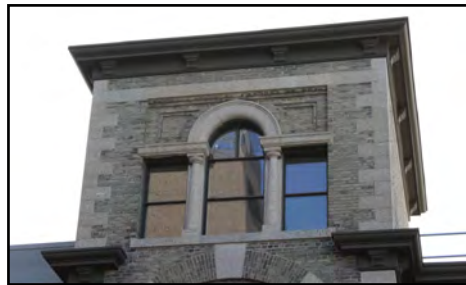
Tower detail, Manitoba Medical College Building
