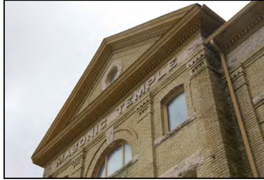
Detail of main façade, Masonic Temple
