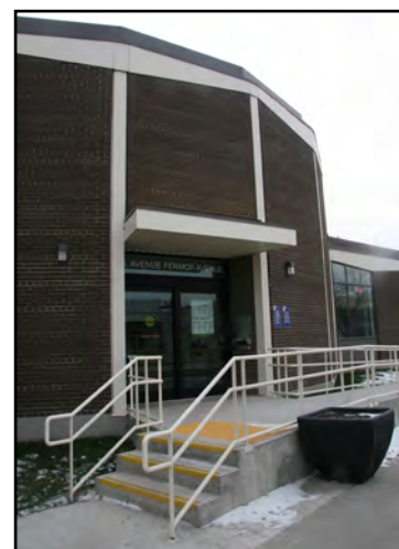
Newly designed main entrance, St. Vital Library
