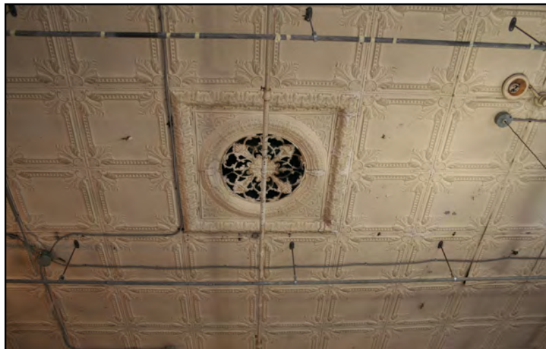
Ornamental tin ceiling, 5th floor, Silvester-Willson Building
