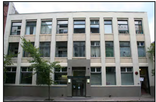
Dominion Electric (Hemisphere) Building, 87 Princess Street
