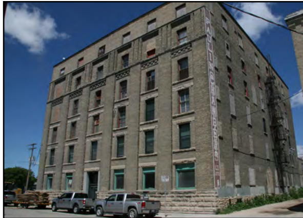
Paulin-Chambers Building, 311 Ross Avenue
