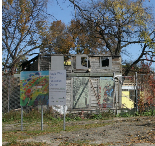
Restoration work underway at Barber House.
