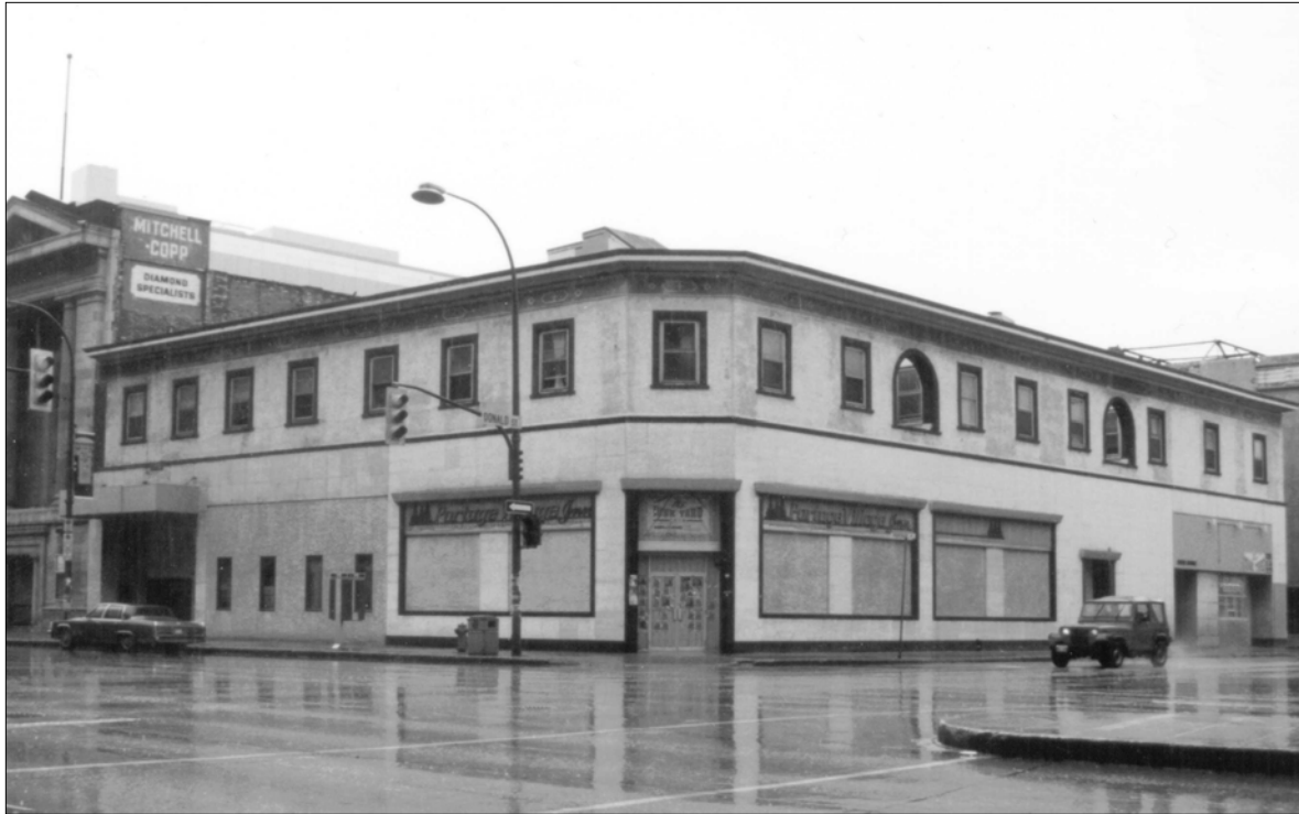
The vacated Portage Village Inn, prior to its rehabilitation, 1999. City of Winnipeg
