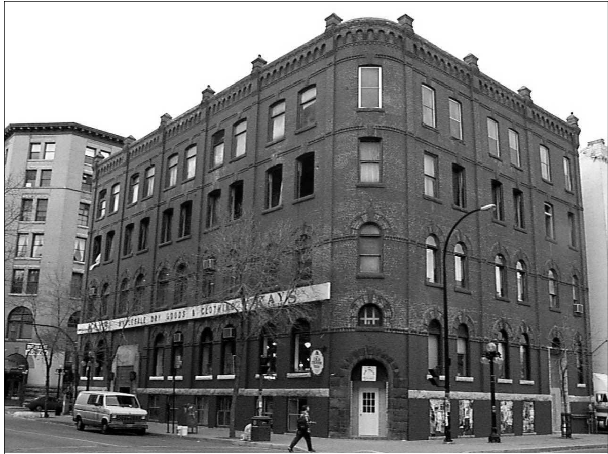
Kay Building, 1998. City of Winnipeg
