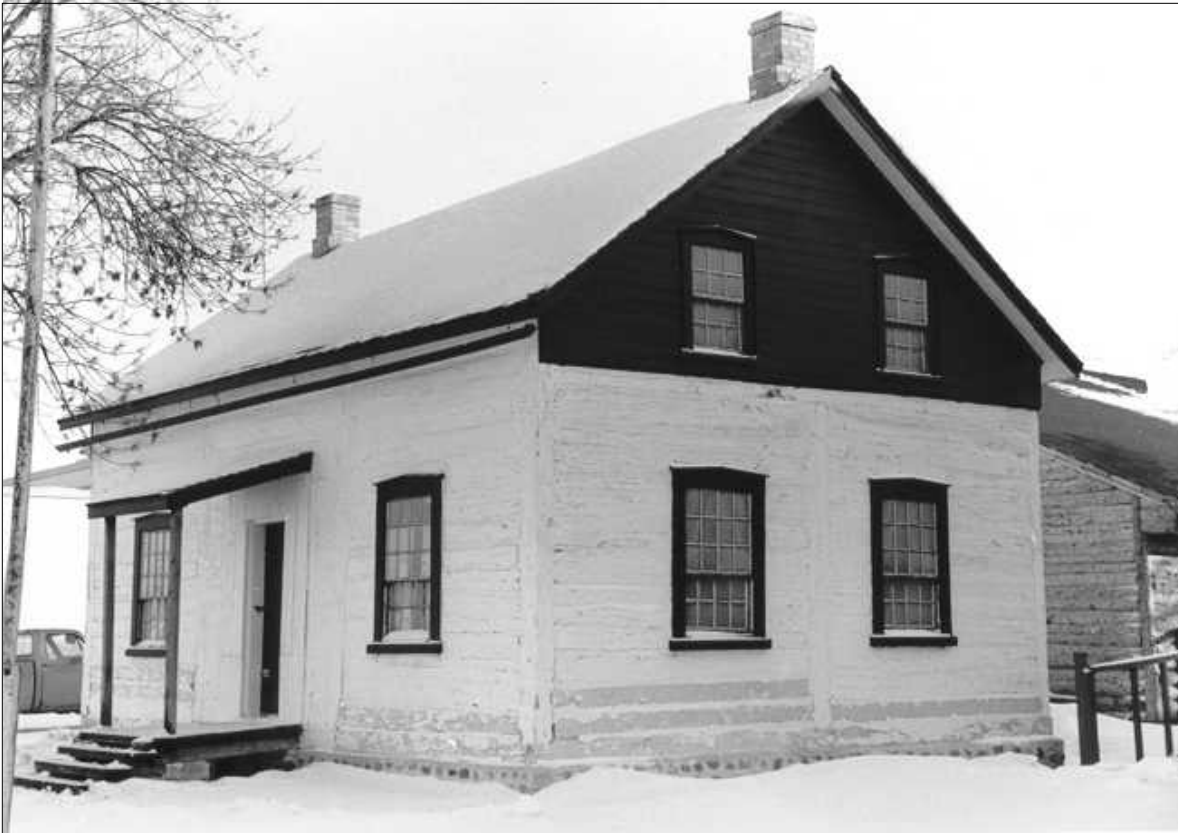
The Brown House in its new location as a museum, Portage Avenue, 1996. City of Winnipeg
