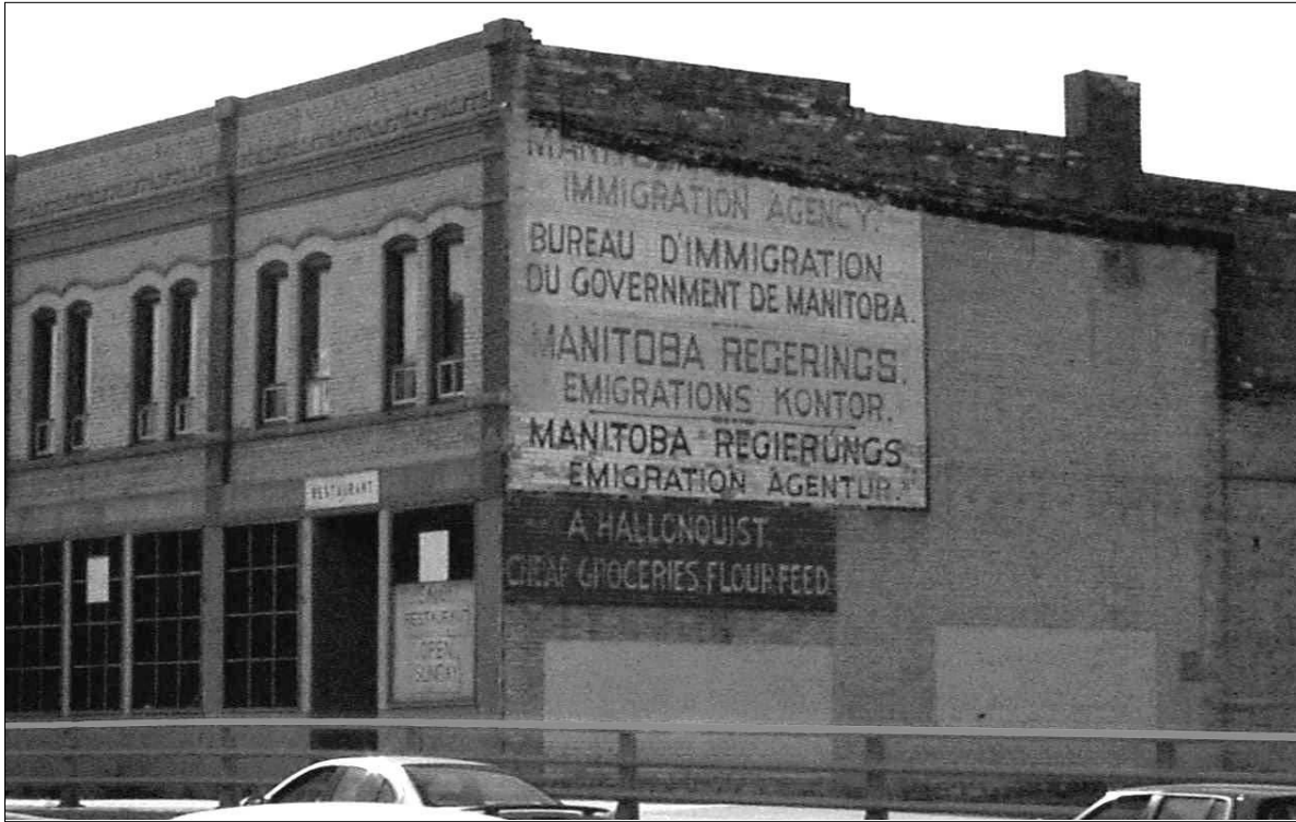
The demolition of the neighbouring building uncovered this painted advertisement on the north wall of the Savoy Hotel. It lists two of the early occupants of the Sproule Block, 1998. City of Winnipeg
