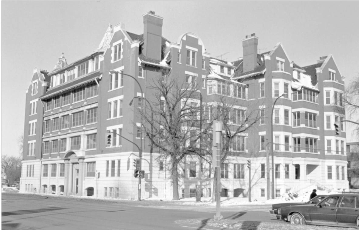
The magnificent south and west façades of the Roslyn Court Apartments, 1998. City of Winnipeg
