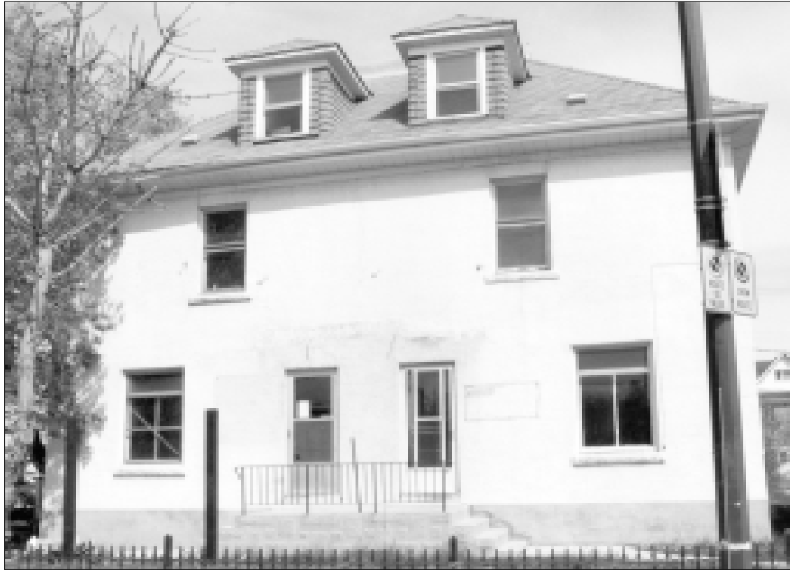
The severely altered front façade of the Royal House, 1998. City of Winnipeg
