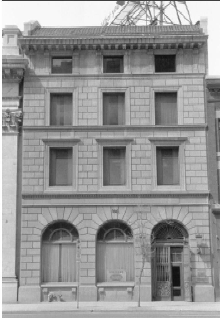
The Leon A. Brown Building, 1999. City of Winnipeg
