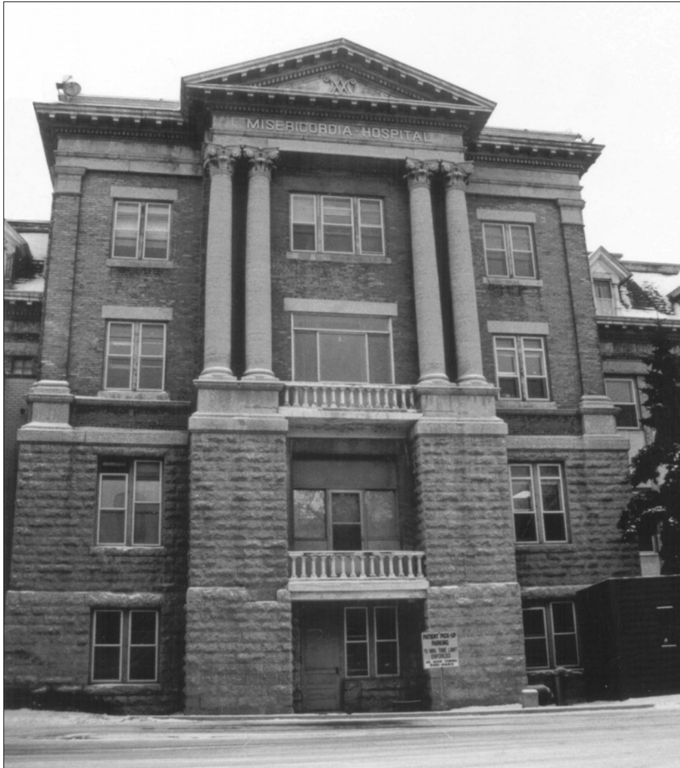
The 1906 façade of the Misericordia Maternity Hospital in 1997. City of Winnipeg
