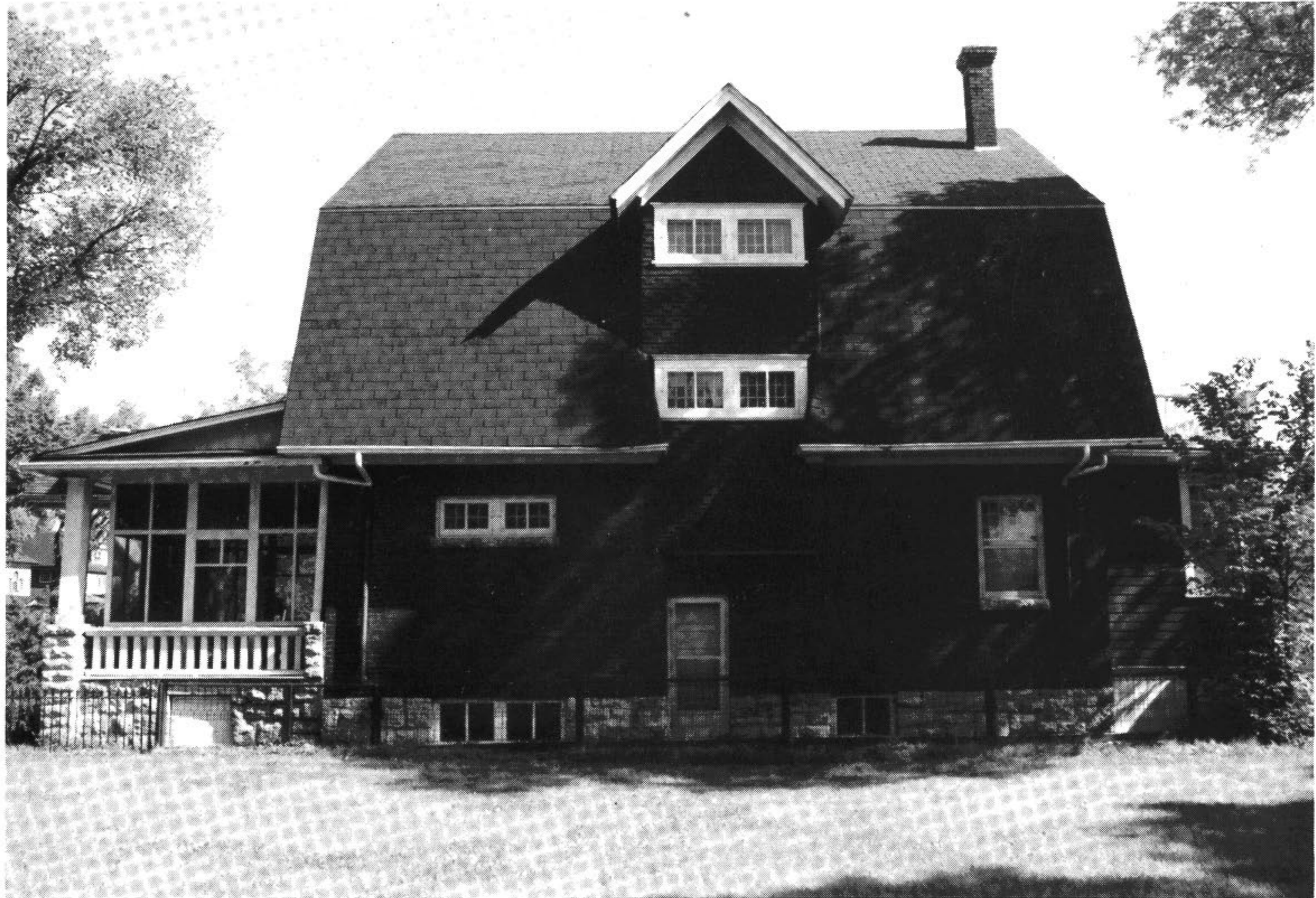
A side view showing the gambrel roof. City of Winnipeg
