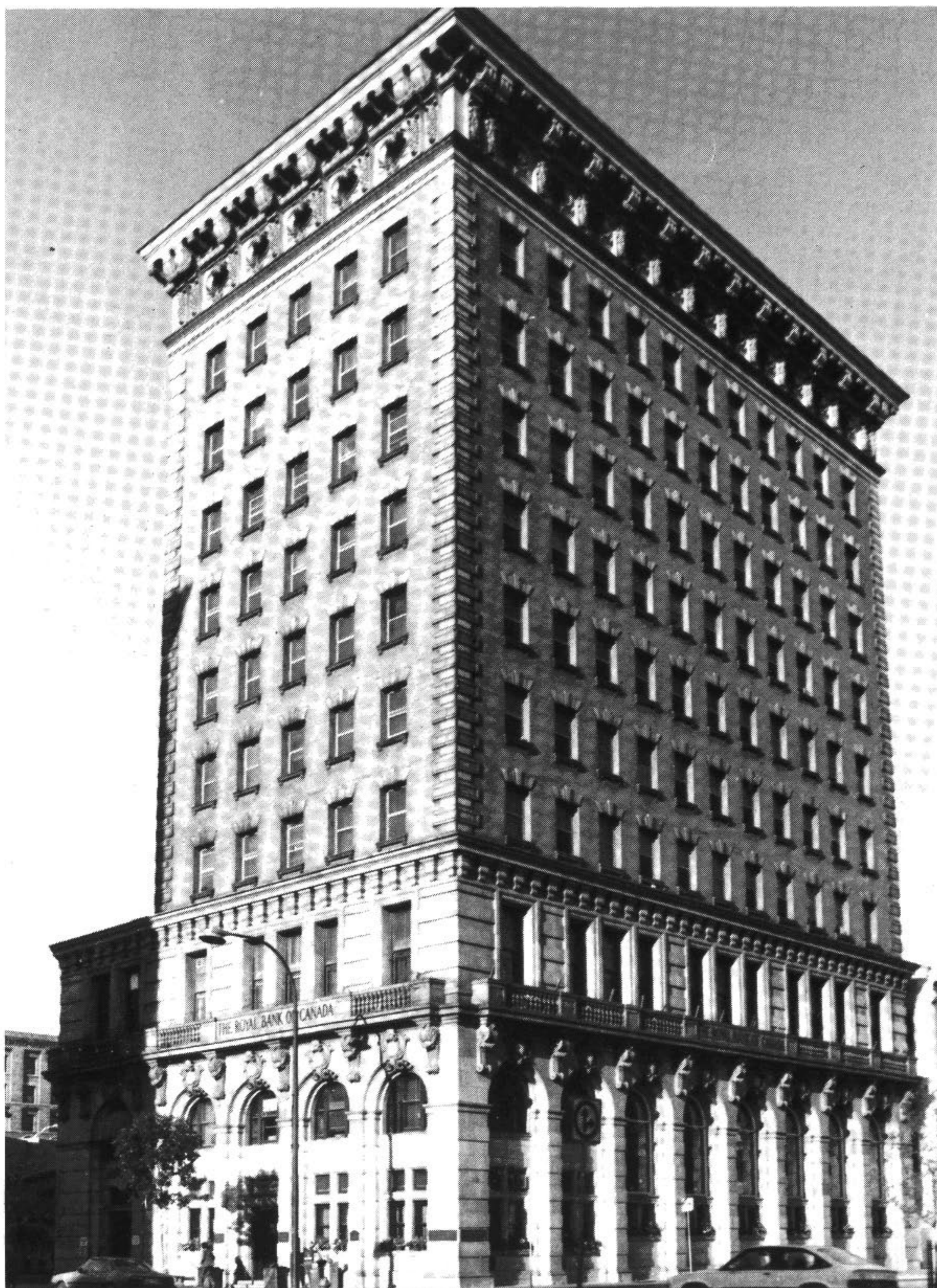
Darling and Pearson's Union Bank Building in 1992. City of Winnipeg
