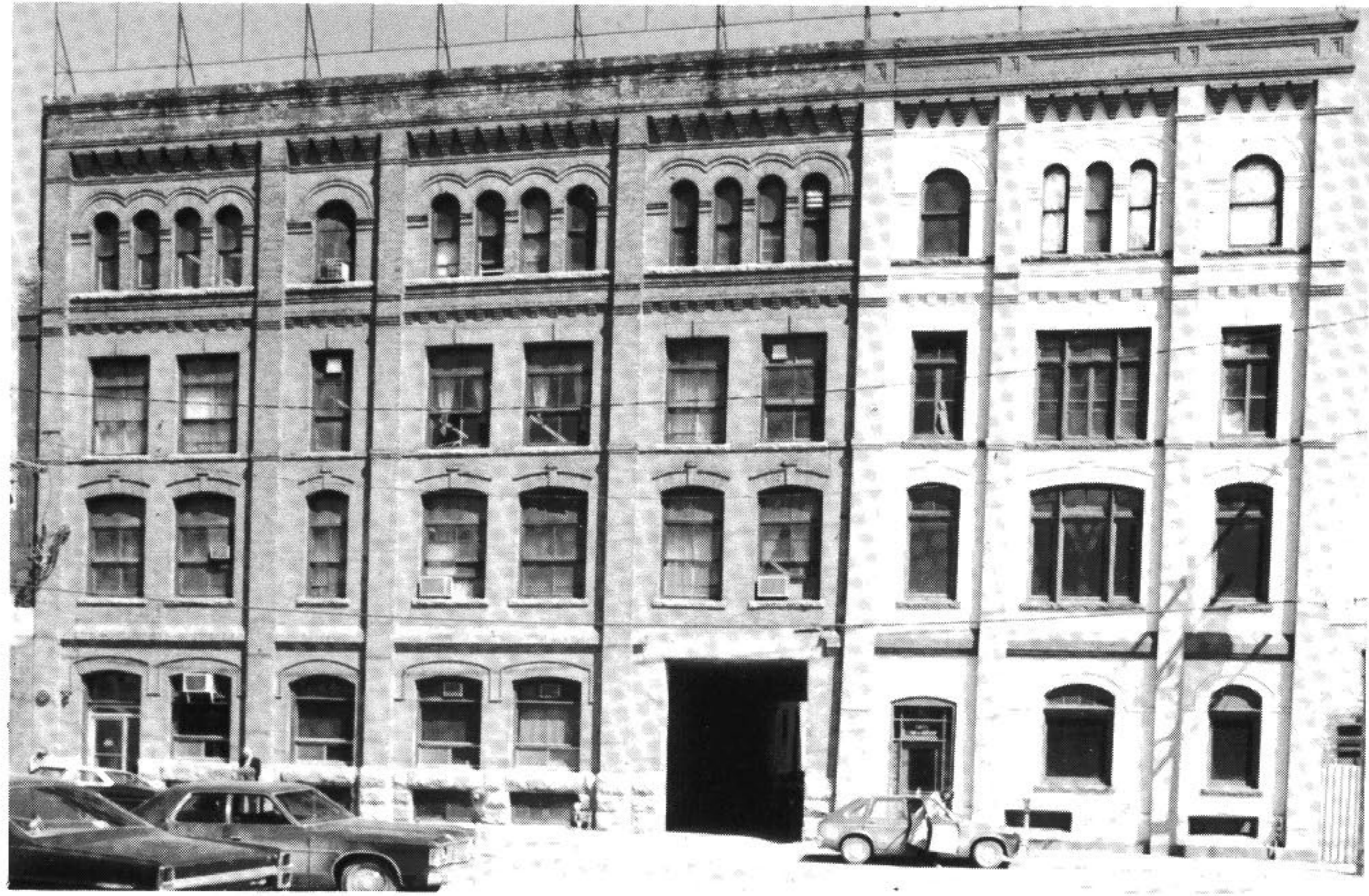
137 and 141 Bannatyne Avenue prior to rehabilitation, c. 1975. City of Winnipeg
