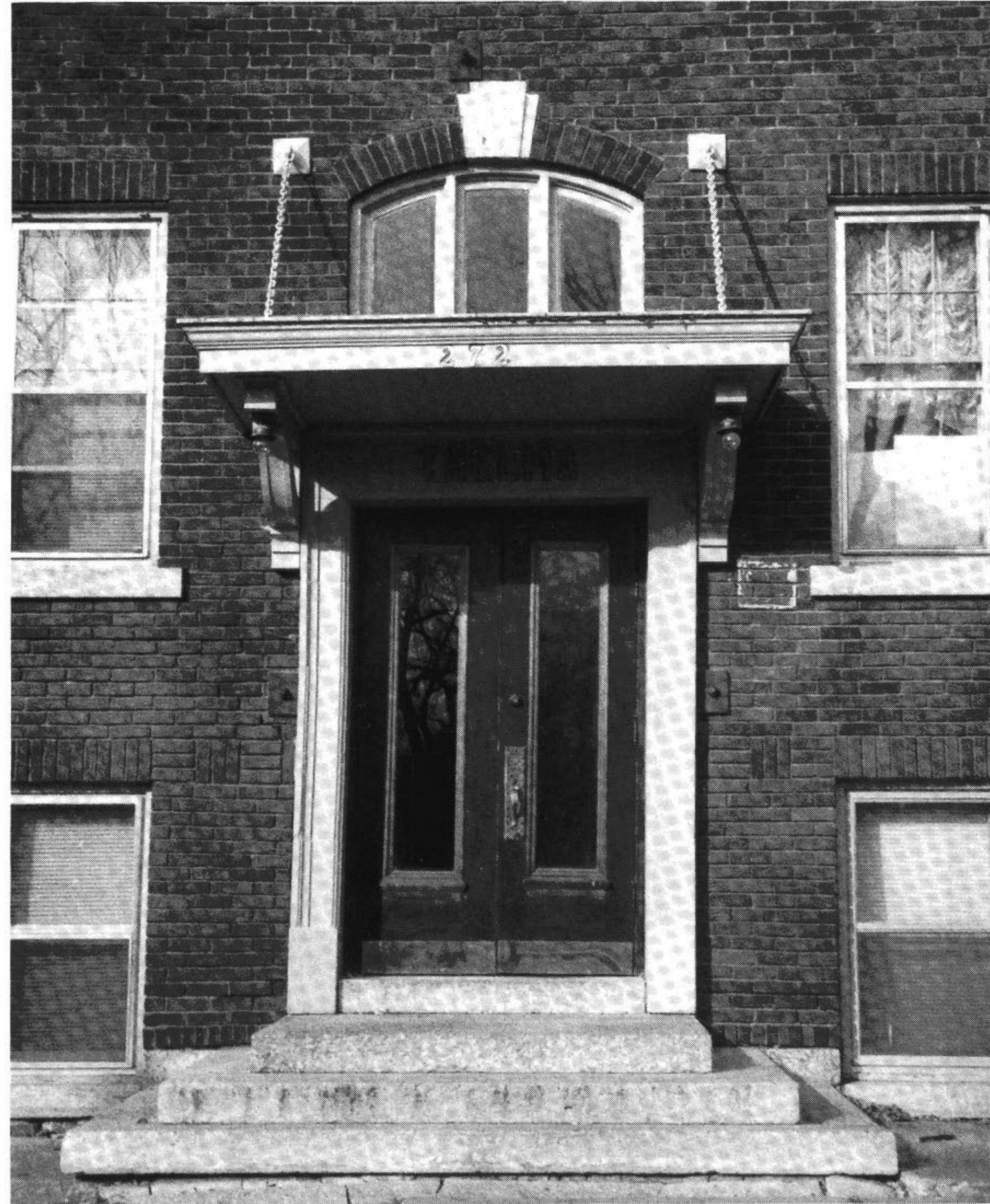
The detail of the front entrance. City of Winnipeg
