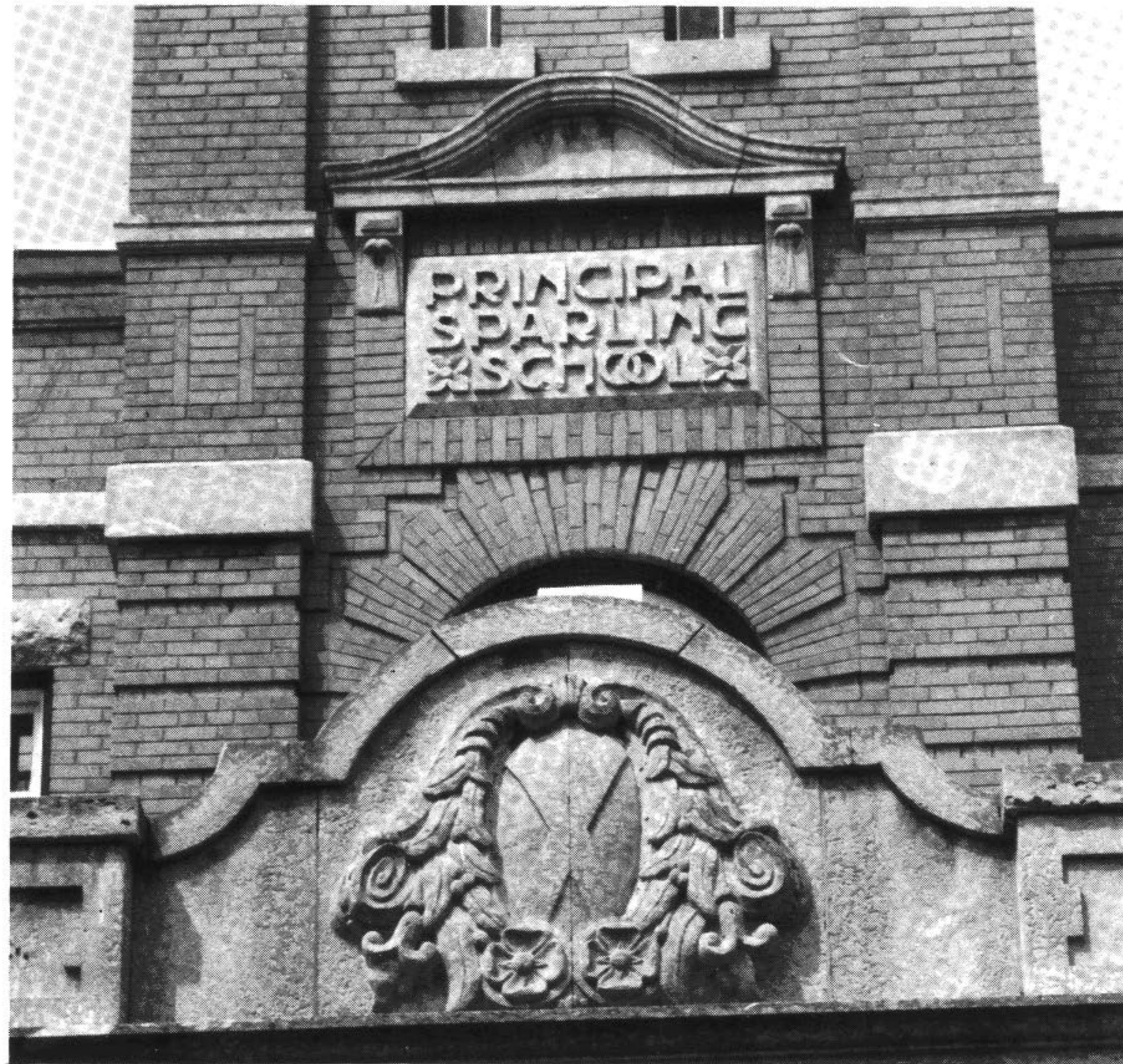
Detail above the front entrance. City of Winnipeg
