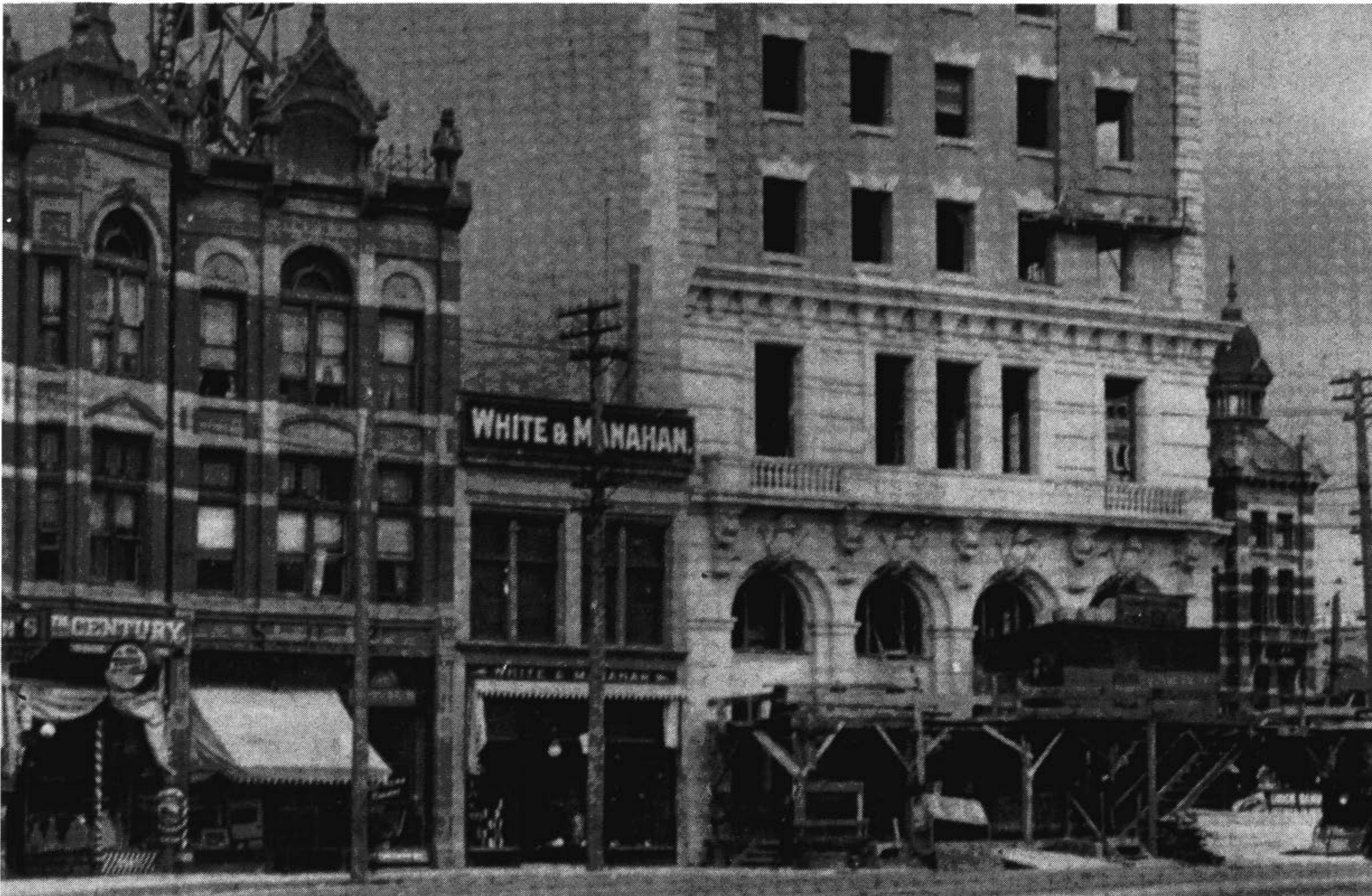
The White and Manahan Building (centre) during the construction of the Union Bank Building, c. 1905. Provincial Archives of Manitoba
