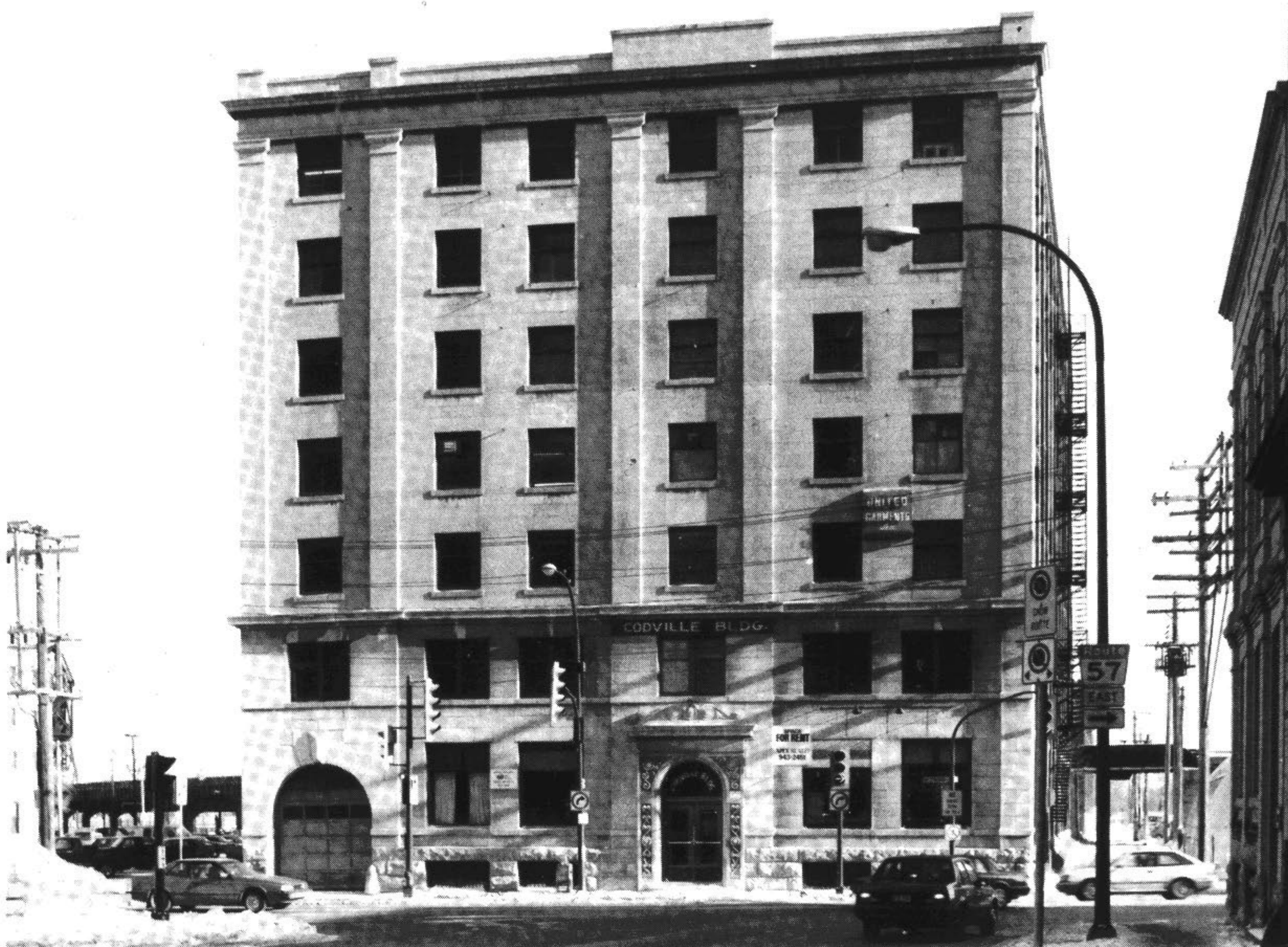
The Codville Company's warehouse building, 1993. City of Winnipeg
