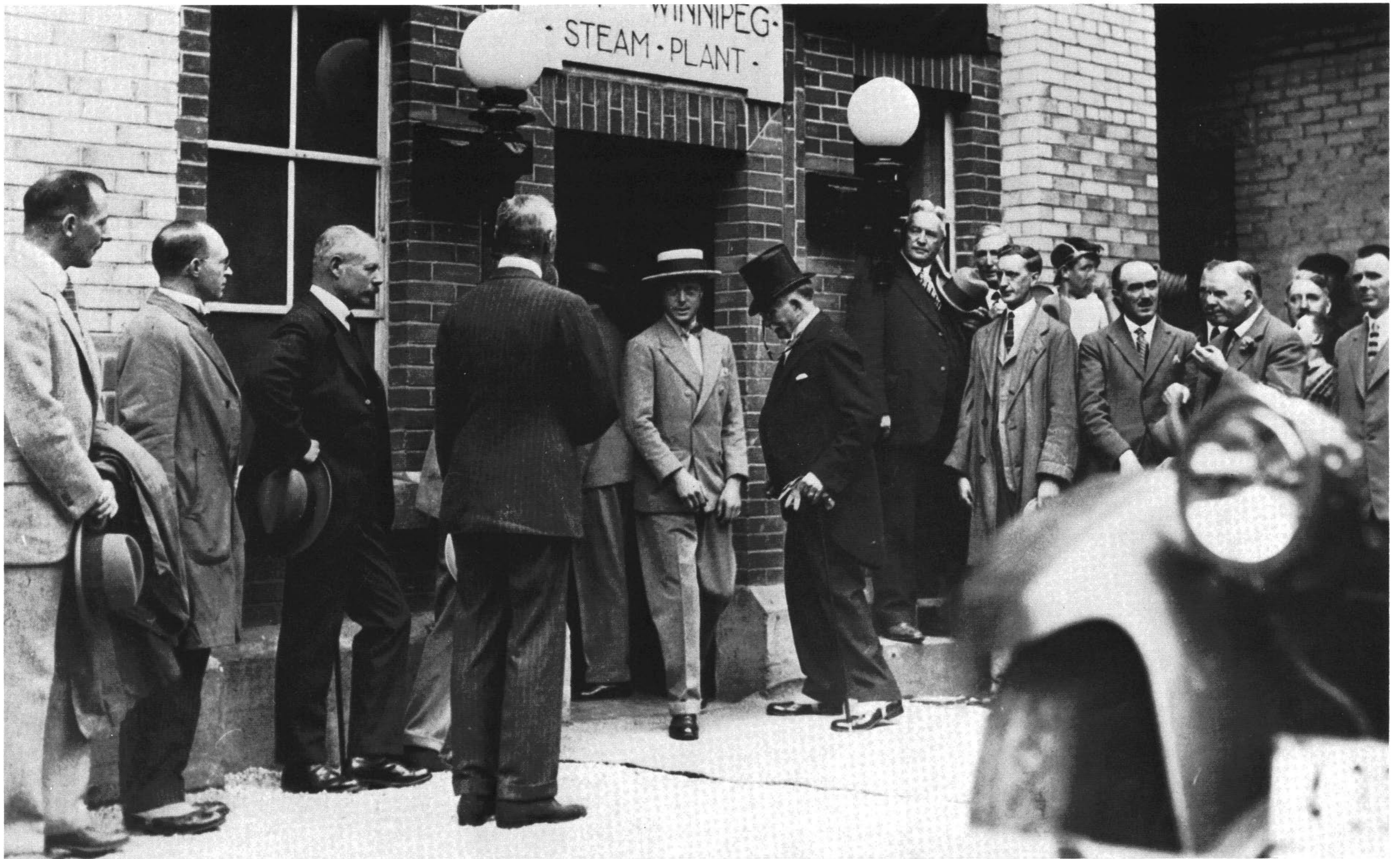
The visit of the Prince of Wales to the Winnipeg Steam Plant, 1927. Provincial Archives of Manitoba
