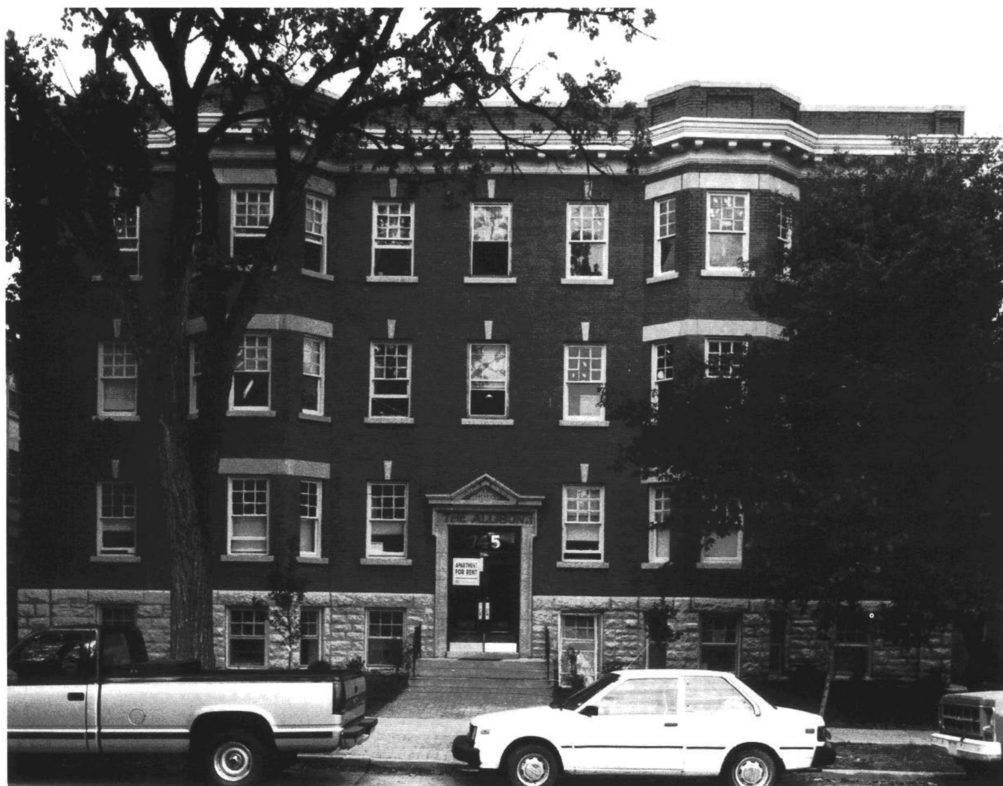
745 Wolseley Avenue in 1990. City of Winnipeg
