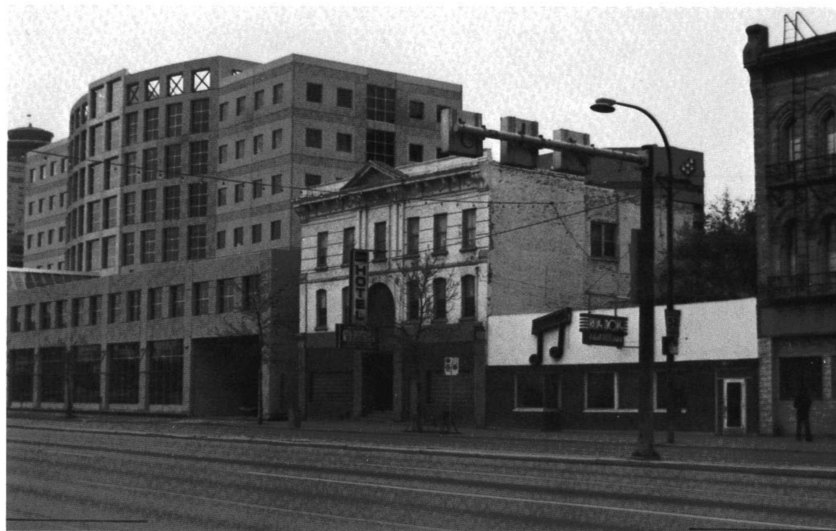
A view of the Winnipeg Hotel in 1990. City of Winnipeg
