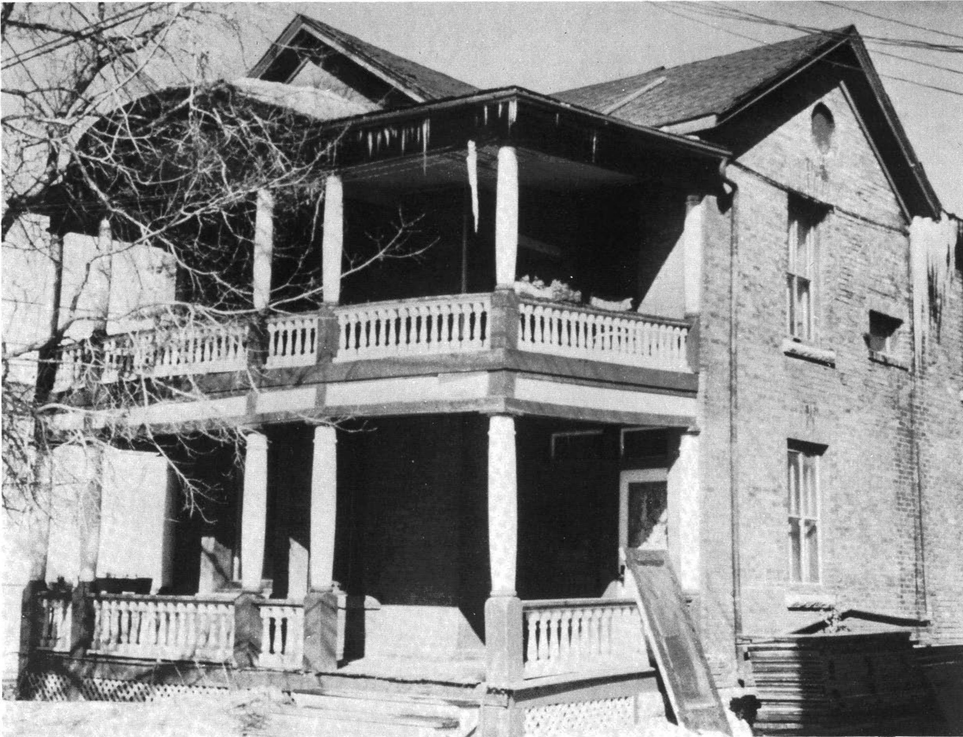
115 Pioneer Avenue with its large porch, c.1974. R.Rostecki Collection
