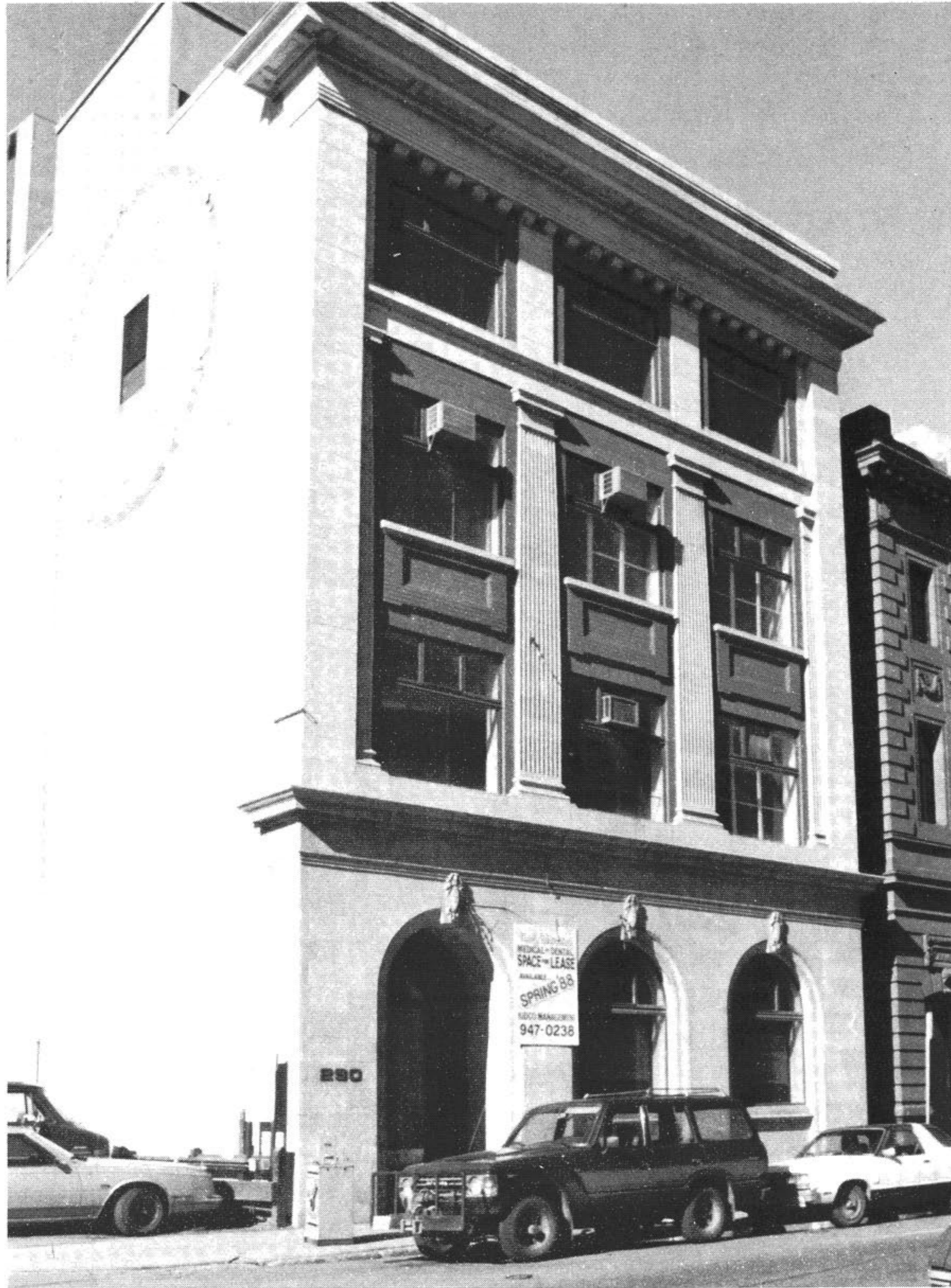
The Garry Block in 1987. City of Winnipeg
