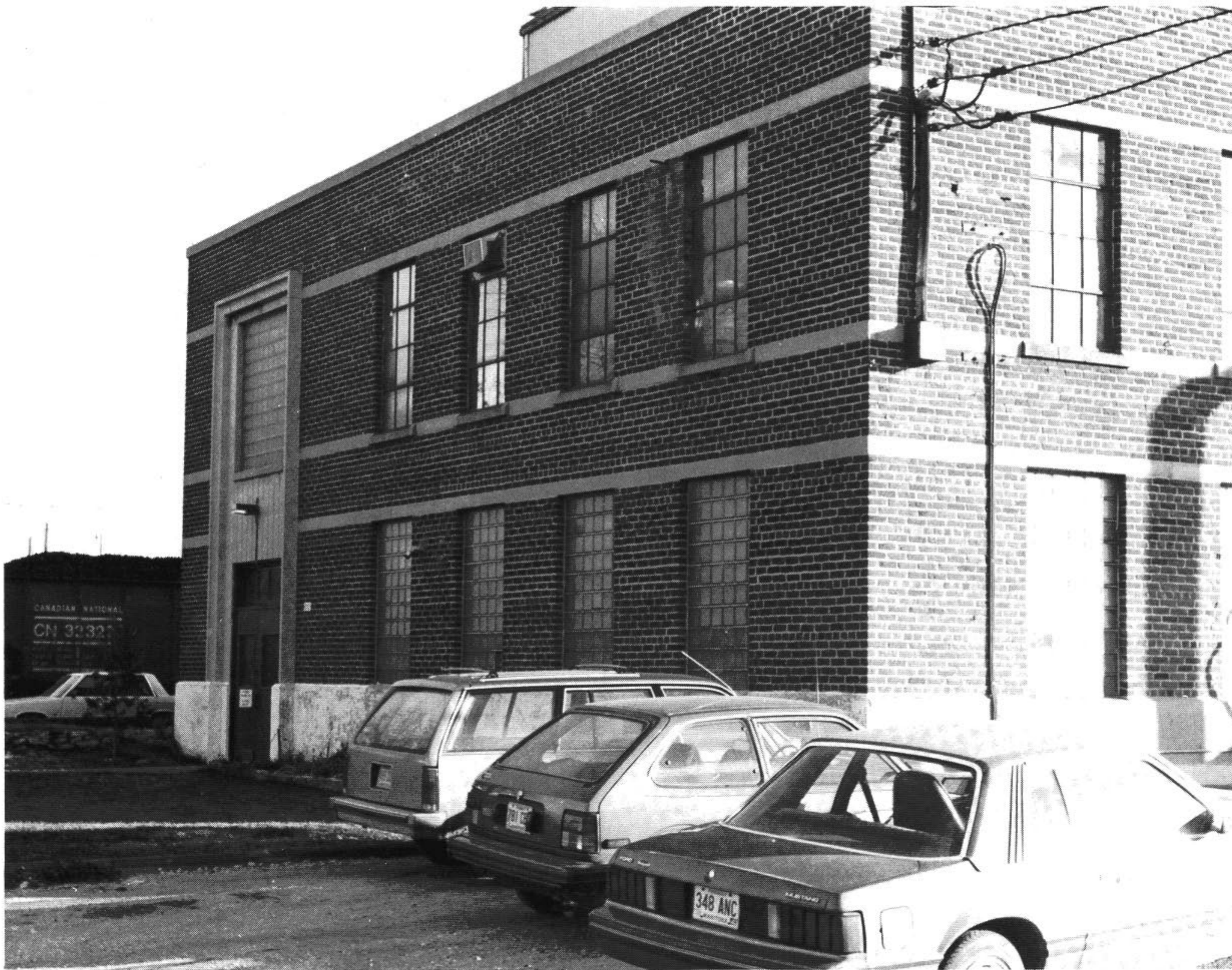
The C.N.R. Power Plant in 1987. City of Winnipeg
