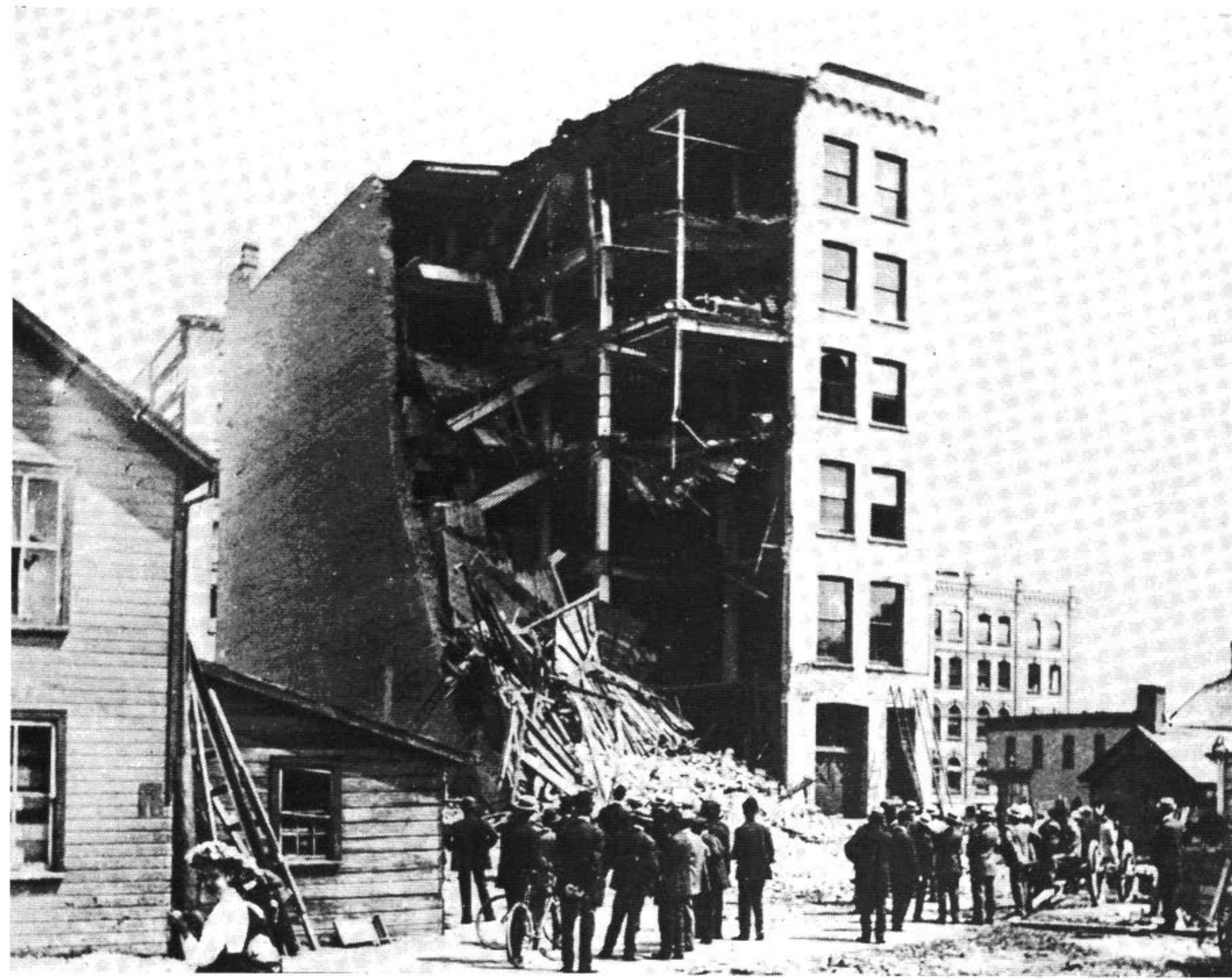
The collapsed rear of the Wilson Building, 1909. Provincial Archives of Manitoba
