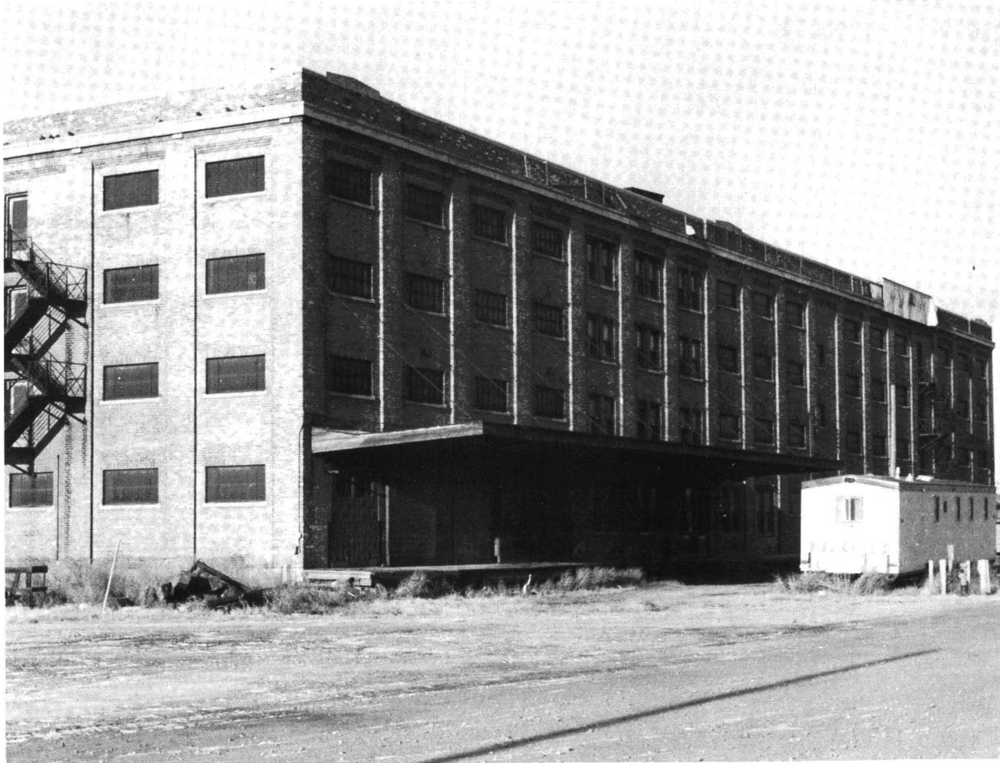
The Johnston Terminal Building, one of the largest warehouses in Winnipeg. City of Winnipeg
