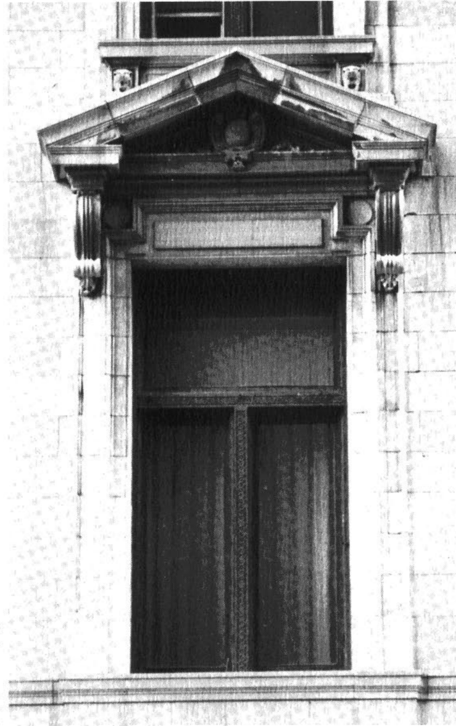
Detail of second-floor perimeter window with pedimental head supported on brackets.
