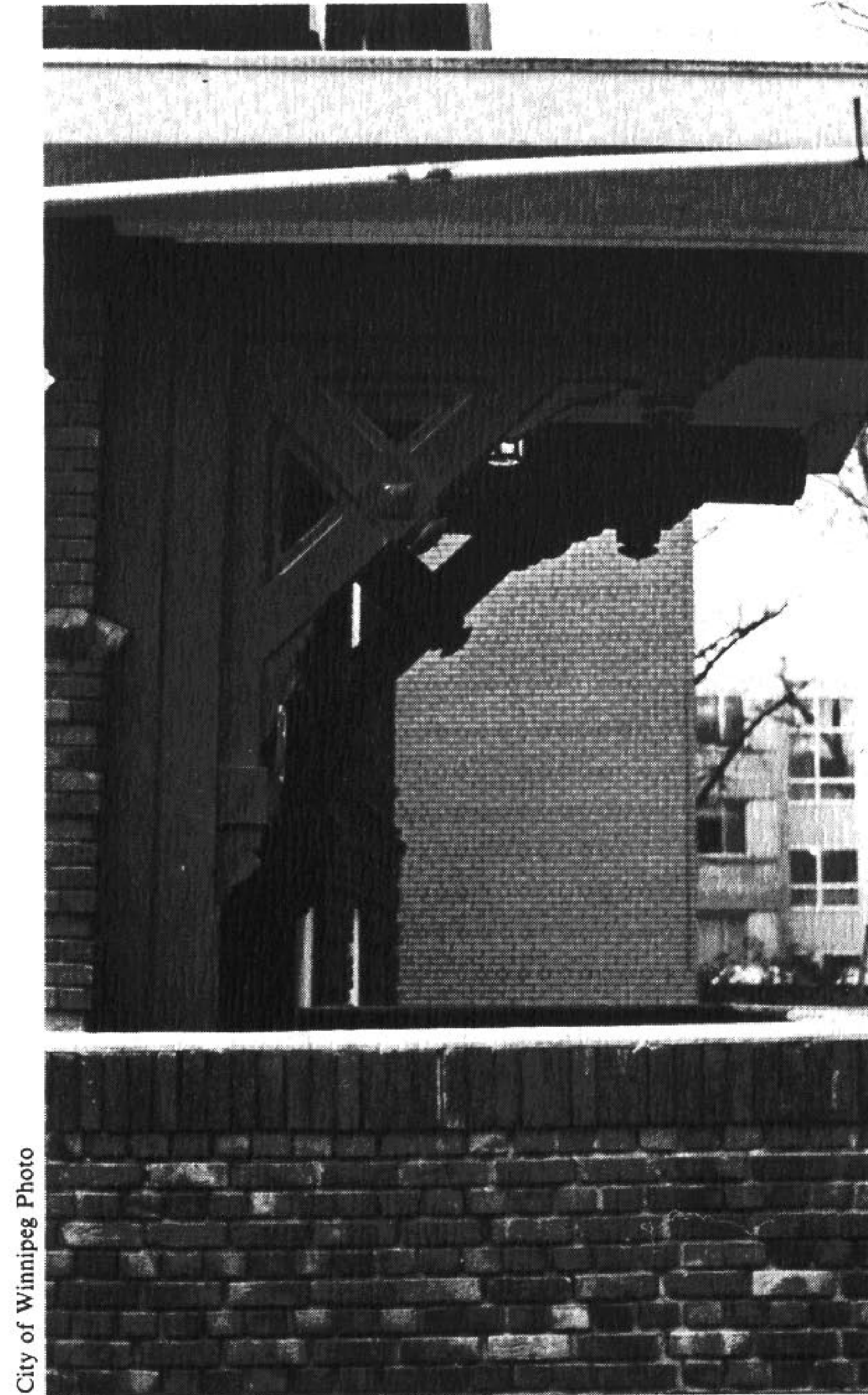
Detail of elaborate bracket supporting the roof of the entrance-way.
