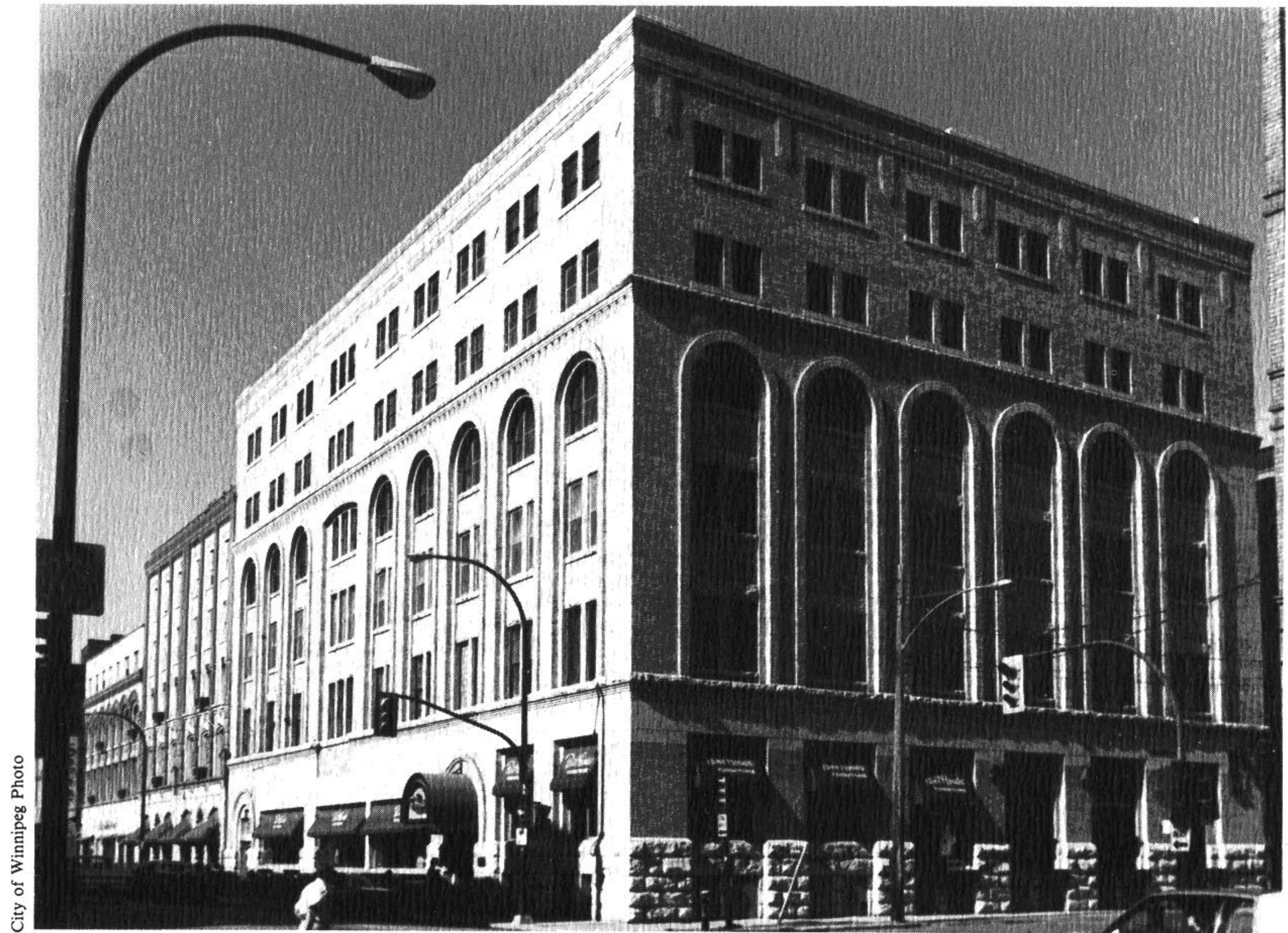
The Campbell Bros. and Wilson Building with its two storey addition.
