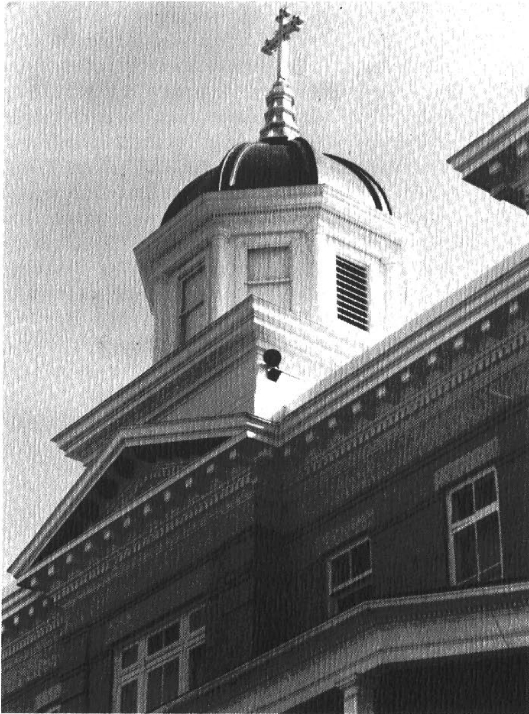
Detail of the elaborate cornice and central dome on the 1911 addition.
